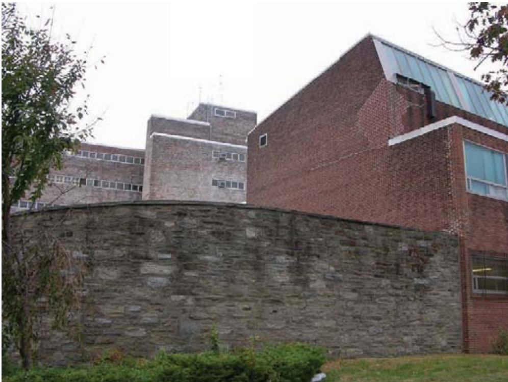
fig. 7 SW view from Pennsylvania Avenue, slanted roof and skylights, photo by Anny Su, November 2005
