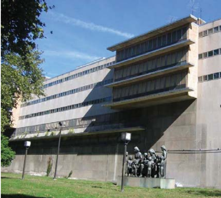
fig. 10 Boarded windows on Parkway façade, photo by Anny Su, November 2005
