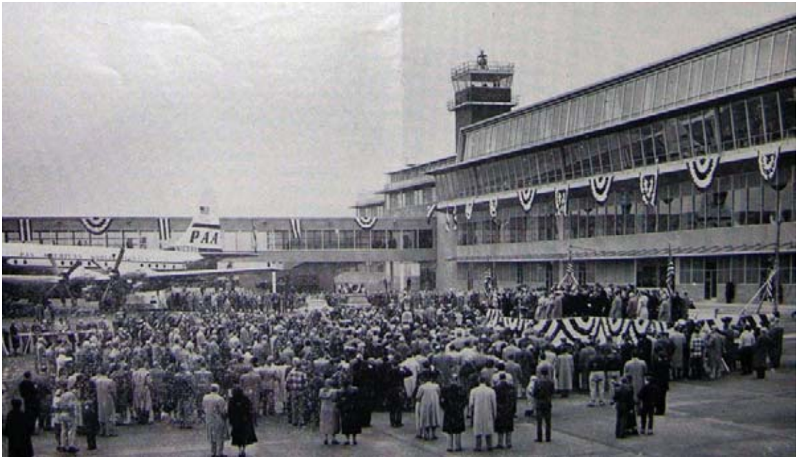
fig. 38 Detail of Philadelphia International Airport on Dedication Day, Commercial America (January 1954) 9.
