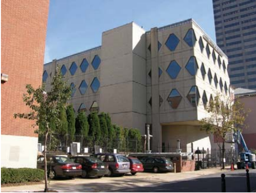
fig. 39 East view of American Society for Testing and Materials (currently Moore College of Art) at 19th and Parkway, photo by Anny Su, November 2005
