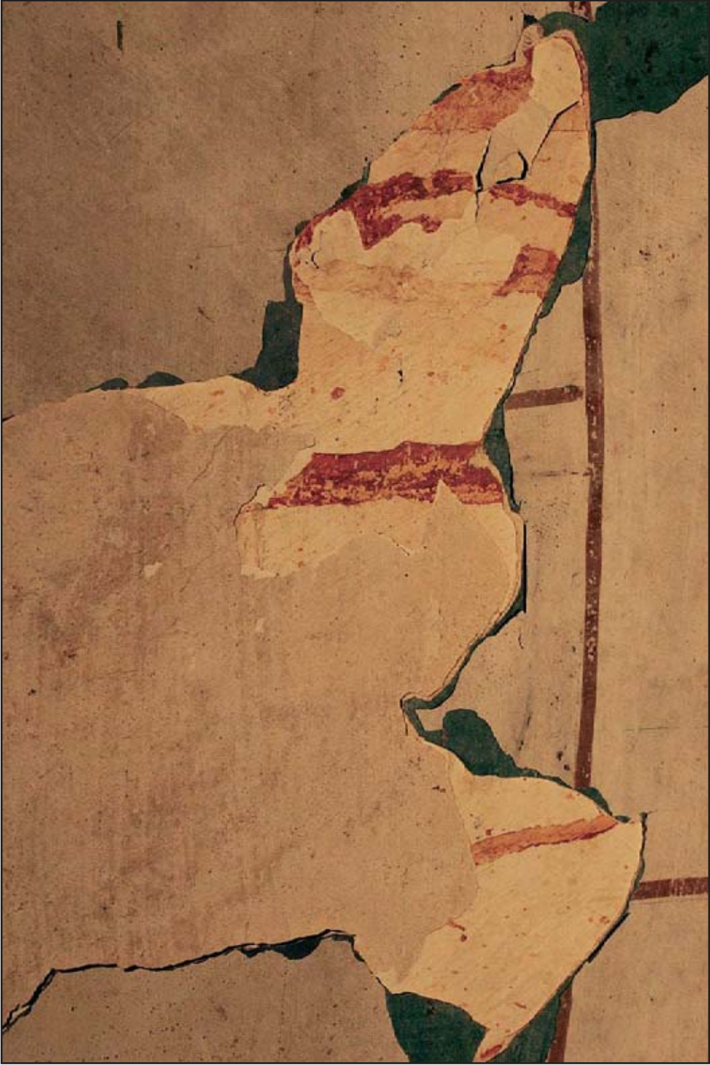
Figure 31: Detail (A6-3). Red marbalizing, Campaign B under later limewashes. (Source: C. Silva, 2006)
