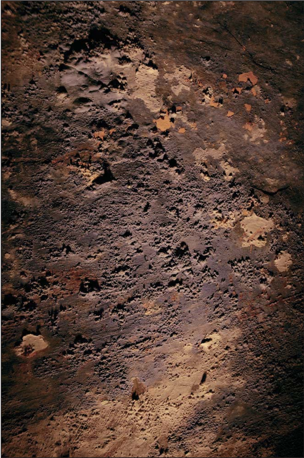
Figure 36: Detail (A6-8) Image of surface conditions: blistering, flaking, and salts. (Source: C. Silva, 2006)
