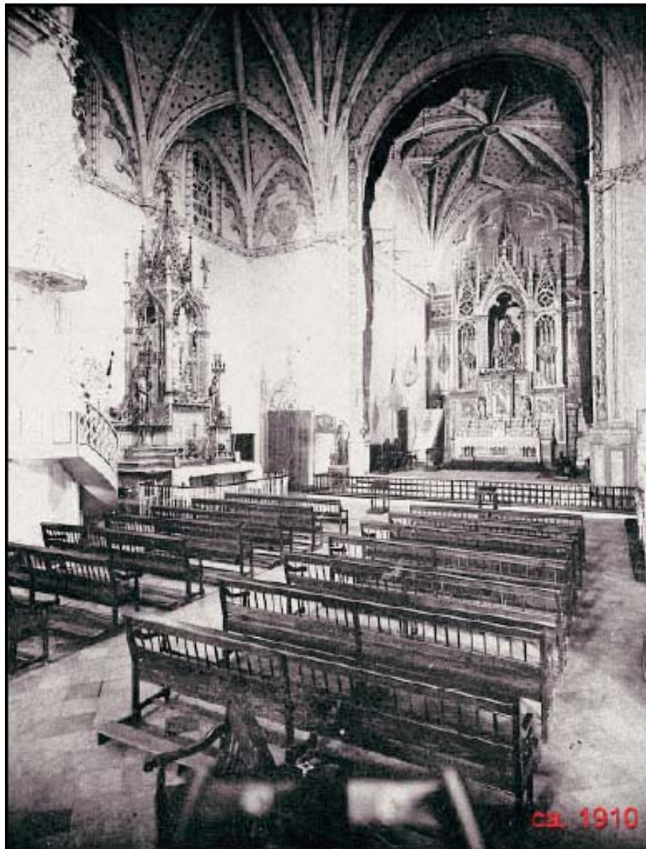
Figure 8: Circa 1910 photograph taken from the transept looking towards the sanctuary. (Source: Antonio Daubón, private collection)
