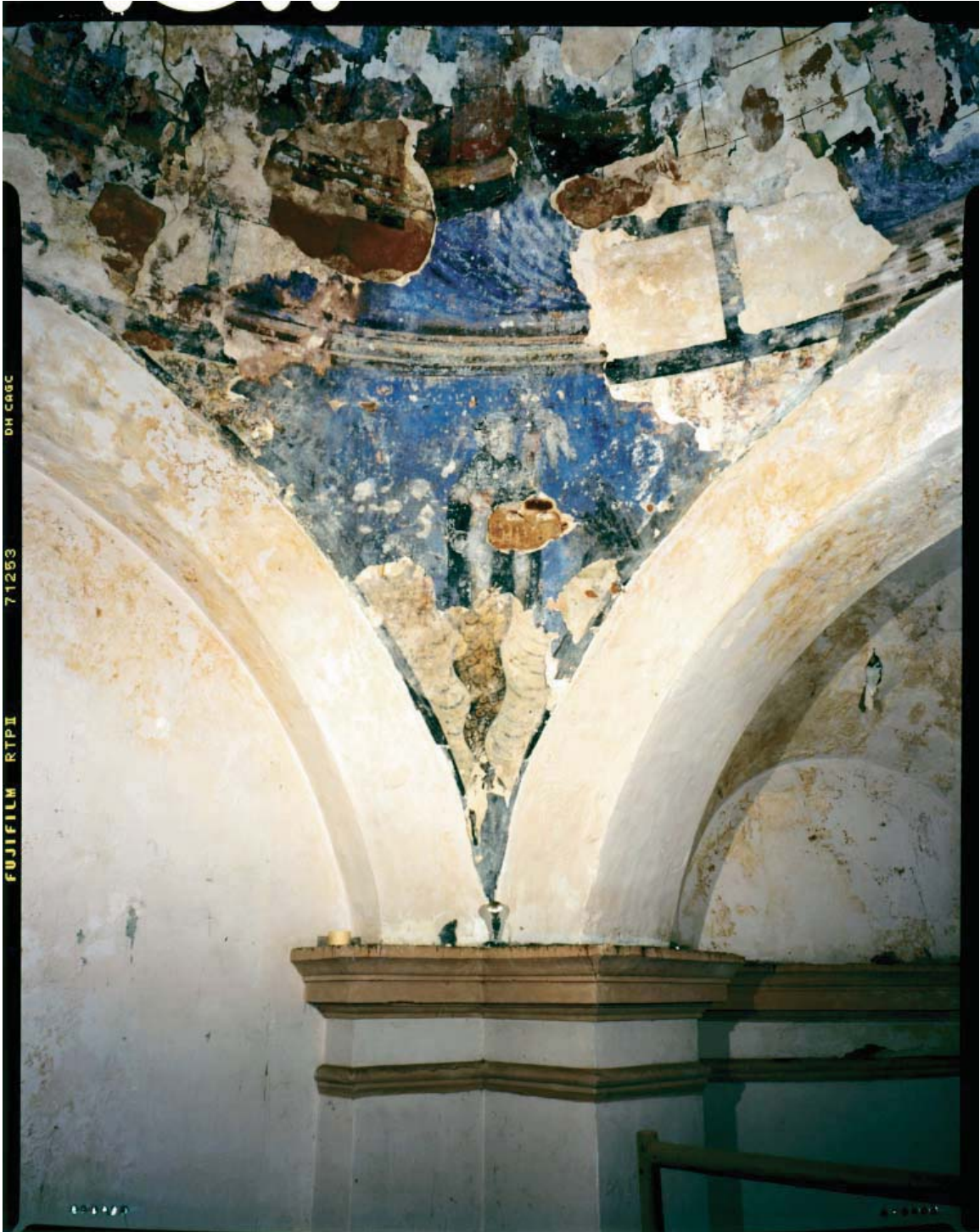
Figure 16: Pendentive 1, southeast corner of Rosario Chapel. (Source: Joseph Elliott, 2004)
