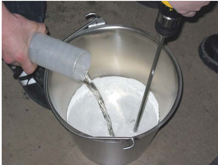
Figure 2.1 – Mixing Grout Formulation A
