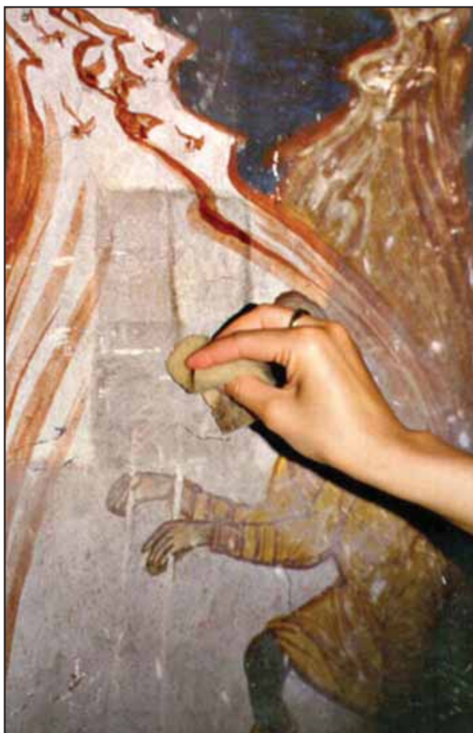
Figure 4.6: Cleaning mural with ion exchange resin through Japanese paper (Source: Metaneira).
