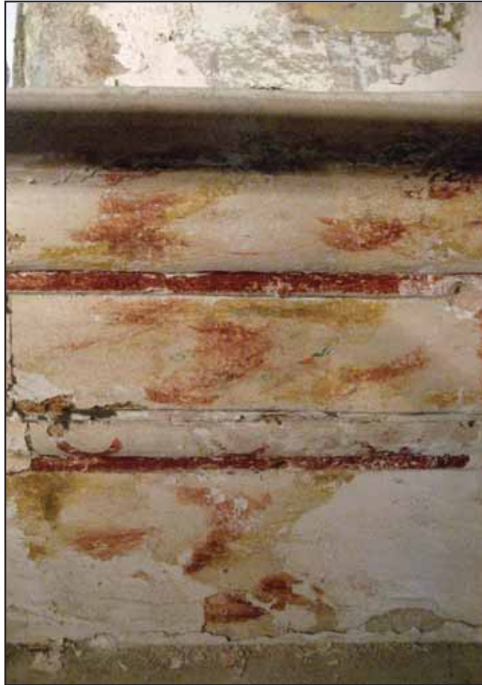
Figure 2.6: Faux marbling on sanctuary cornice (Source: Johnston and Silva, 17).
