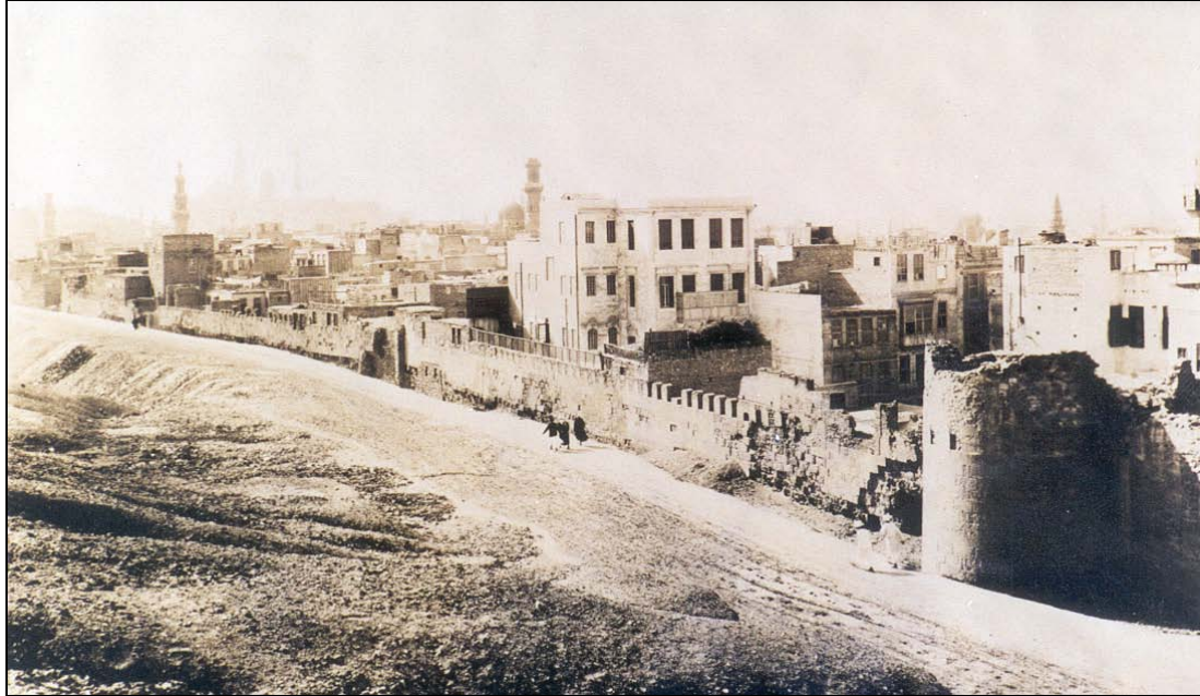
Figure I.4 View of the eastern portion of the Ayyubid city wall of Cairo from the Darassa hills with the former Darb Shoughlan School noticeable in the center of the photo. Note the extensive loss of veneer stone in certain areas of the wall.
