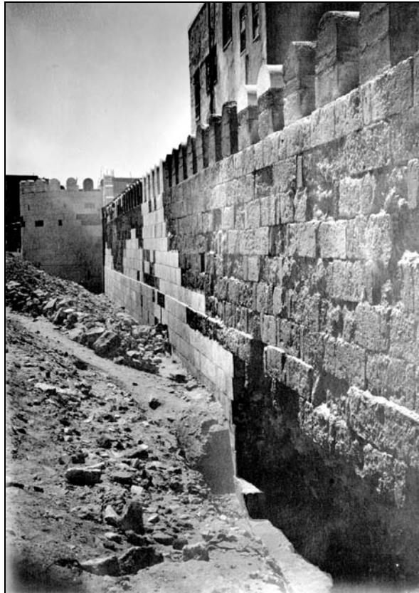
Figure I.7 Tower 4 after Comité reconstruction, 1951.
