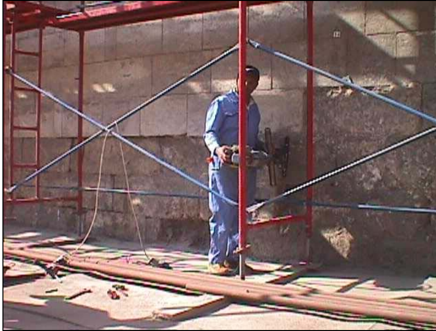
Figure IV.22 Coring of the first core sample. From Rock Engineering Laboratory 2000a.
