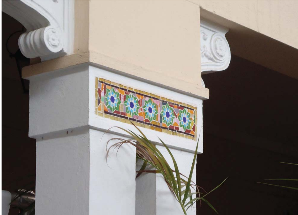
Figure 8: Castillo Serrallès, Ponce, Puerto Rico: interior patio column. (source: by author, 2010)
