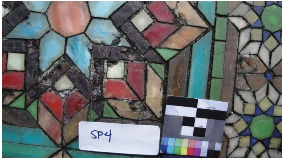
Figure 15: Sample ME_4 Main Entrance door. (source: by author, January,2010.)
