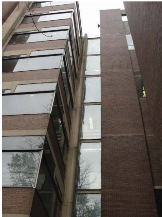
Figure 5.21- Column in situation less exposed to environment action.
