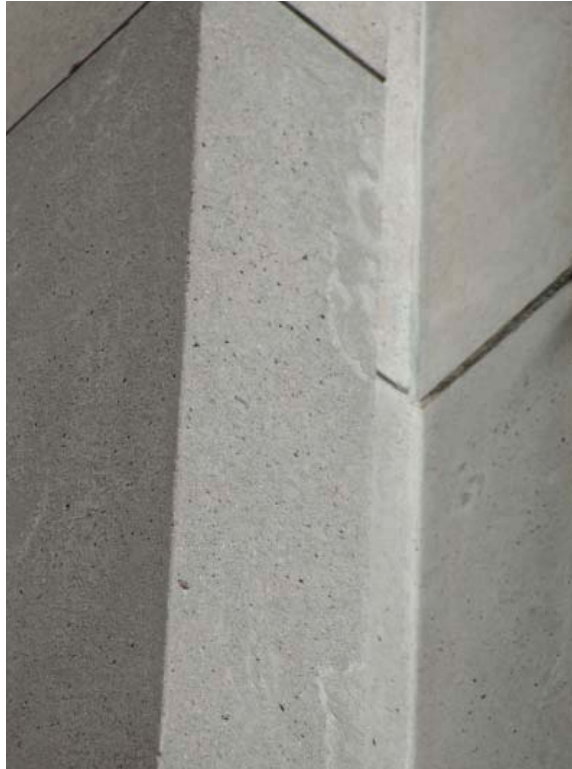
Figure 5.32- Repair on the edge of column flange.
