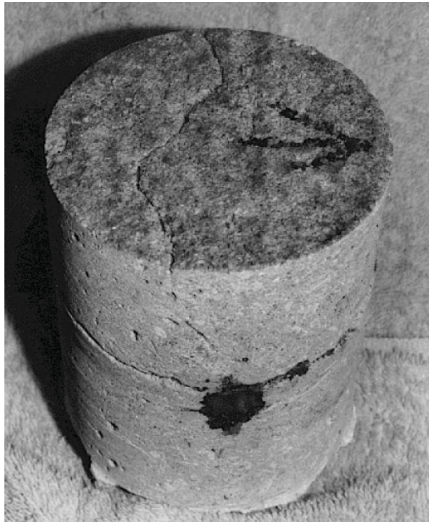
Figure 4.2- Example of a core sample showing corroded reinforcement and cracks. (Walker, Lane and Stutzman, 2006)
