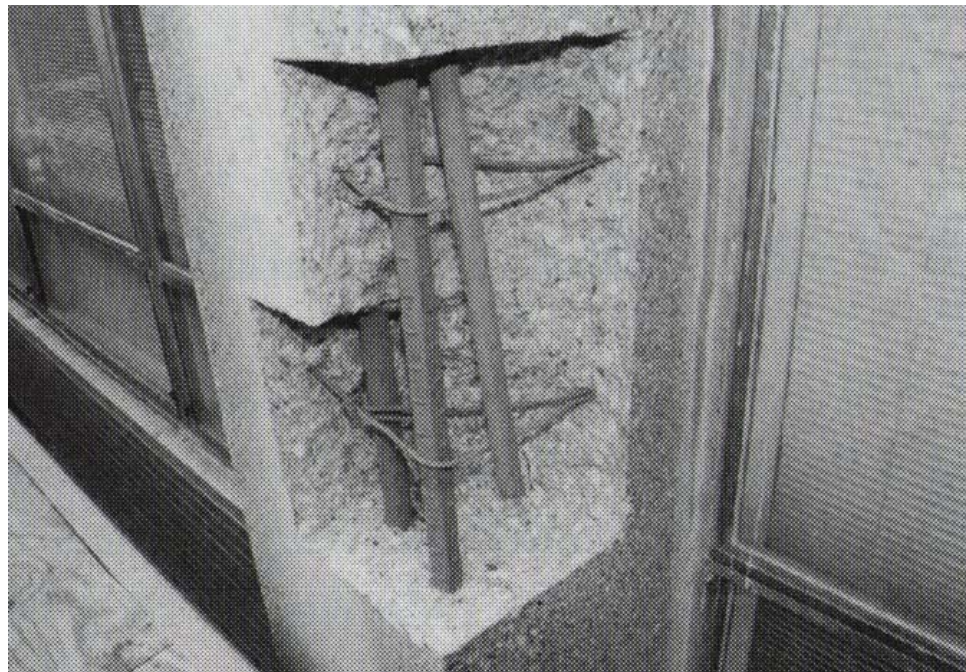
Figure 3.4- Preparation of damaged area to be repaired by patching. (Macdonald, 2003)
