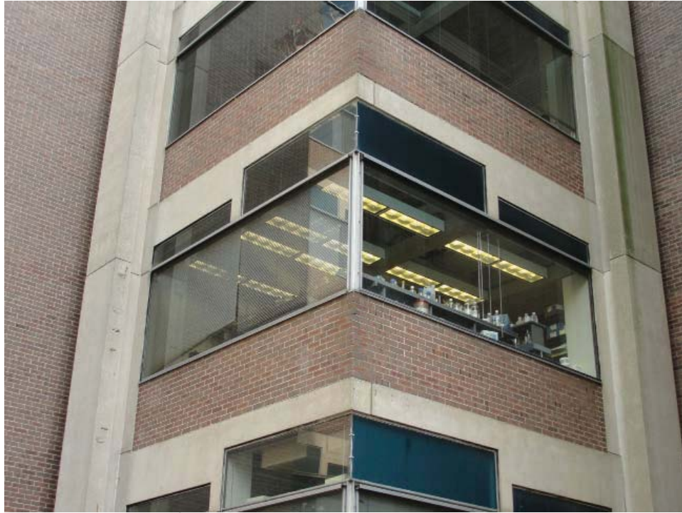
Figure 5.20- Detail of corner window and brick masonry wall.
