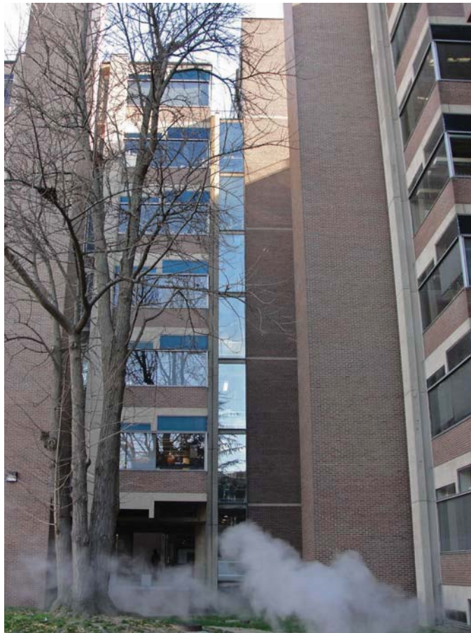
Figure 5.10- Enclosed bridge between towers B and X.
