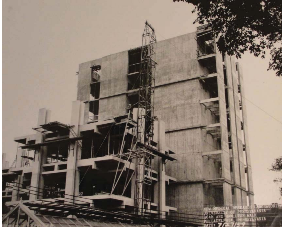
Figure 5.11- Construction photograph showing tower X's cast-in-place structure. (The Architectural Archive, University of Pennsylvania, 030.IV.A.490.12.42)
