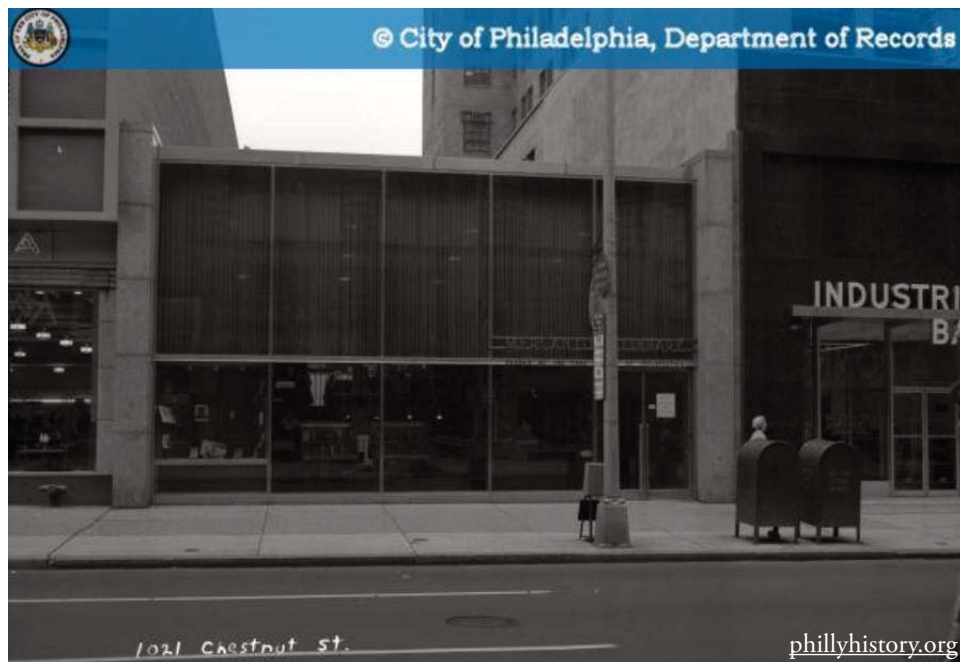
Fig. 4: The Mercantile Library (Martin, Stewart and Noble, 1954) a Center City branch of the Free Library of Philadelphia, won the Philadelphia Chapter AIA Gold Medal of 1954, as well as the AIA's Pittsburgh Plate Glass Award. It was the first postwar building added to the Philadelphia Register, in 1990.
