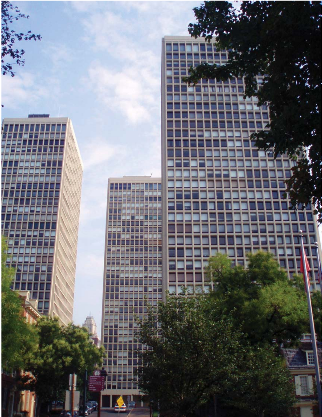
Fig. 11: The Society Hill Towers (I. M. Pei and Associates, 1964) at 200-20 Locust Street.
