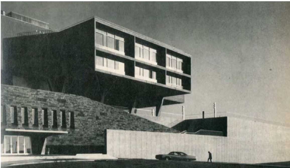
Fig. 12. Milwaukee Art Center Addition (1975). The relationship of the new addition to Saarinen's original building and to the street entry.
