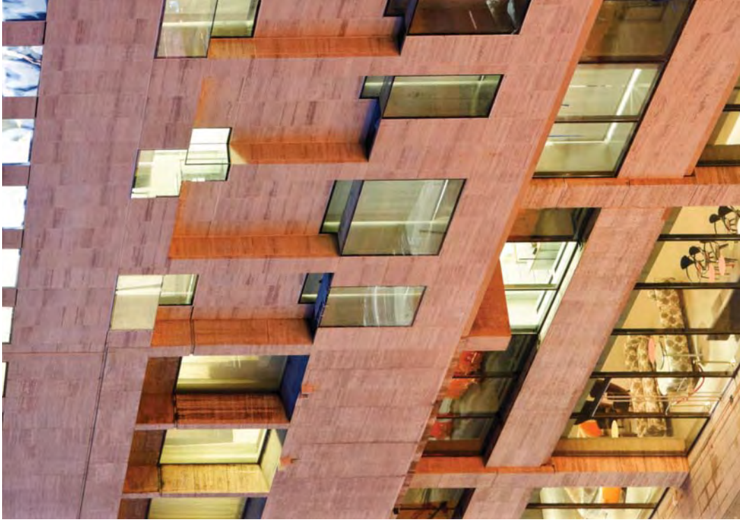
Fig. 204. Julliard and Alice Tully Hall Addition (1969). The contexted ground: 1969 meets 2009 in travertine. The glazed moments denote the 'new' portion and express differing floor levels.
