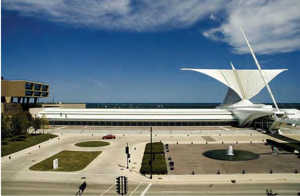
Fig. 13. Milwaukee Art Museum (2001). Santiago Calatrava's recent addition to the complex, creating a brand new entry for the museum complete with signature footbridge and dynamic brise-soleil, seen flying here.
