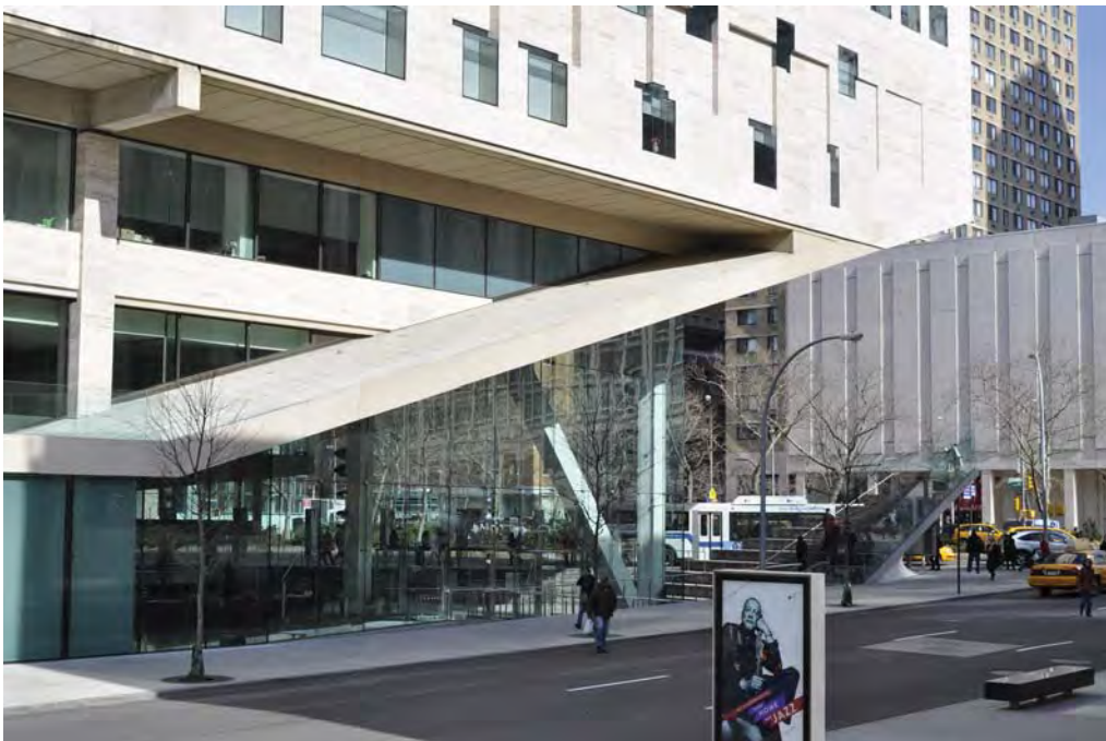
Fig. 214. Juilliard and Alice Tully Hall Addition (2009), southeast corner. The launch of the new addition. The single pier seen at left is original: it is the corner pier in Fig. 213 above.
