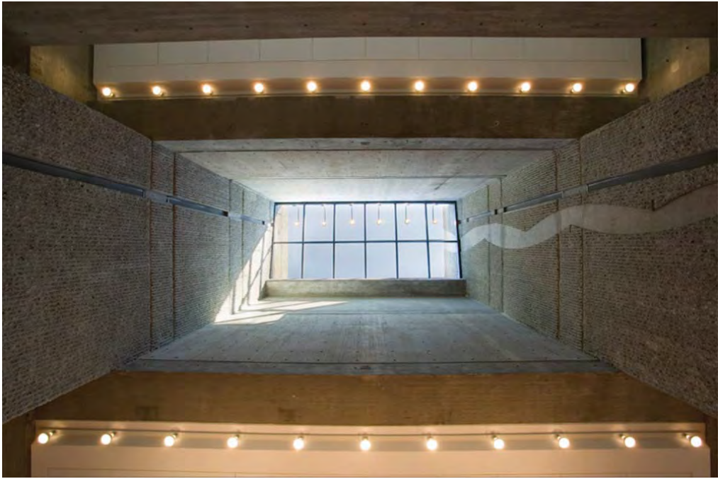
Fig. 138. Yale A&A Renovation (2008), light well. The lightwells that illuminate the fourth and fifth floors were uncovered after several decades. Here, Le Corbusier's modular snake runs up the wall.
