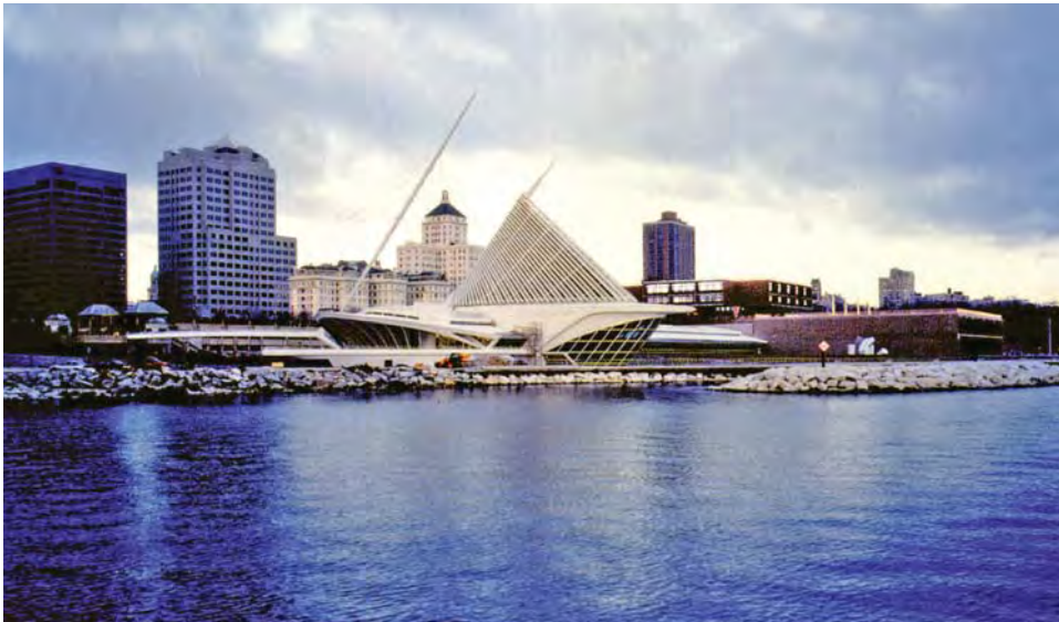
Fig. 14. Milwaukee Art Museum (2001). Calatrava's addition seen from Lake Michigan, with the 1975 addition and original 1957 building to the right.
