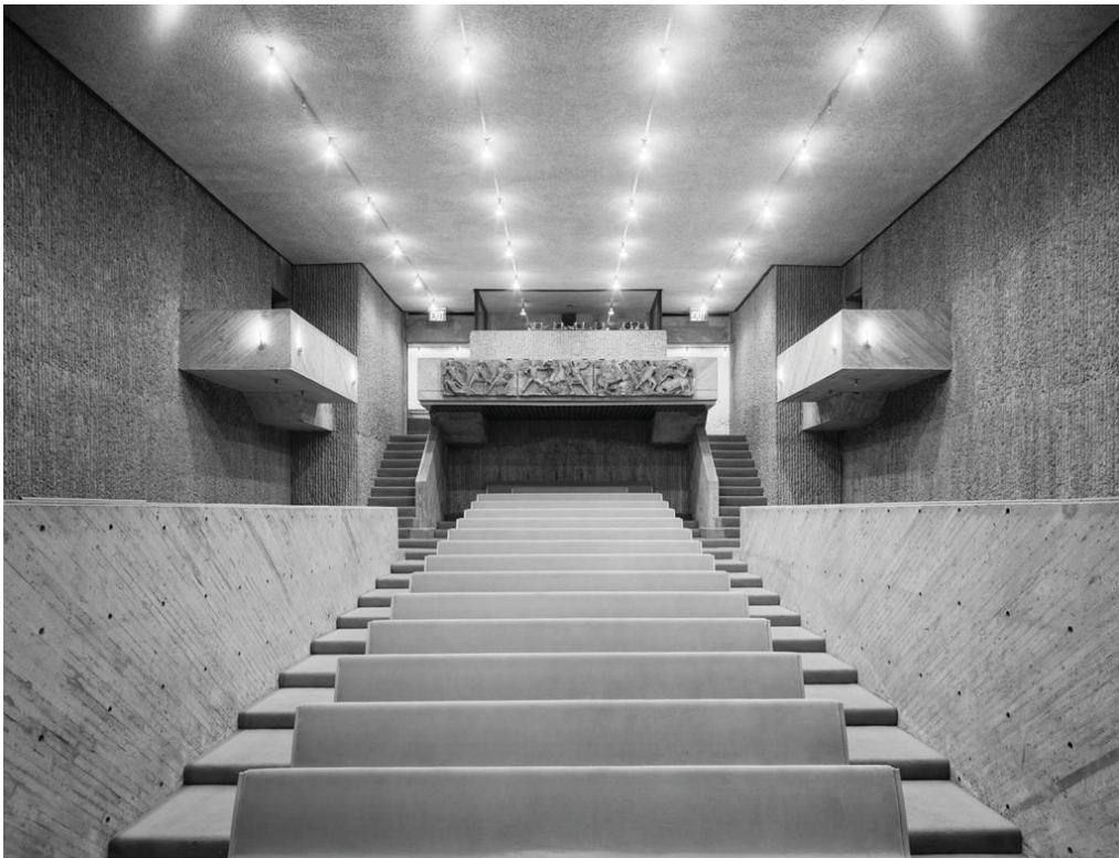
Fig. 121. Yale A&A (1963), main lecture hall. Concrete, either corduroyed or board-formed, covers almost every vertical surface. Casting of Greek frieze on balcony railing.
