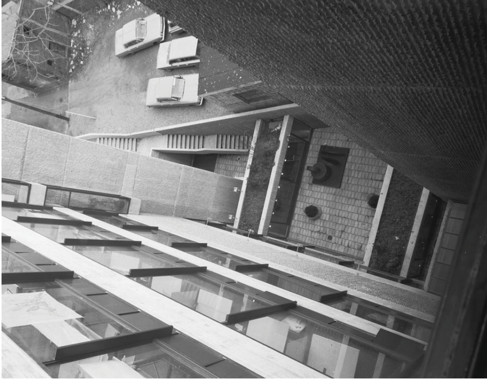
Fig. 123. Yale A&A (1963), north "courtyards." Rudolph's vertically complex sunken spaces. Largely dismantled in the 1970's, this area became the lower floor of Gwathmey's double-height library court.
