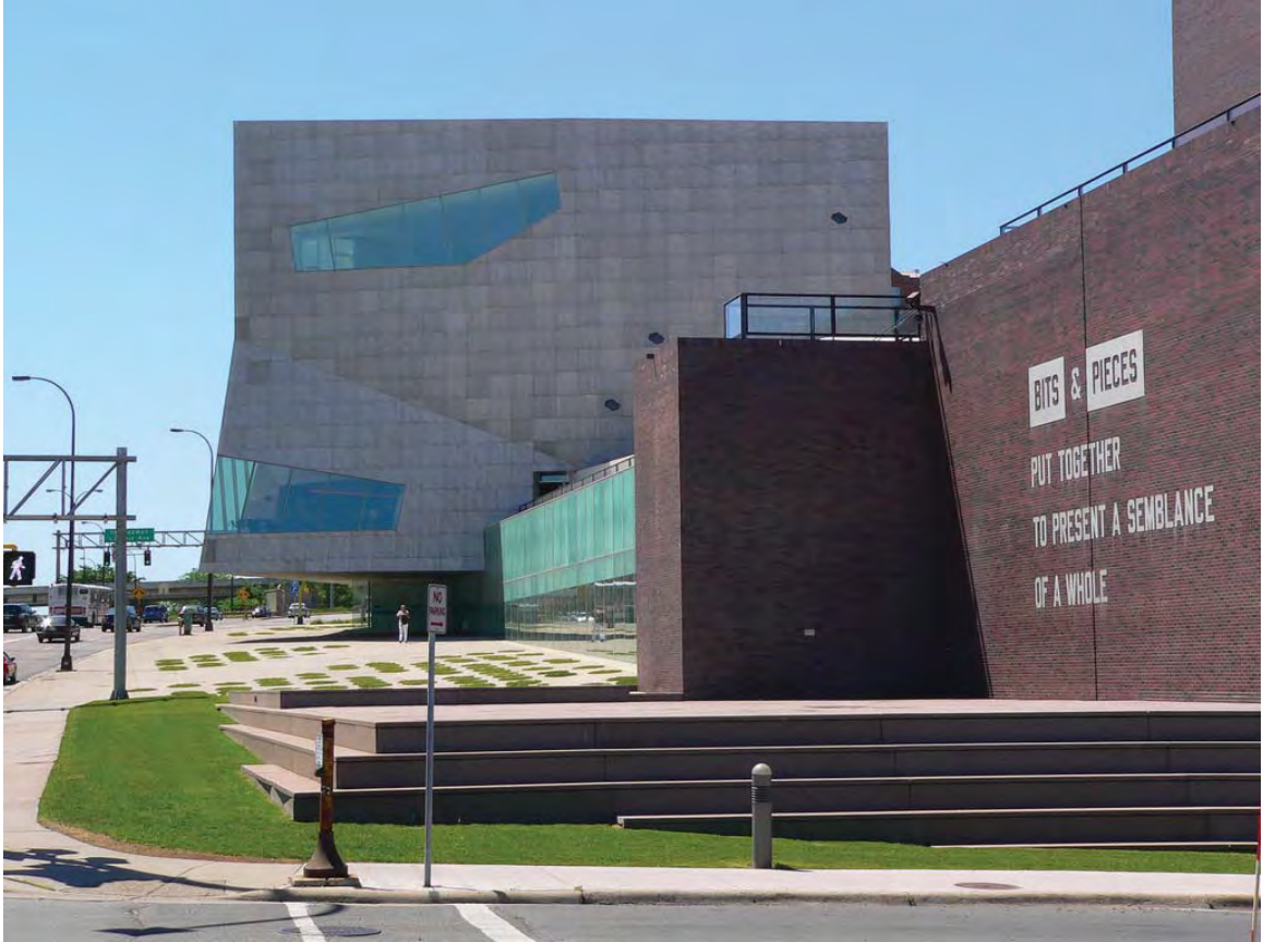
Fig. 5. Walker Art Center (east elevation). Herzog + de Meuron's zinc-clad 2005 addition to Edward Larrabee Barnes' 1971 building is a set of similar massings radiating from a connecting glazed concourse.
