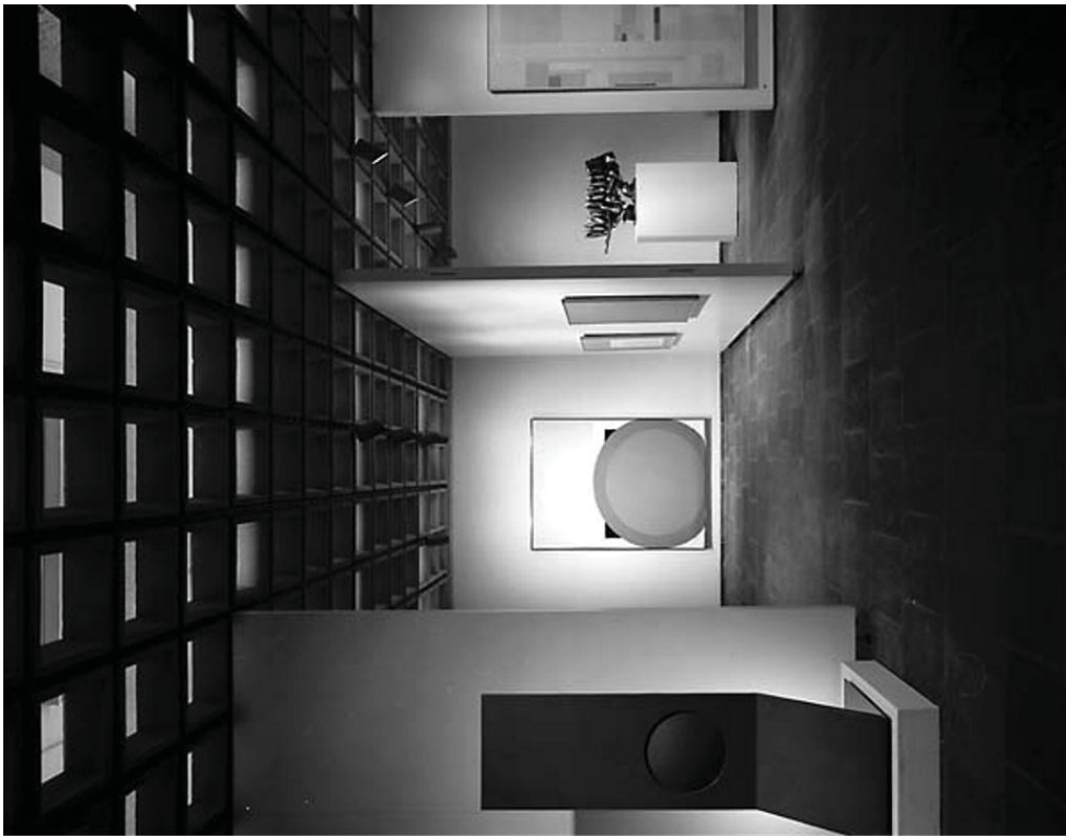
Fig. 71. Whitney Museum (1966), Interior. Breuer employed a modular gridded ceiling system that carried moveable partitions and lighting. The floors are stone.
