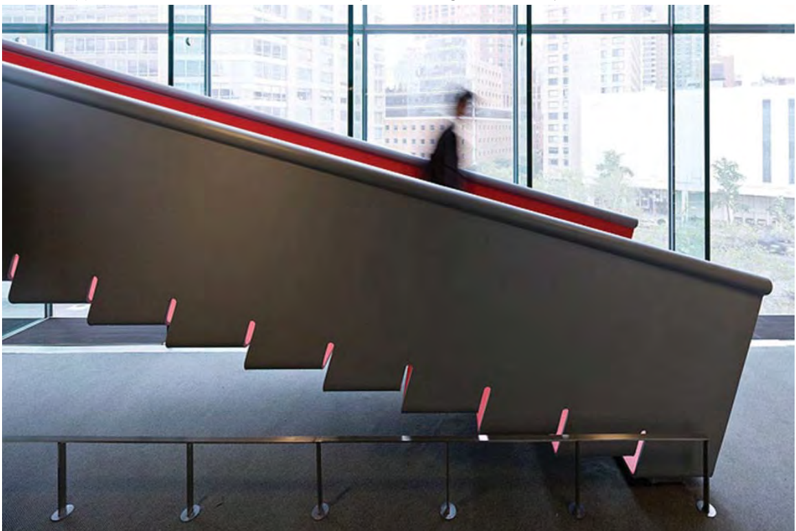
Fig. 212. Juilliard School Addition (2009). One of the addition stairs, cut and bent from a single piece of steel, it appears as a single, ad-hoc element.
