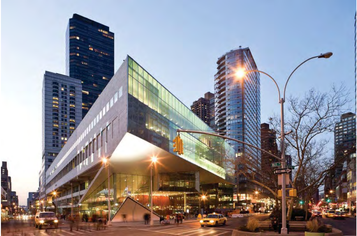
Fig. 168. Juilliard and Alice Tully Hall Addition (2009), street view. The new Broadway facade, with 65th Street receding at left. Note slight line in the travertine revealing the new cladding, upper left.
