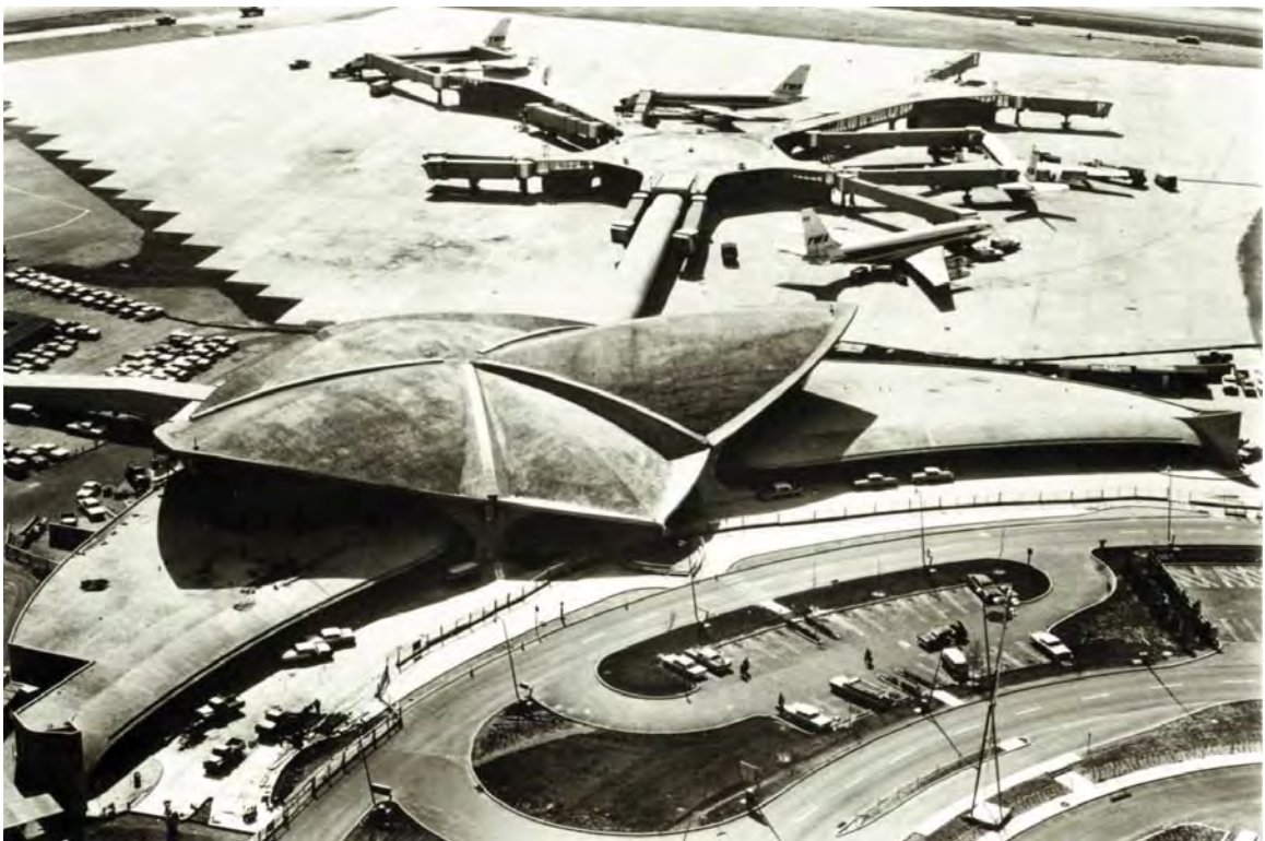
Fig. 29. TWA Flight Center, Idlewild Airport, New York (1962). This aerial photograph of Saarinen's terminal shows the relationship of the main terminal with curbside arrival to the flight "tubes," leading to the two gate lounges. Also visible in the terminal roof are the articulated skylights between roof shells.
