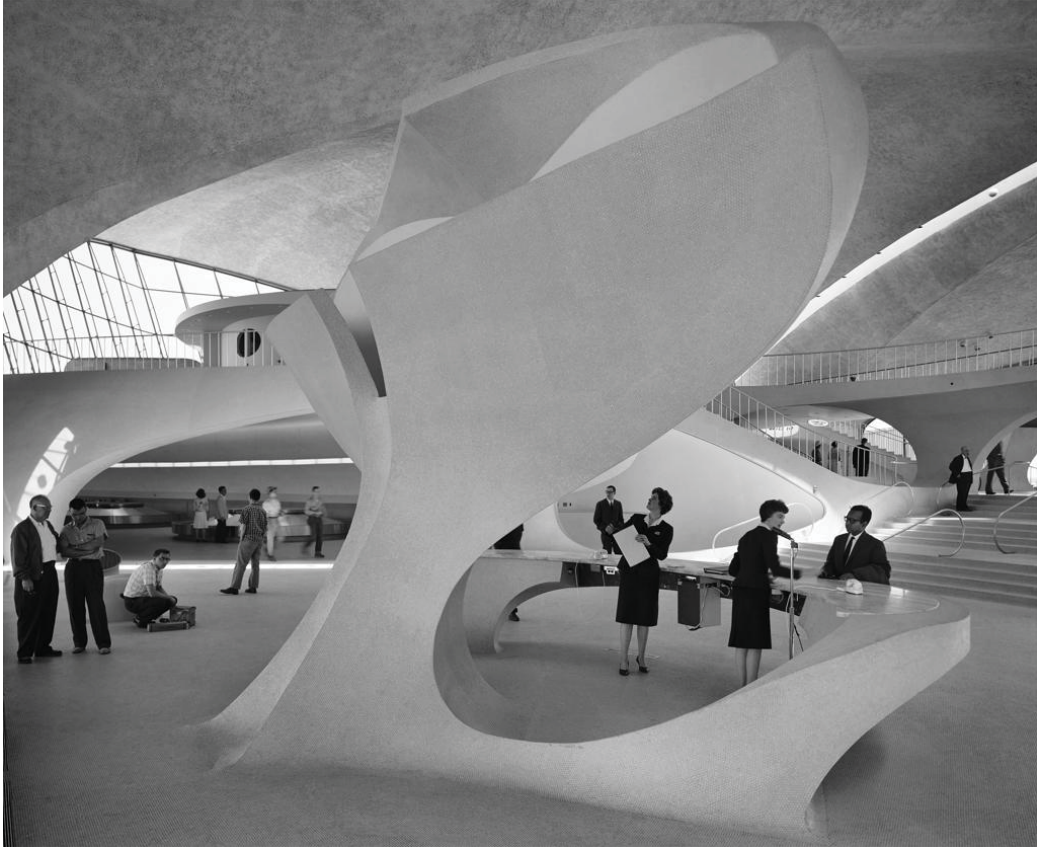
Fig. 30. TWA Flight Center (1962) - Interior view. The information desk, like many elements of the terminal interior, were designed through iterative physical modeling rather than through plan and section.
