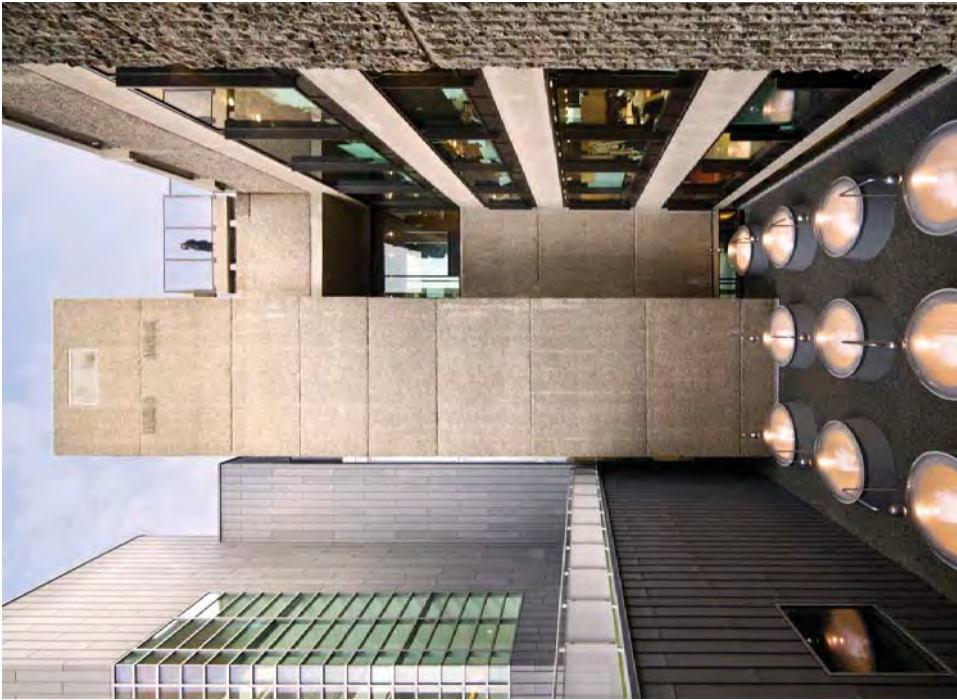
Fig. 149. Yale A&A and Loria Center addition (2008), library roof. The new, enclosed triple-height library court is lit by a series of bubble-like skylights. The landscaped roof is a level above; at left. The window at lower-left aligns another, offering a glimpse of the A&A.
