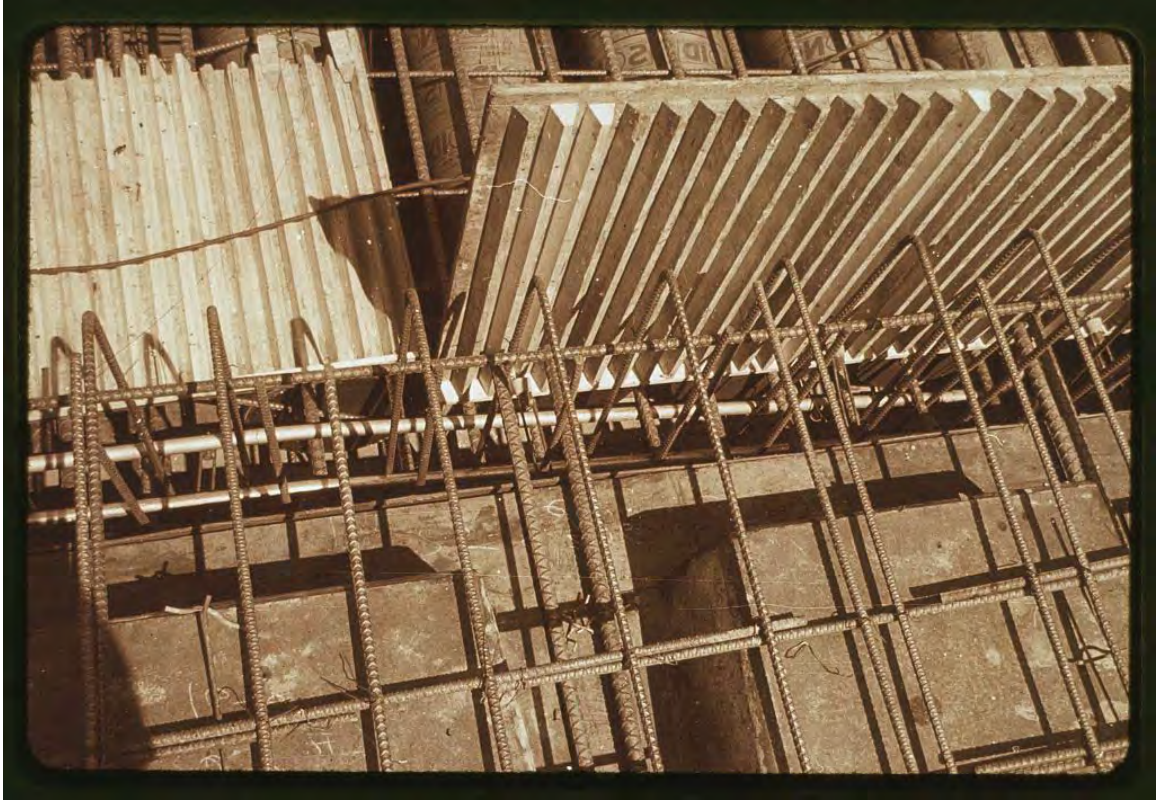
Fig. 104. Yale A&A (1963), process. The corduroy mold that gave the concrete its texture. After the concrete had set, the ribs were painstakingly knocked back with hammers to expose the aggregate.
