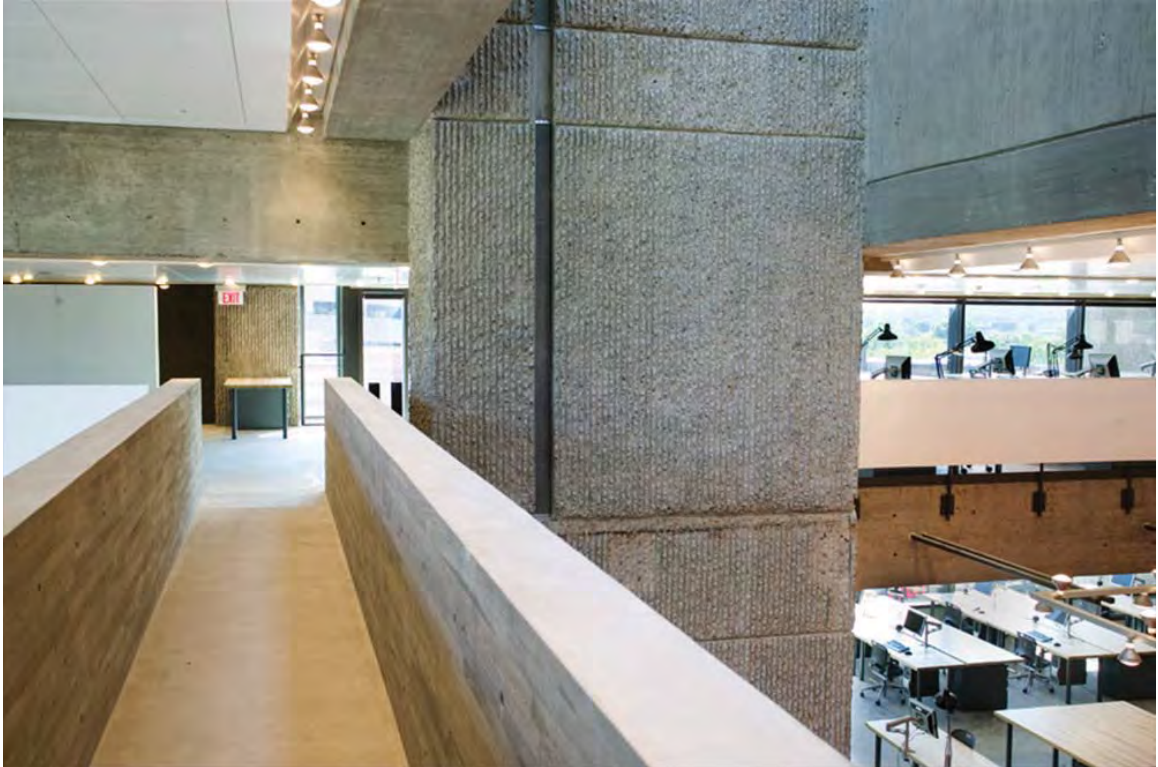
Fig. I35. Yale A&A Renovation (2008), west U-channel bridge. Gwathmey restored Rudolph's narrow bridge (making it flush with the fifth floor), and installed his own at the east end of the studio.
