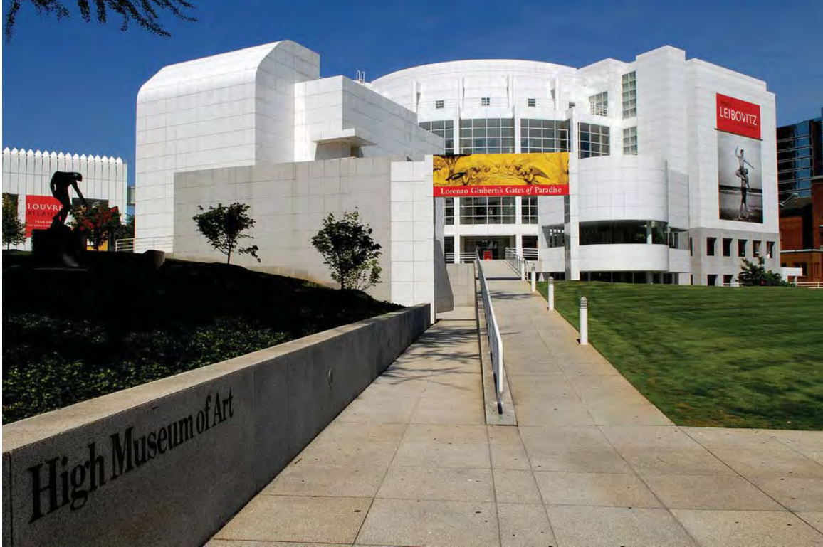
Fig. 45. High Museum of Art, Atlanta, Georgia. Richard Meier's white temple (1983) viewed from the building's organizing ramp. At left, in the background, is one of Renzo Piano's pavilions (2002 addition).
