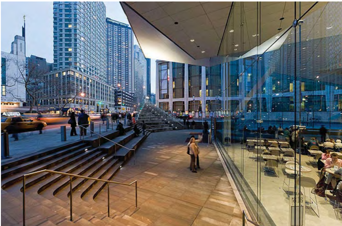
Fig. 192. Alice Tully Hall Addition (2009), plaza. The hardscape that mediates between sidewalk level and the lobby below. Note the minimal construction detailing on the mullion-less glass curtain wall.
