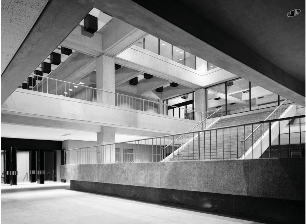
Fig. 215. Juilliard School (1969). Belluschi's principal entry lobby for the school on 65th Street, located on the first floor with the entry doors beneath the Milstein bridge. Significantly altered in the 1990's when principal the entry was moved to the plaza level above and a recital hall was carved out of the space.
