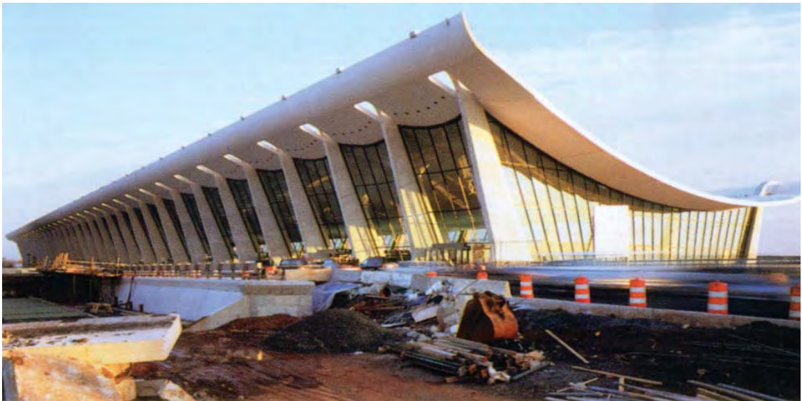
Fig. 25. Dulles Airport Expansion (1997). Skidmore Owings and Merrill's 1997 expansion of Saarinen's landmark terminal increased the original building from 15 bays to 31.
