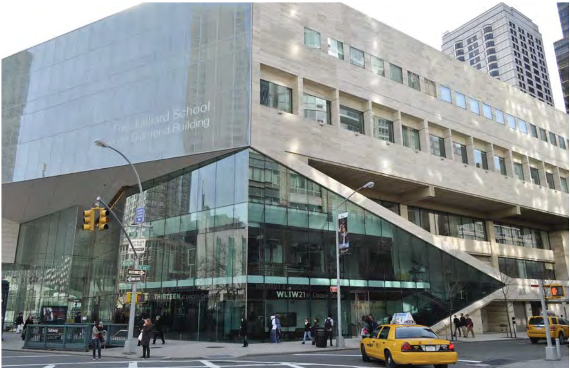
Fig. 200. Juilliard and Alice Tully Hall Addition (2009), street view. The northeast corner of the building. The upper travertine is original, but the inclined planes that split from the terrace railing below this cantilever are part of the addition. A public television studio occupies this lower portion of the addition.
