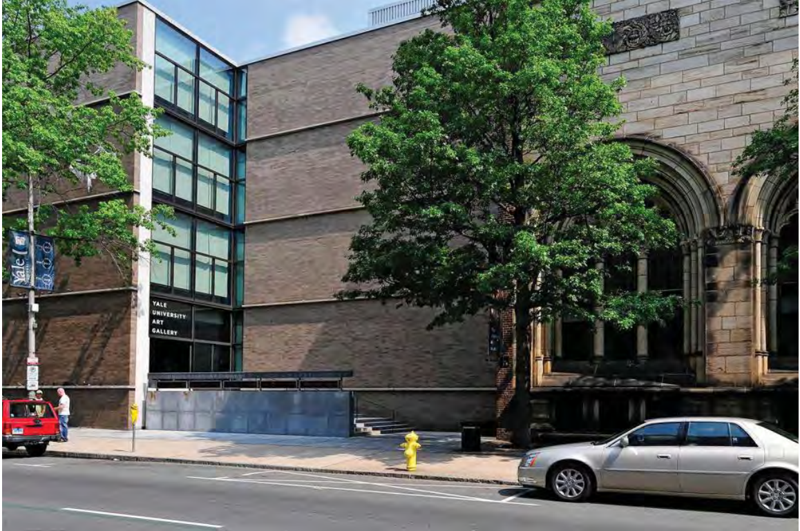
Fig. 2. Louis Kahn's Yale University Art Gallery, 1953. Egerton Swartwout's 1928 building is to the right.
