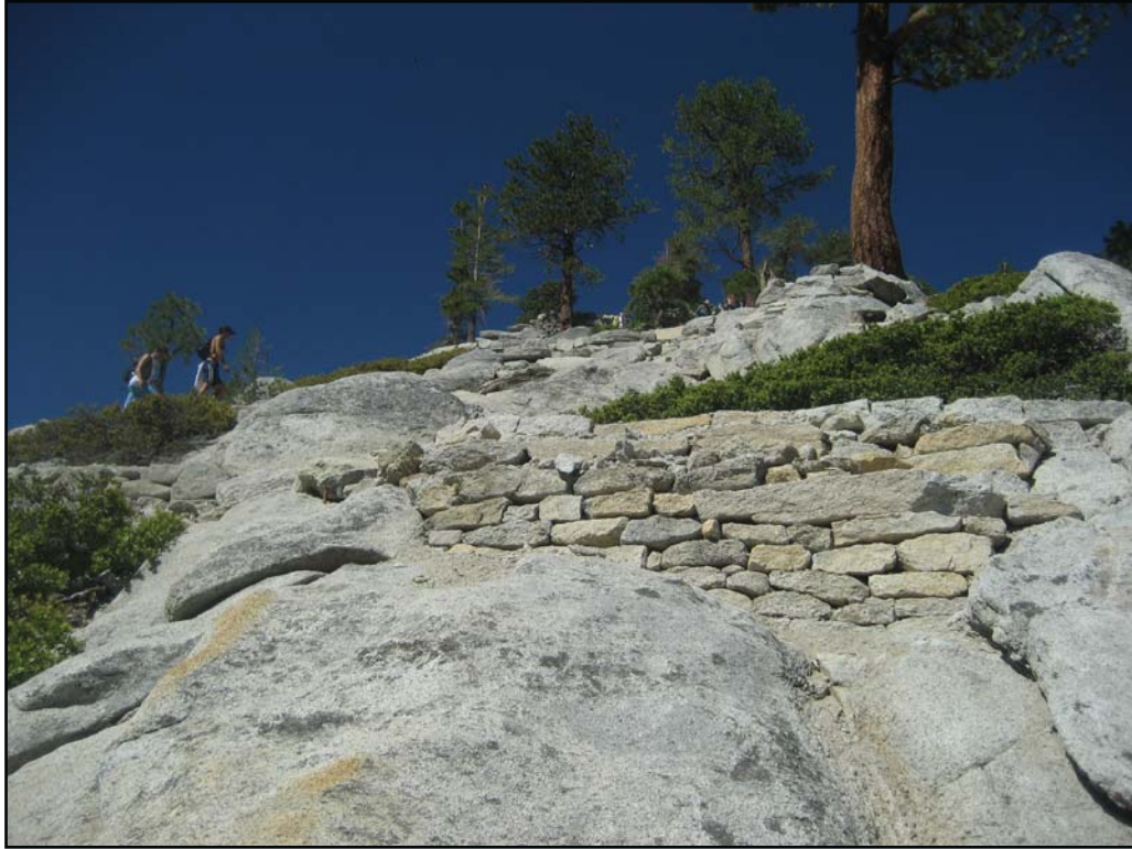
Fig. 4.1 Granite retaining wall on Half Dome Trail, July 2010. Source: Photograph by Alison Swing.
