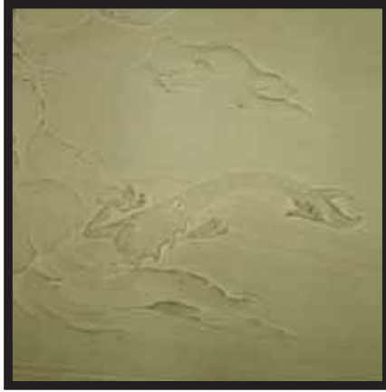
(a) soiling along high relief
