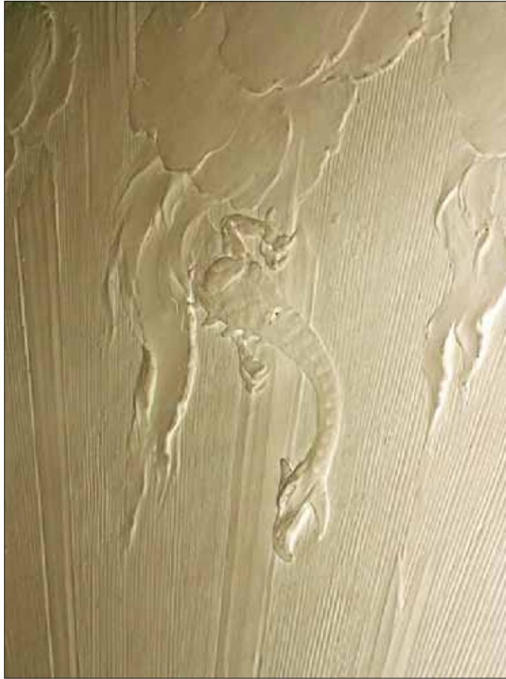
Figure 5.5. Griffin (relief appliqué) with exposed nail used to fix piece. The over tooled background surface (in situ applied rays and ridges) continues under the pre-cast figure, with hand-applied relief-work (flames and clouds) used to conceal the edges of the appliqué (L. Vollono, 2009).
