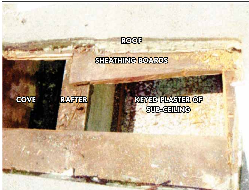
Figure 5.3. Roof probe towards the west wall, with cove to the far left, roof rafter and keyed plaster of sub-ceiling in the center (Kaitsen-Woo, 2008).
