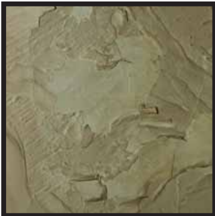
(b) extensive paint flaking
