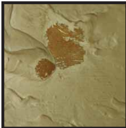
(c) evidence of former paint reveals
