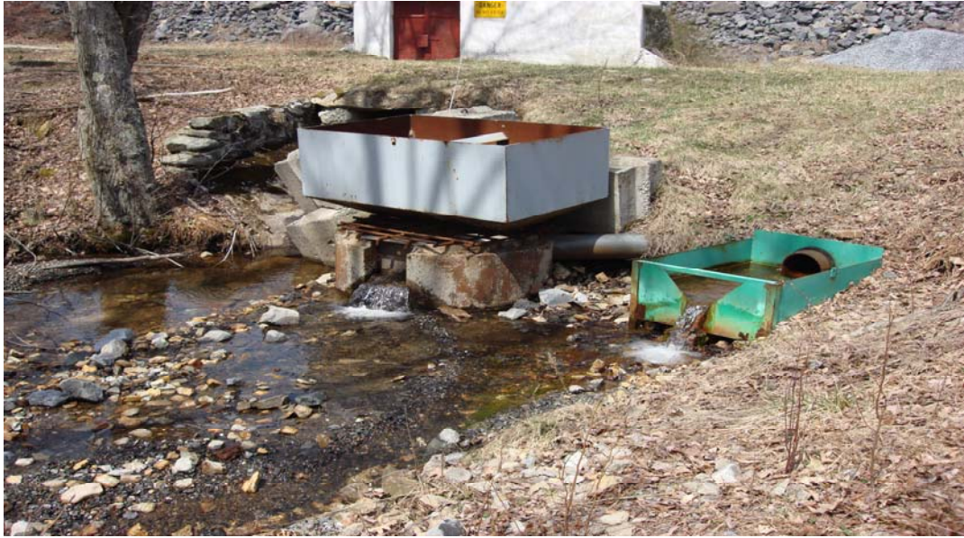
Figure 19: Another view of the Dyer Run Diversion Wells
