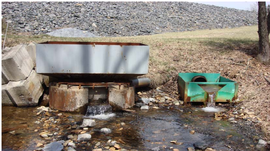
Figure 18: Small scale diversion wells at Dyer's Run. The limestone is contained in the hoppers and the river is diverted over the limestone.
