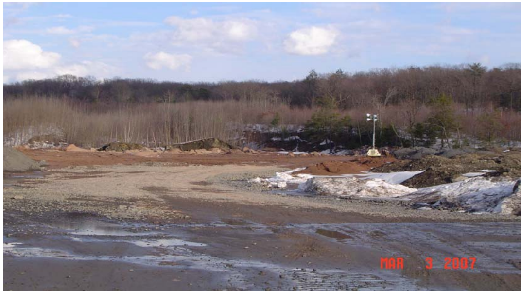
Figure 22: An area of the same mine site that has been reclaimed back to its original grade
