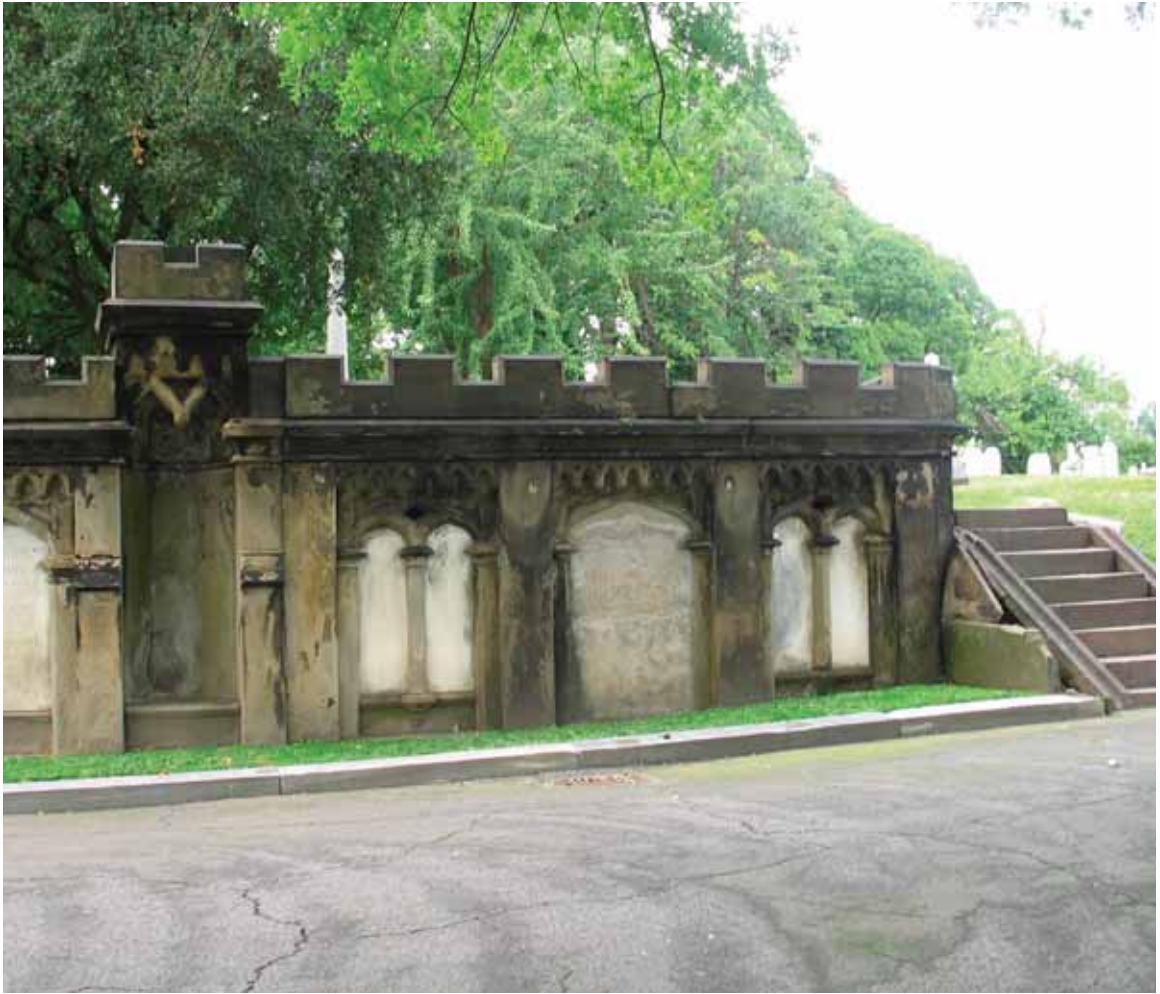
Figure 2.9 Suddards-Manuel-Clark monument, Clark (east) section (Source: E. Kemery, 2008)
