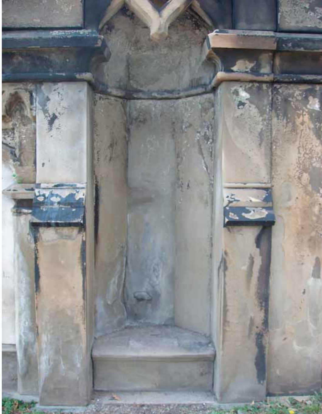
Figure 7.6 Cove area after cleaning with Cathedral Stone® Products D/2 Biological Solution (Source: E. Kemery, 2009)
