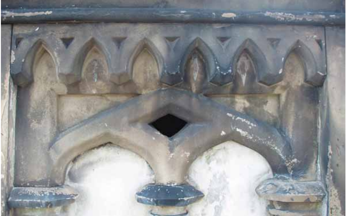
Figure 7.8 D/2 Solution removed biological growth in this area but did not remove other soiling (Source: E. Kemery, 2009)
