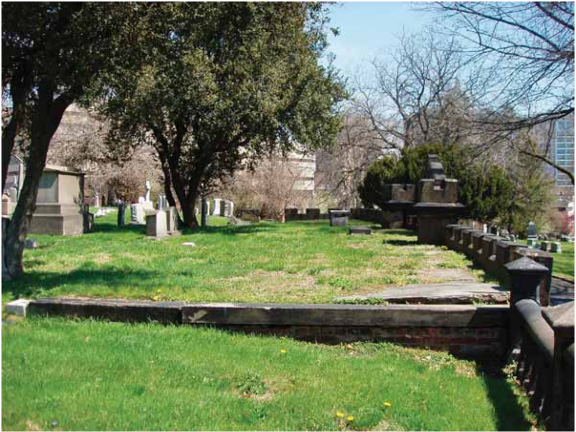
Figure 6.6 Top of the Suddards-Manuel-Clark monument, note slate paving stones in foreground and ventilation sources at center (Source: E. Kemery, 2009)
