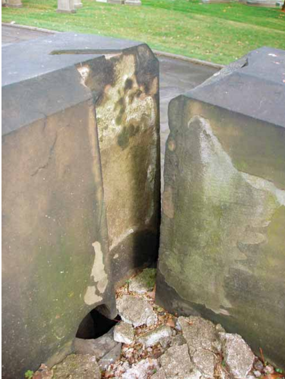
Figure 6.15 East corner of the Suddards-Manuel-Clark monument, gutter drain hole and evidence of a strap that held these two blocks together (Source: E. Kemery, 2008)
