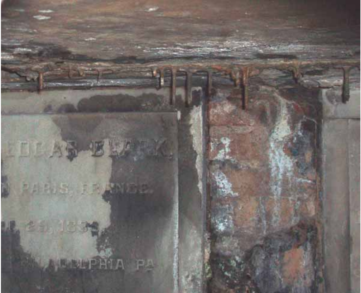
Figure 6.3 Interior of Suddards-Manuel-Clark vault showing black biological colonization (Source: E. Kemery, 2009)
