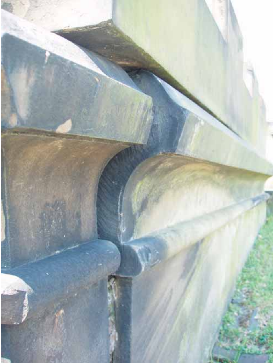
Figure 2.11 Toolmarks visible on east wall open joint (Source: E. Kemery, 2009)
