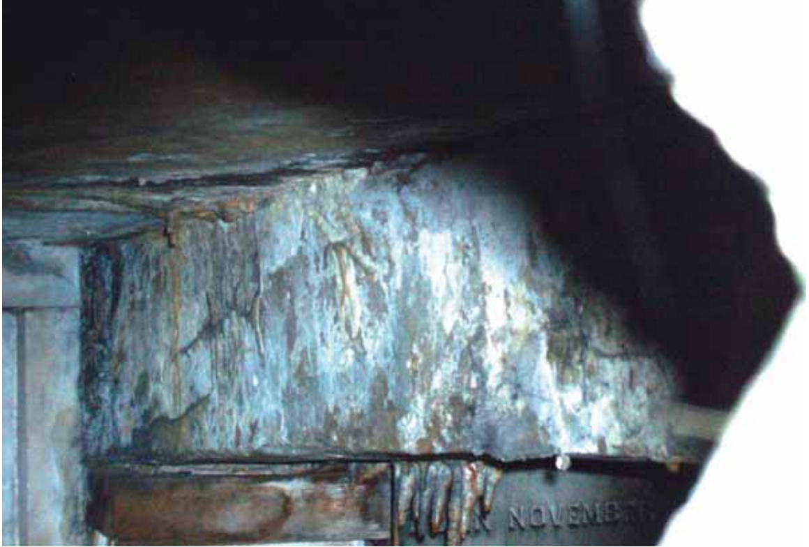
Figure 6.4 Interior of Suddards-Manuel-Clark vault showing stalactites and calcite buildup (Source: E. Kemery, 2009)
