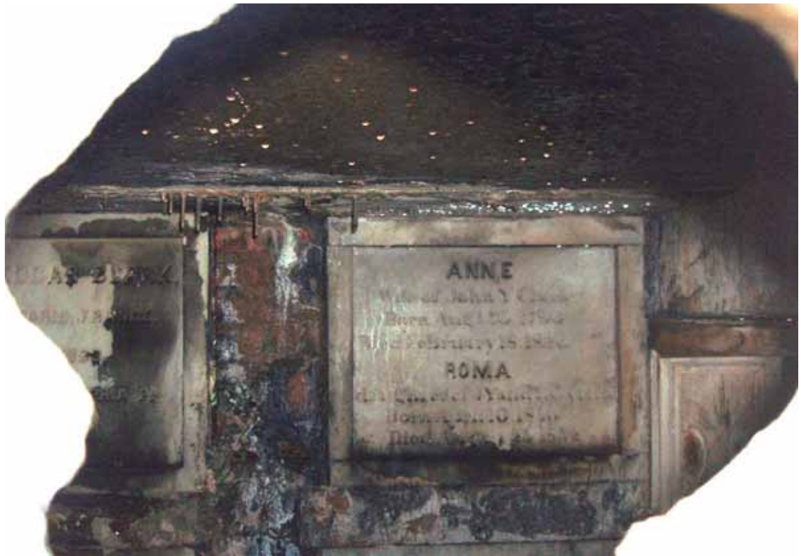
Figure 6.9 Interior of Suddards-Manuel-Clark vault under wet conditions (Source: E. Kemery, 2008)
