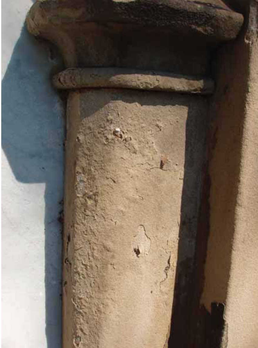
Figure 4.1 Sample area of flaking (Source: E. Kemery, 2009)
