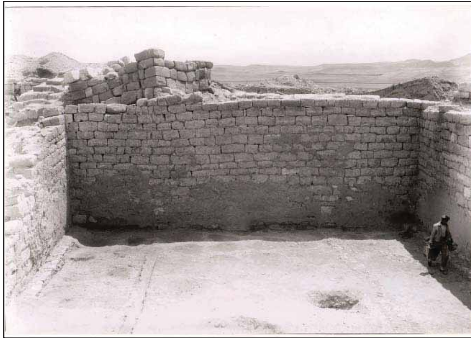
Figure 34. East interior wall of the North Court with shear cracks from the remaining Middle Phrygian wall. From the Gordion Archives, ca. 1955.
