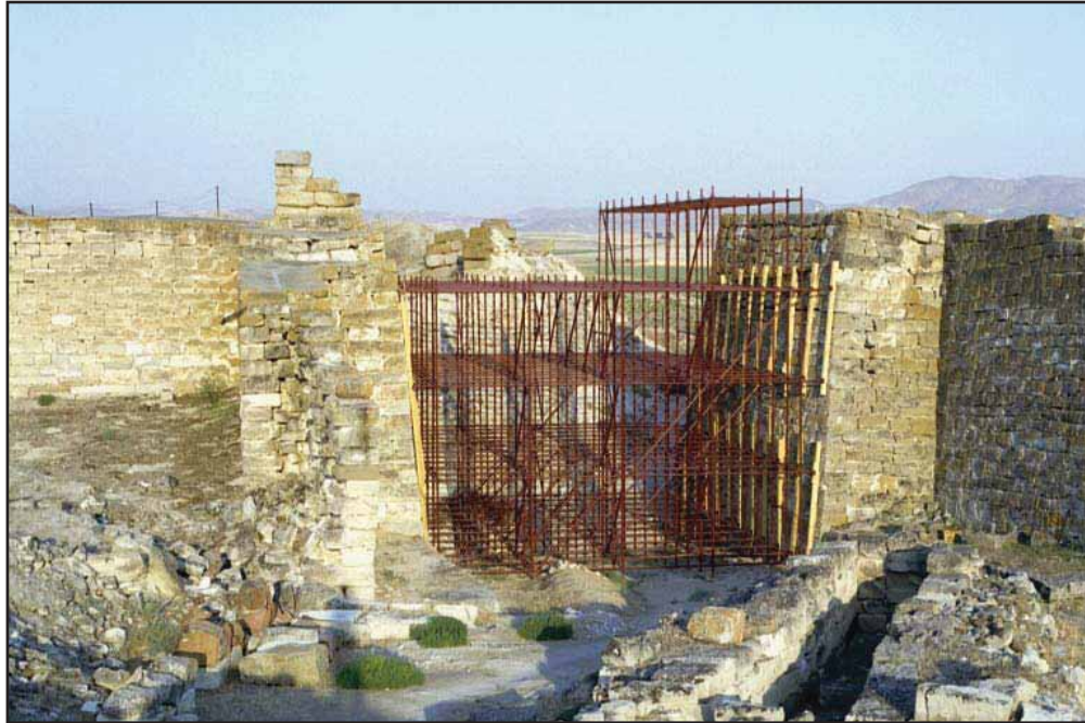
Figure 14. The scaffolding erected after the Izmit earthquake. By Goodman, 2001.
