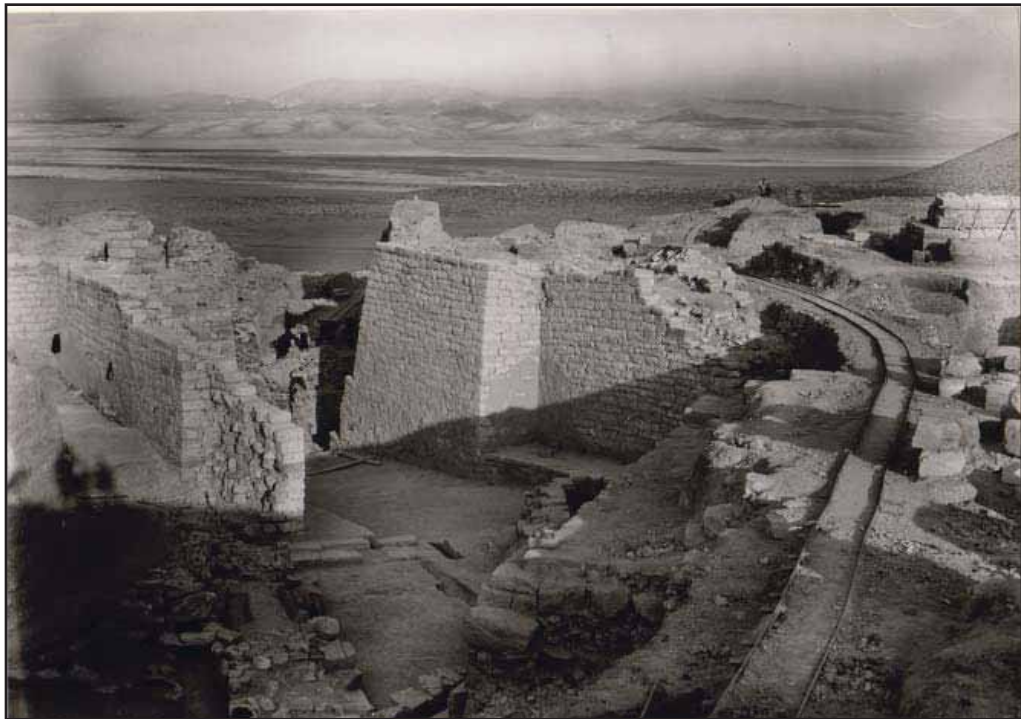
Figure 12. The Polychrome House foundations were uncovered at the interior of the main entryway. From the Gordion Archives, ca. 1955.
