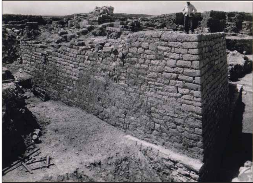
Figure 37. The east elevation of the South Court shows missing stones and depressions in several areas. From the Gordion Archives, ca. 1955.
