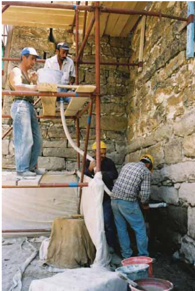
Figure 15. Gravity grouting process applied to the South Court. By Goodman, 2001.
