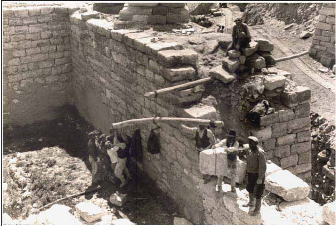
Figure 11. Reconstruction of the southwest elevation of the North Court. From the Gordion Archives, ca. 1955.
