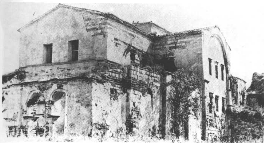
3 Enez. View from southwest
