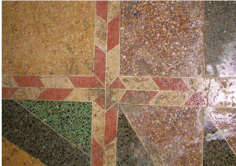
Figure 8: The terrazzo floor in the lobby of the East Columbia Building before conservation. Source: Andrea Morse, Sculpture Conservation Studios.
