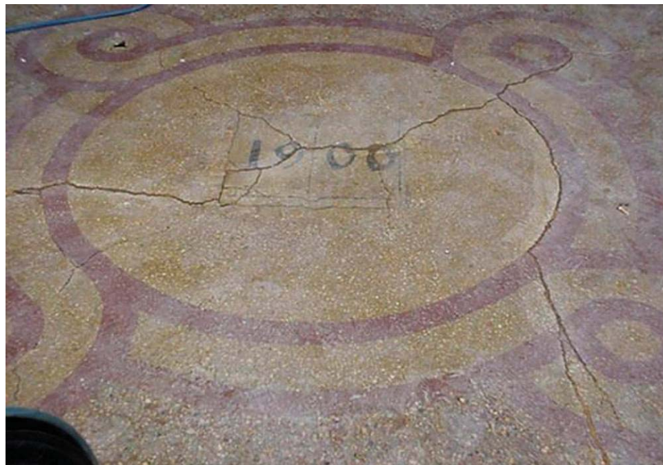
Figure 6: After restoration of the terrazzo in St. Joseph's Library, St. Joseph Missouri. Source: http://www.ntma.com/07_2005_honor_awards_desc.php?job_name=stjoseph1
