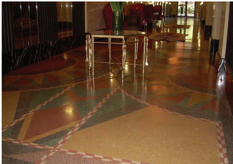
Figure 9: The terrazzo floor in the lobby of the East Columbia Building, after conservation. Source: Andrea Morse, Sculpture Conservation Studios.
