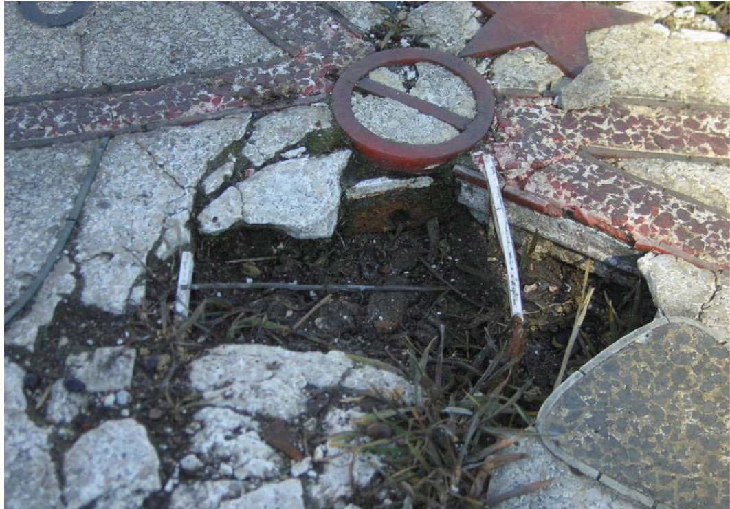
Figure 16: Detail of the insets and support system in a damage tile on site. Source: photo by author
