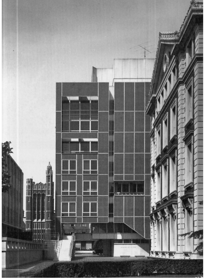
III. 8 Sherman Fairchild Center North Facade. Architecture of Additions, p.120
