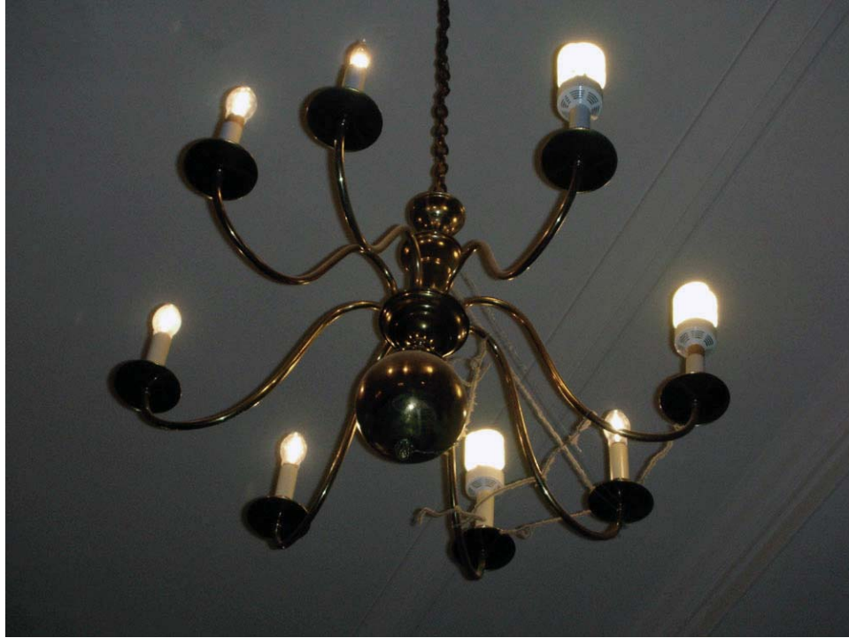
Figure 10: The addition of CFLs to this candelabra contrast starkly with the imitation candles and candelabra lamps. (Photograph by Ellen Buckley)
