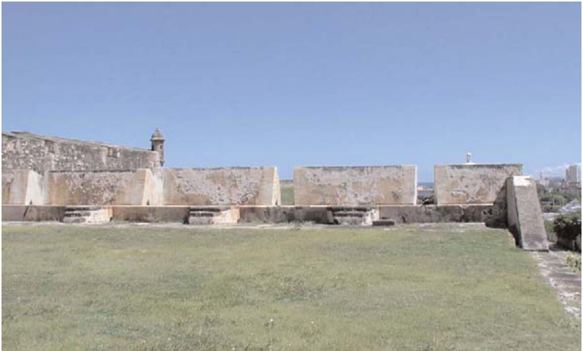
Illustration A8: South side of upper level of La Trinidad (14), facing northeast. San Carlos (13) is visible in the background.
