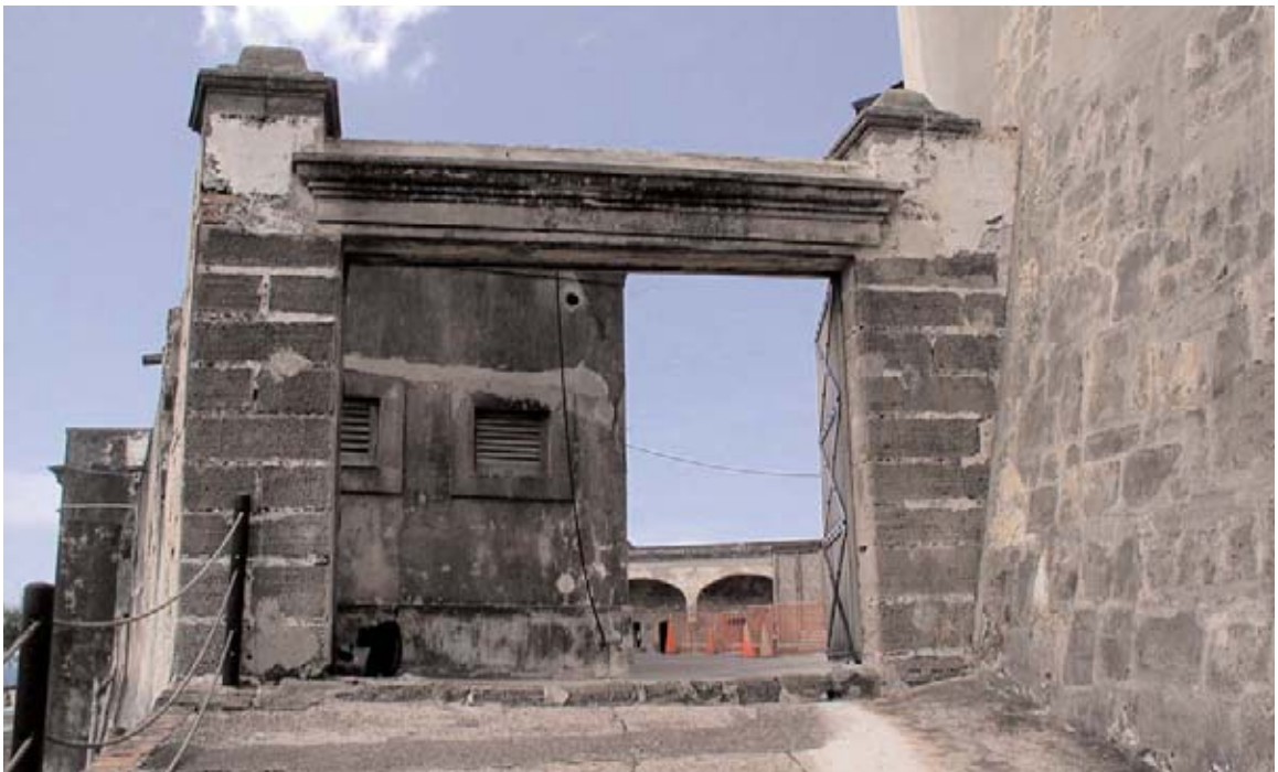
Illustration A4: South Gate (08), facing north.
