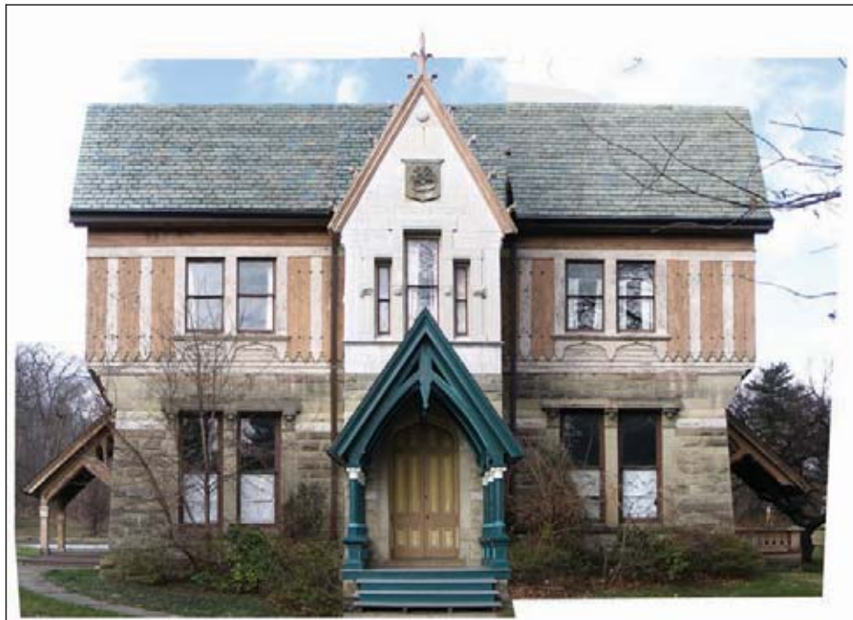
Figure 4.1: Photographic montage of south elevation.
