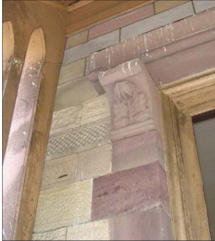
Figure 4.3: Detail various surface finishes, under porch on west elevation.
