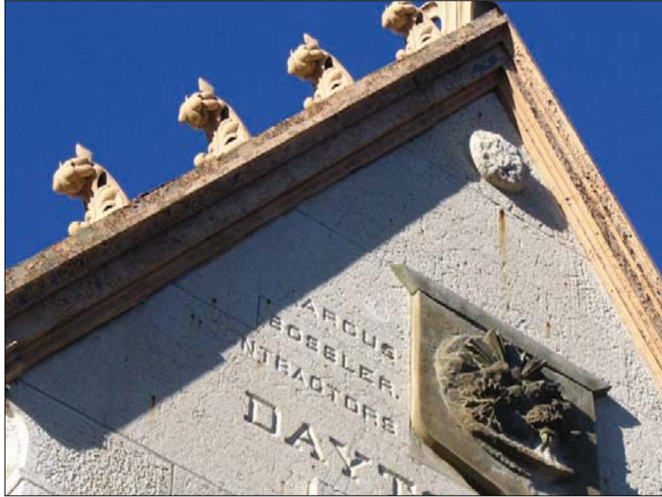
Figure 3.2: Detail of pyrite inclusions and pitting in Dayton limestone.
