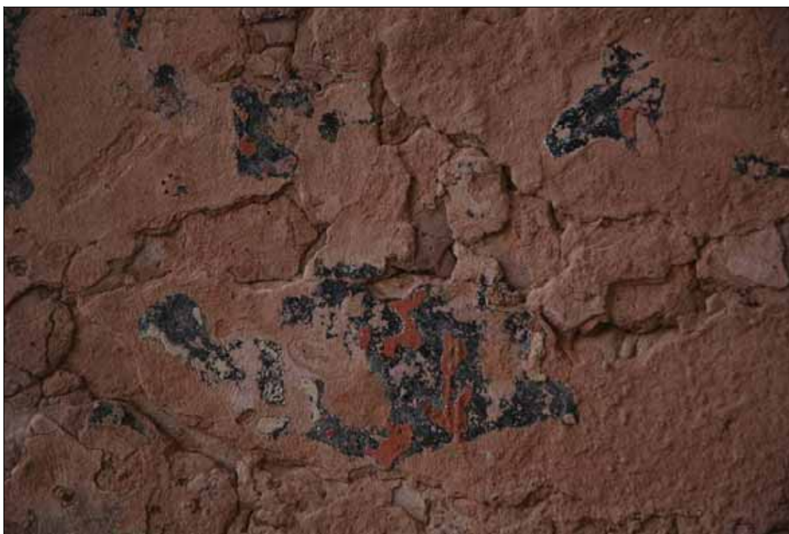
Figure 4.6. Detail of fragmentary bright red paint on the mid-face of Pilaster 1 (Ferron 2006).
