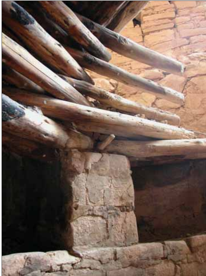
Figure 3.2. Kiva roof cribbing with vigas supported by the pilaster and resembling basketry in Cliff Palace (CASPAR 2003).
