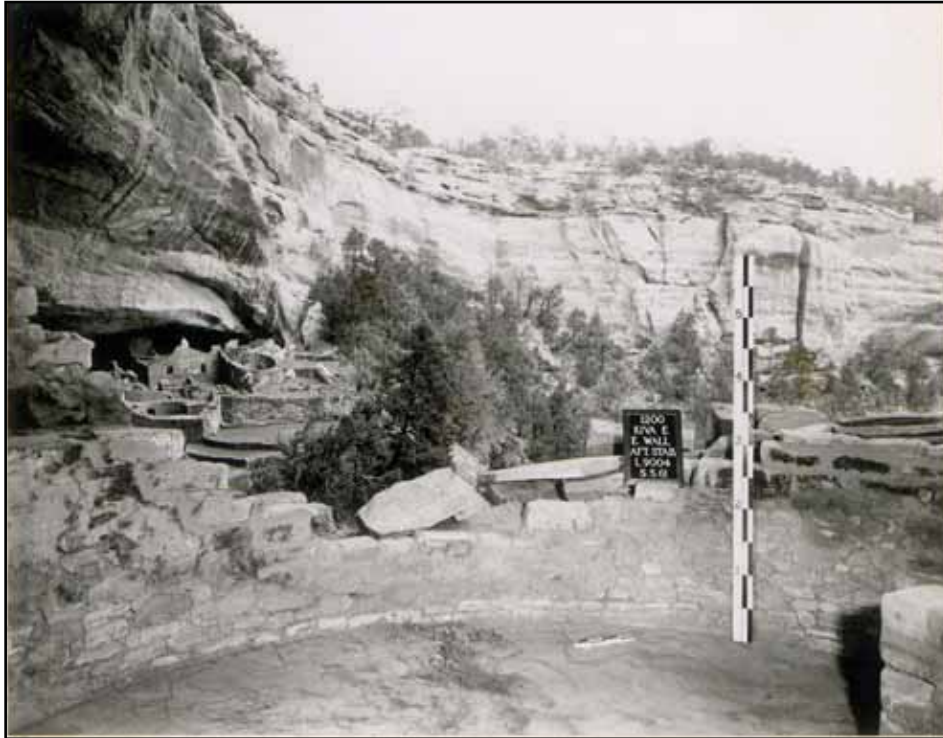
Figure A.15. Southeast wall after stabilization (Hannah 05/05/1961).
