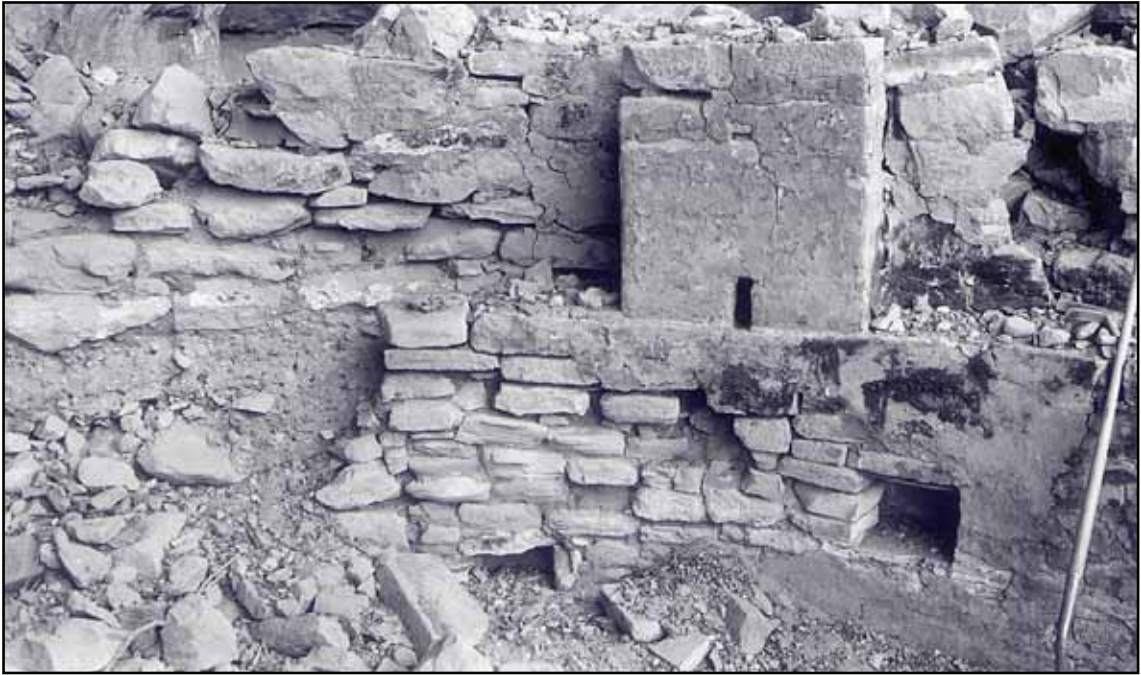
Figure A.6. Northeast wall and Pilaster 4 before excavation/stabilization (date unknown).
