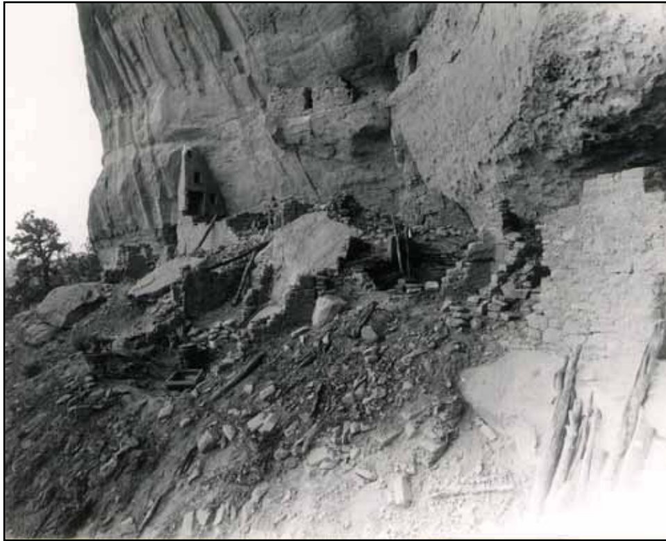
Figure A.5. General view of Long House looking west (Werner 07/02/1959).
