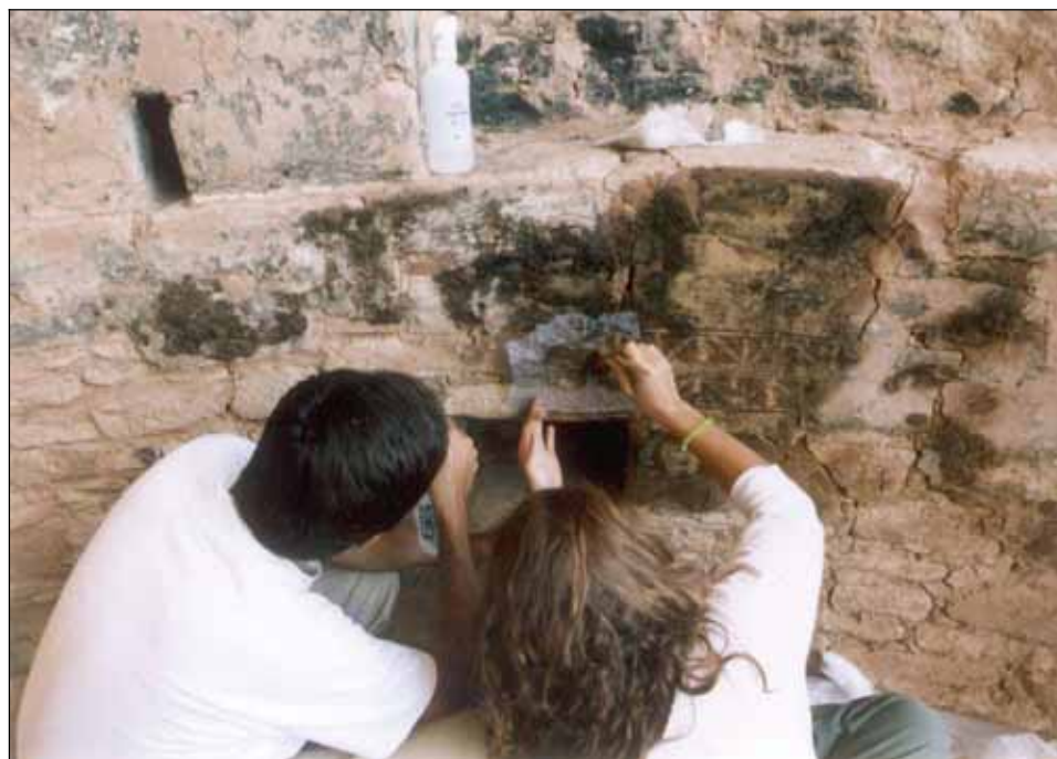
Figure 3.8. Frank Matero and Angelyn Bass Rivera treating the plasters in Kiva E (Fiero 1994).
