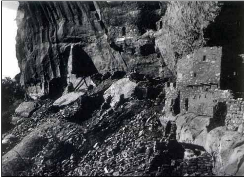
Figure A.1. Early photograph of Long House (attributed to Wetherill and Nordenskiold 1891).
