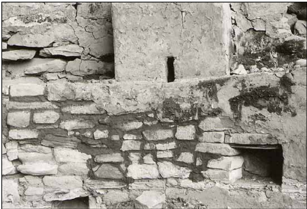
Figure A.7. Northeast wall and Pilaster 4 after stabilization (1959).
