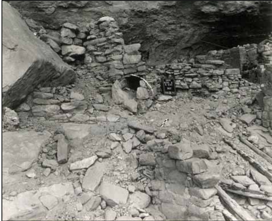
Figure A.11. Kiva E south exterior wall before excavation/stabilization (Werner 6/12/1959).
