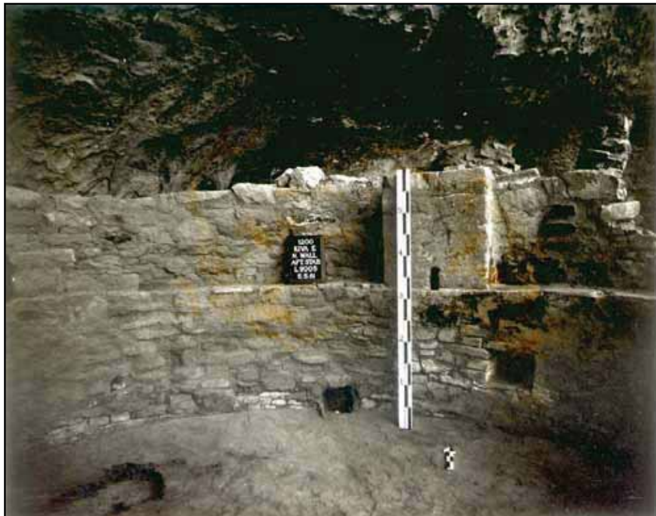
Figure A.18. North wall after reconstruction (Hannah 05/05/1961).
