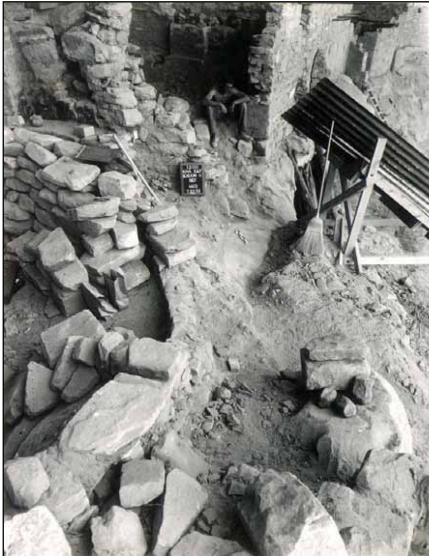
Figure A.10. Wall reconstruction between Kivas E and F (Werner 7/23/1959).
