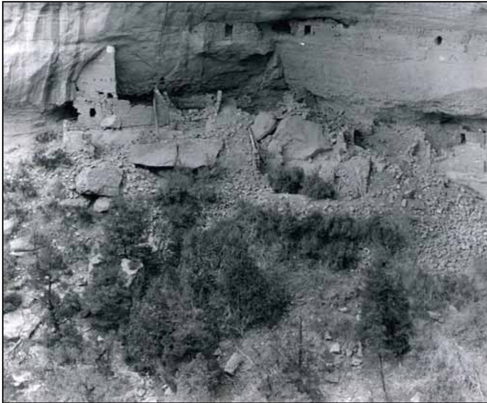
Figure A.3. Image of Long House from across the canyon before excavation during the Wetherill Mesa Project (Cattanach 11/06/1958).
