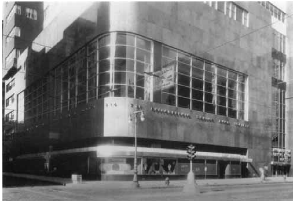
Figure 5.2 - Base of PSFS Building showing expansive glass window at second floor Banking Level. Source: George Howe, et al., "The PSFS Building, Philadelphia, Pennsylvania, 1929-1932." Perspecta . 25 (1989): 93.
