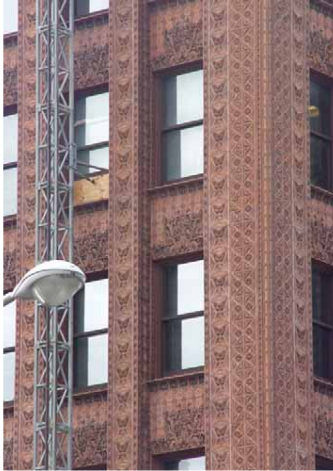
Figure 4.3 - Detail of the Guaranty Building facade, photo by B. Dandona 6 Nov. 2006.
