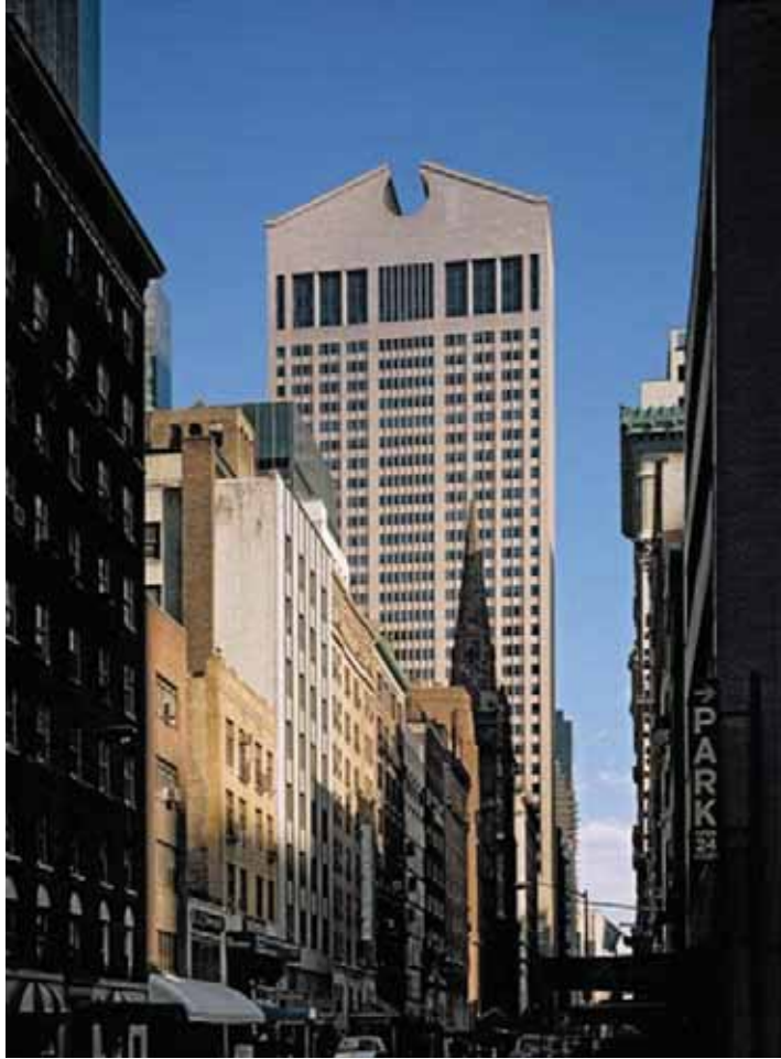
Figure 7.3 - AT&T Building. Source: < www.archpaper.com/.../03_05_philip_johnson.html >.
