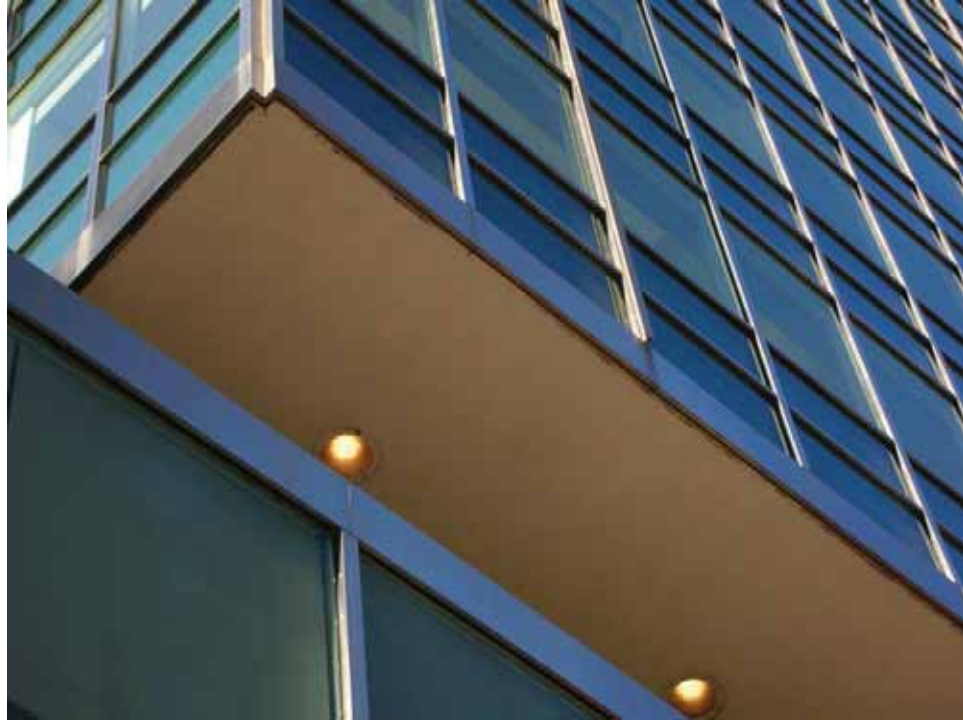
Figure 6.3 - Lever House curtain wall after replacement, photo by E. Buckley 19 Dec. 2006.
