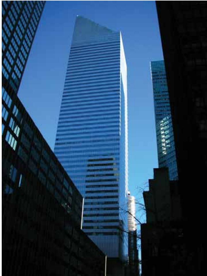
Figure 7.1 - Citicorp Center, photo by E. Buckley 19 Dec. 2006.
