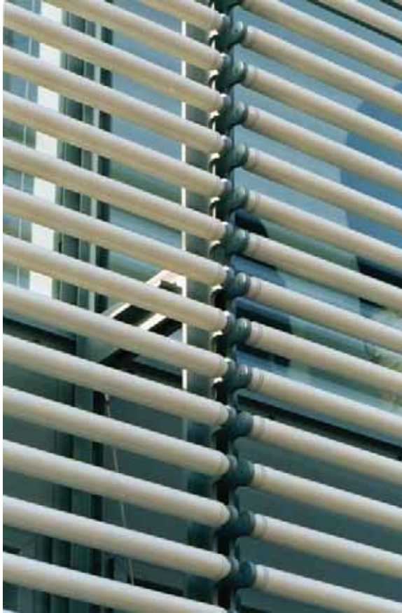
Figure 8.3 - Mock-up of ceramic tube skin on New York Times Tower. Source: Fx Fowle Architects.
