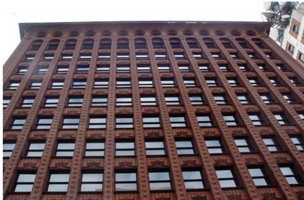
Figure 4.4 - Shaft of the Guaranty Building, photo by B. Dandona 6 Nov. 2006.
