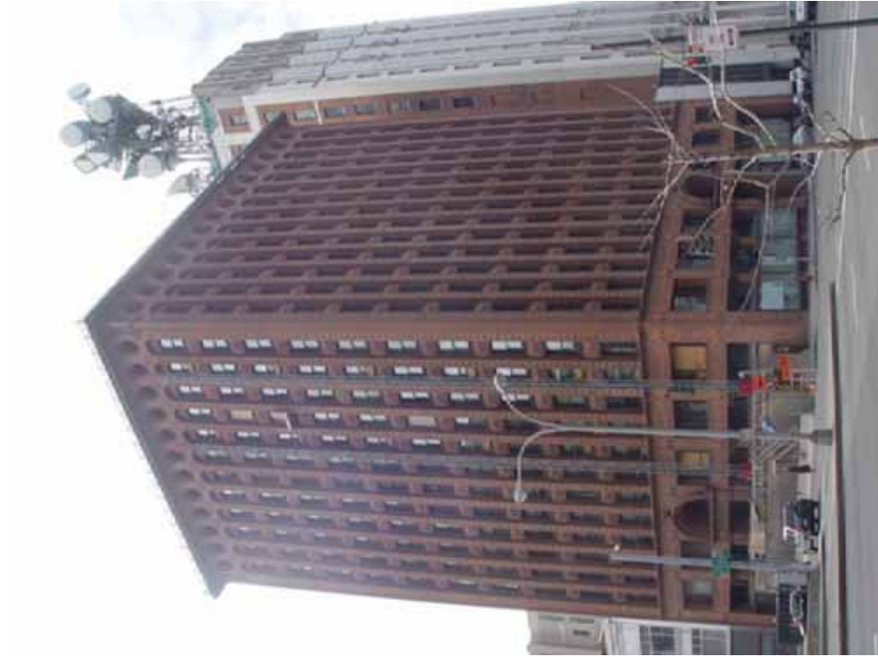
Figure 4.1 - The Guaranty Building, photo by B. Dandona 6 Nov. 2006.
