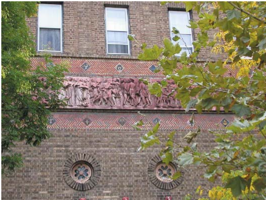
Fig. 6, Exterior, Frieze, decorative tile work, and circular windows
