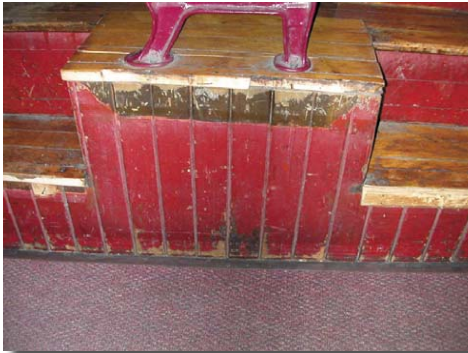
Fig. 29, Above , Chipping Red Paint on Seating Platforms Fig. 30, Below , Moulding Missing from Seating Platform
