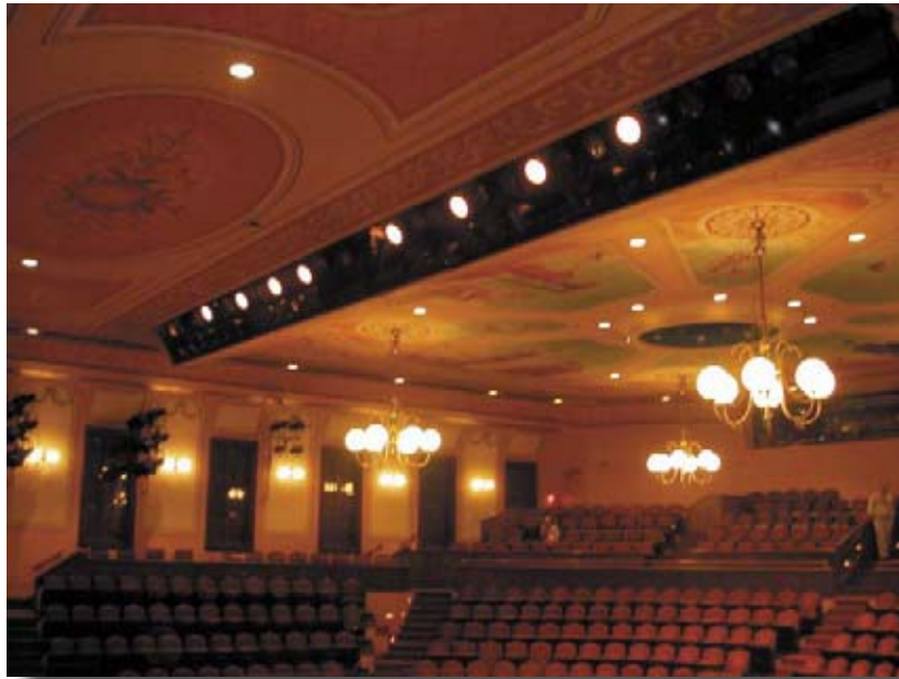
Fig. 58, Above , and Fig. 59, Below , Lighting Cove in Grand Opera House, Wilmington, DE
