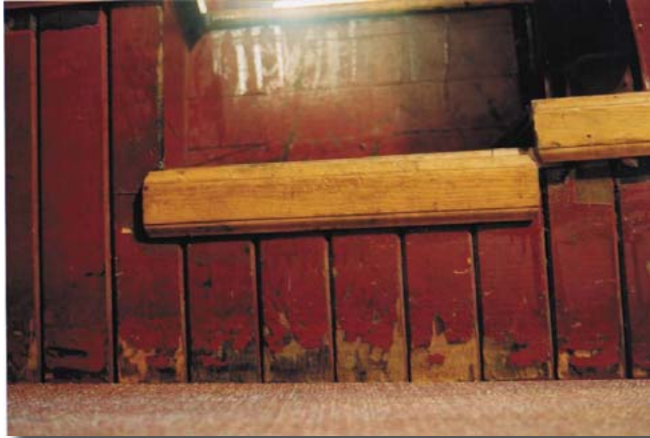
Fig. 29, Above , Chipping Red Paint on Seating Platforms Fig. 30, Below , Moulding Missing from Seating Platform
