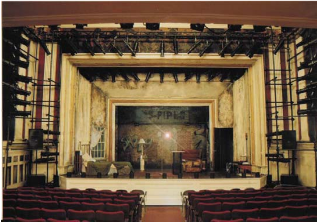
Fig. 53, Steels Pipes Installed for Lighting Instruments
