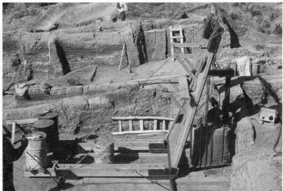
Figure 6.8. Rig assembly on site (South area) during experimental wall lifting operation. (Photo: L. Falck.)
