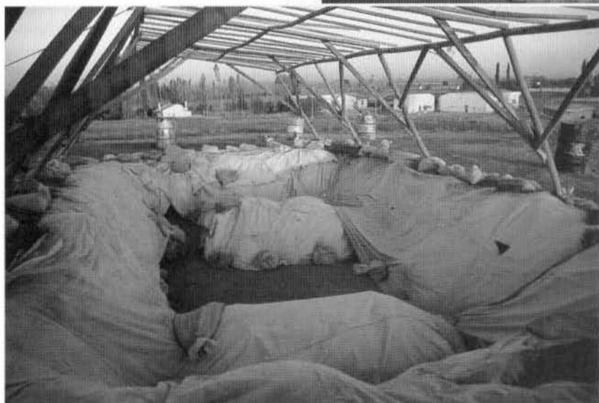
Figures 6.11–6.13. North area - Building 5. Sequential phases of reburial for temporary site protection during the winter months between field seasons. (Photos: E. Kopelson.)
