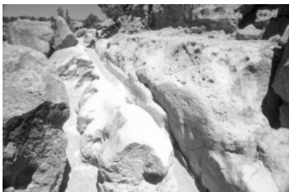
Figure 3. Typical trail degradation characterized by increased depth, collapsed walls from root-induced cracking and parallel secondary trail formation with surface abrasion.
