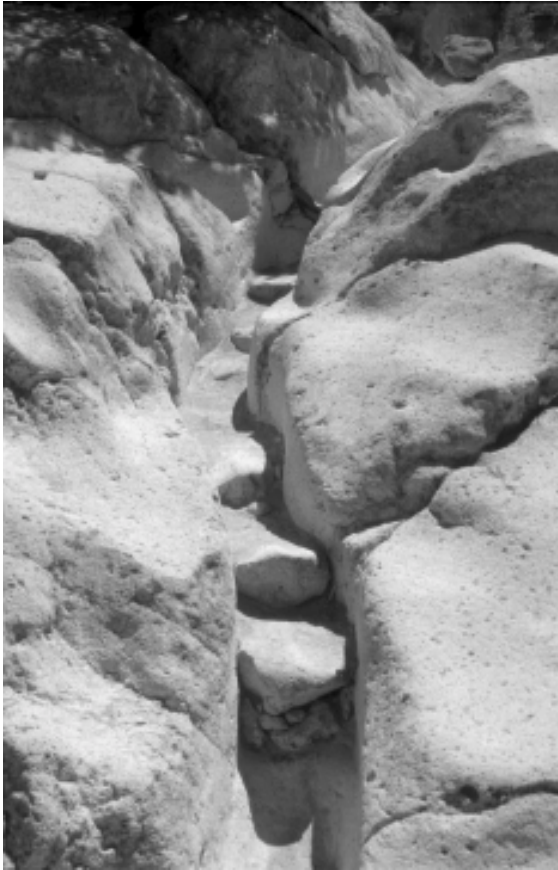
Figure 14. Deeply eroded trail, after stabilization with compacted gravel and added rock retaining steps.
