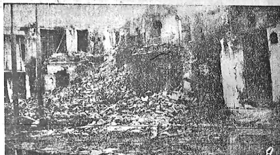
Ruined houses on Halsey Road
