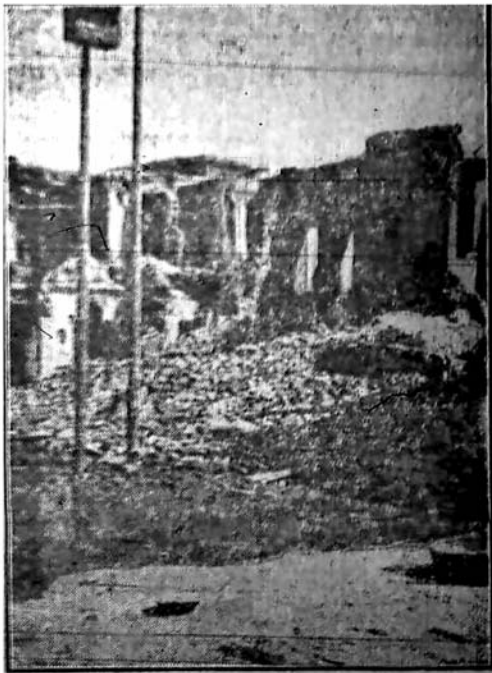
Houses on Halsey Road
