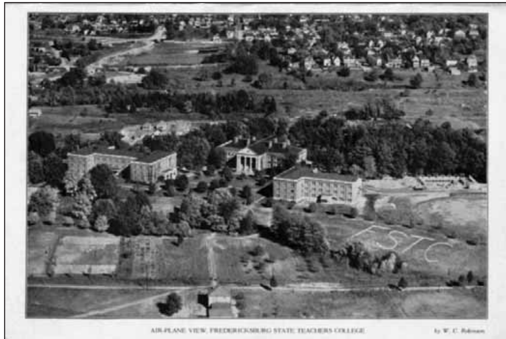
Figure 4: Aerial View, Fredericksburg State Teachers College, 1928.
