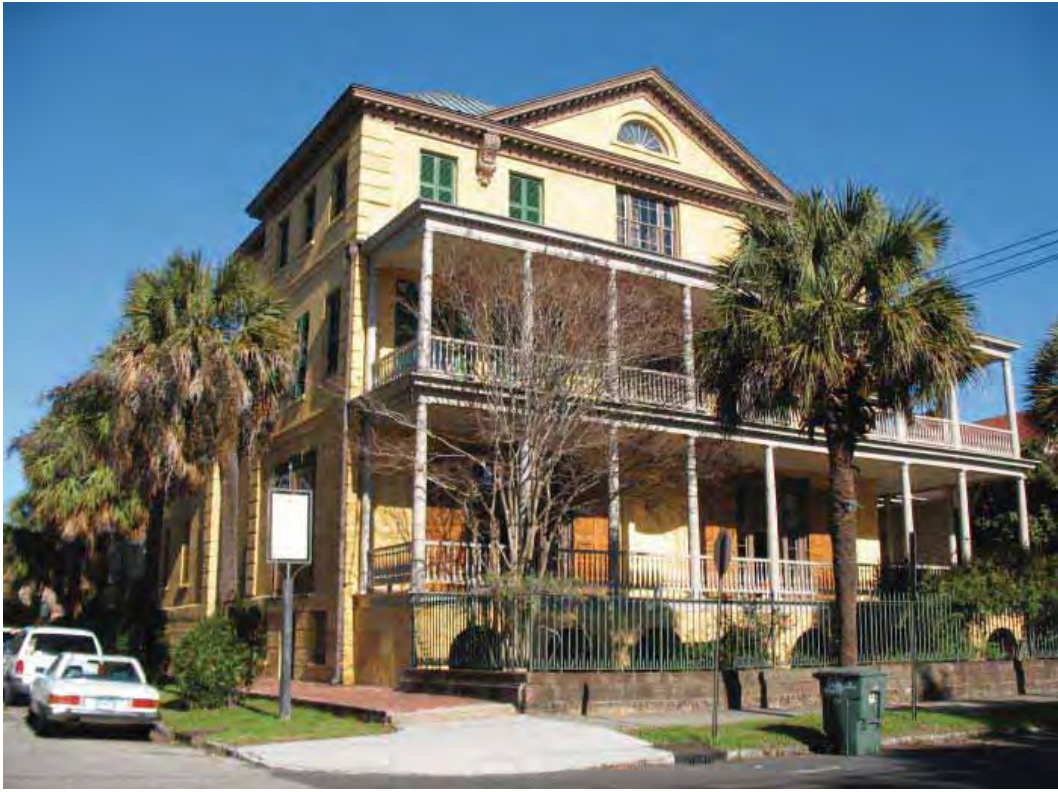
Figure 11: Southern Facade, Aiken-Rhett House, Jan. 2008 photo by author
