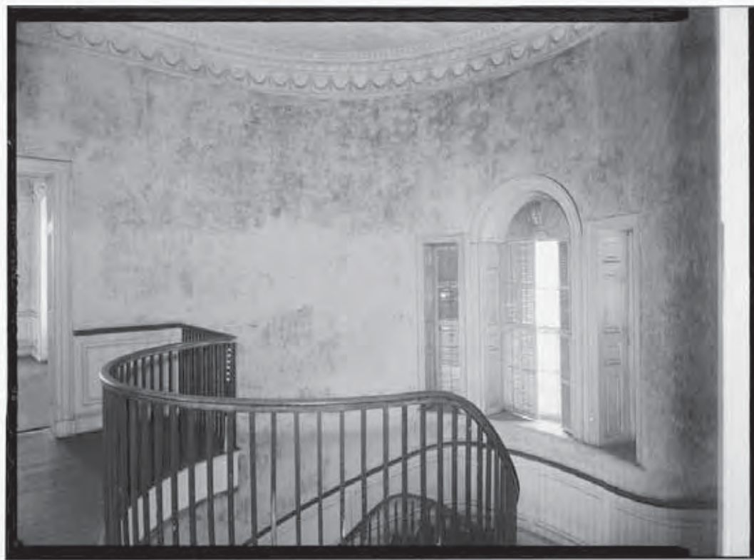
Figure 21: Second Story Stair Hall, Joseph Manigault House, HABS SC, 10-CHAR, 21-5 67-6 (1977-78) This window is said to have been used by the Manigault family to improve ventilation in the house
