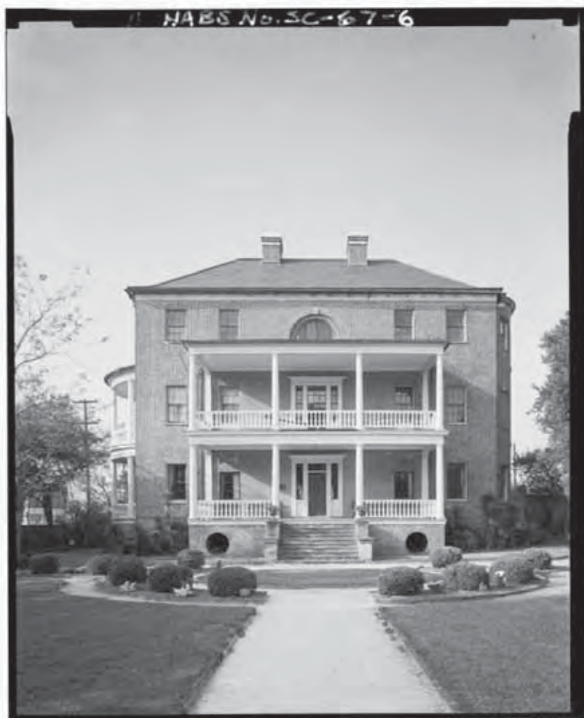
Figure 18: South Facade, Joseph Manigault House, HABS SC 67-6 (1977-78)
