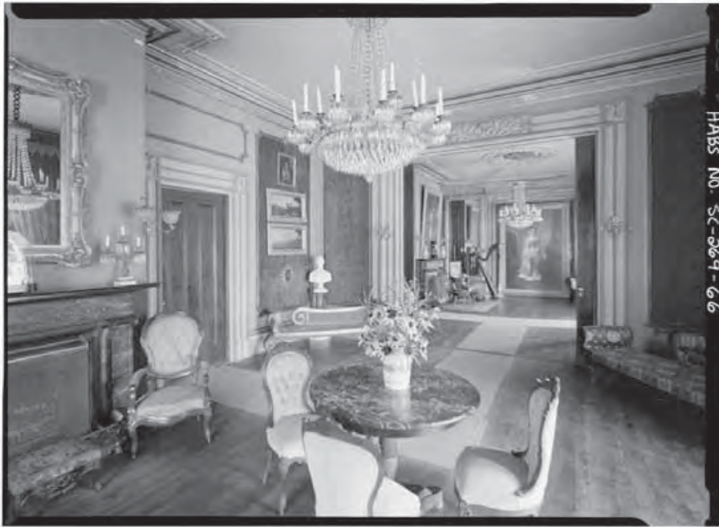
Figure 12: Double Parlor, Aiken-Rhett House, HABS SC 10-CHAR 177-66
