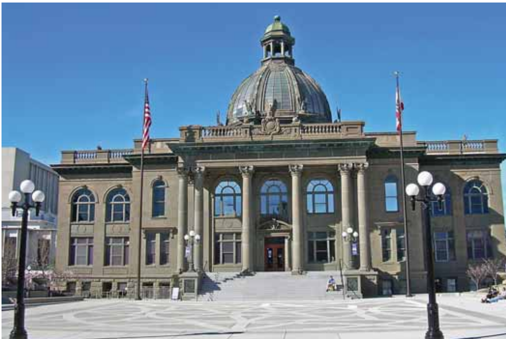
FIGURE 37. The fourth and final San Mateo County Courthouse was completed in 1910. The dome and rotunda of the current building were salvaged from the 1906 Courthouse that suffered irreparable damage from the San Francisco earthquake that same year. Image by roarofthefour, http://www.flickr.com/photos/18702768@N04/1934983450
