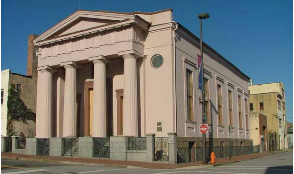
FIGURE 23. The 1845 Lloyd Street Synagogue in East Baltimore was Maryland's first synagogue, and is the third oldest remaining in the United States. Image by Alan Cordova, http://www.flickr.com/photos/acordova/2946090640
