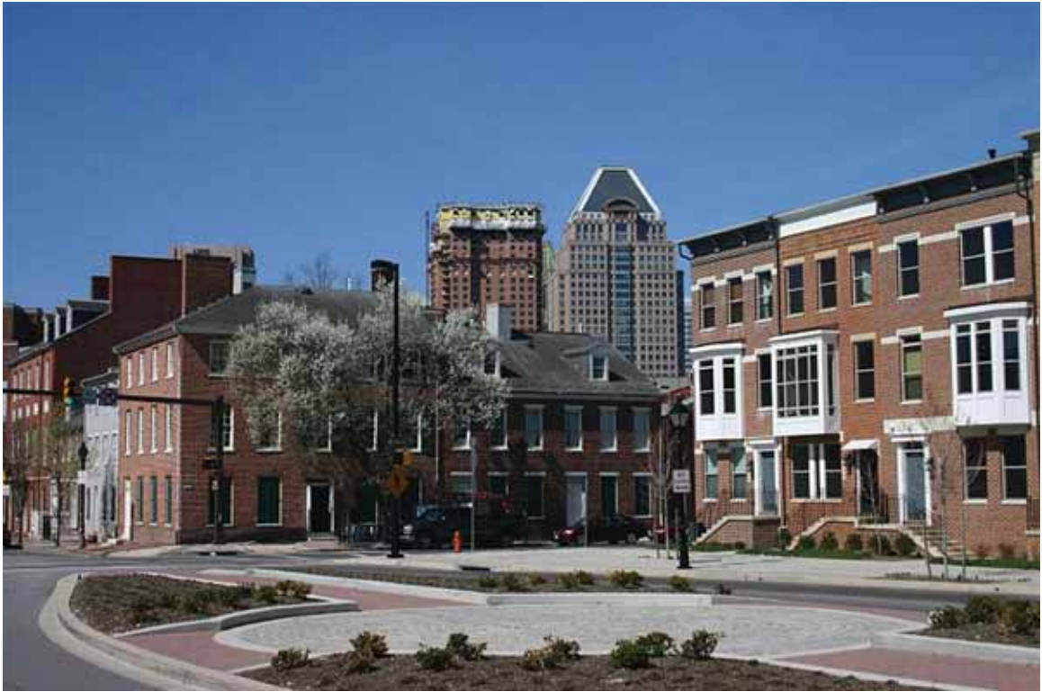
FIGURE 29. Albemarle Square was designed to merge seamlessly with the historic context of East Baltimore. New residential buildings to the right respect the scale and massing of historic structures located on the left. Image by R2 Productions, LLC, http://baltimore.shownbyphotos.com/20070402-federal-hill-0141-800.jpg-large.html
