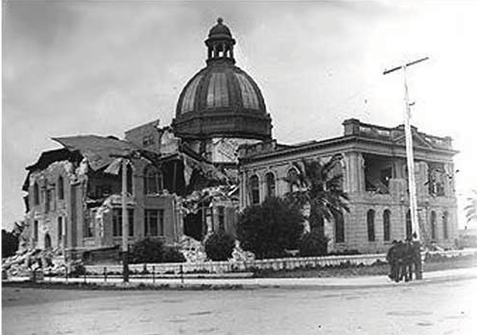
FIGURE 36. The San Francisco earthquake of 1906 decimated the third San Mateo County Courthouse. The dome and rotunda were salvaged for the fourth and final courthouse that now stands on the site. Image by City of Redwood City (all rights reserved), http://www.redwoodcity.org/cds/redevelopment/downtown/history/courthouse3.html
