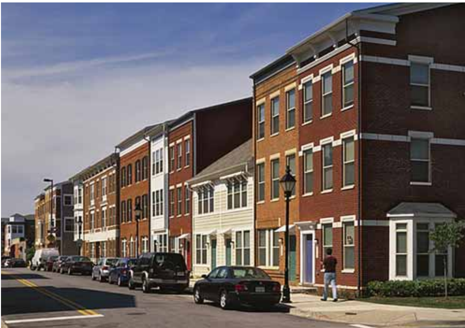
FIGURE 33. The new buildings at Albemarle Square were designed to harmonize with indigenous residential building stock. Image by Torti Gallas and Partners (all rights reserved), http://www.tortigallaschk.com/image_pop.asp?i=images/THUMBS/81286/resource/screen_188730.jpg
