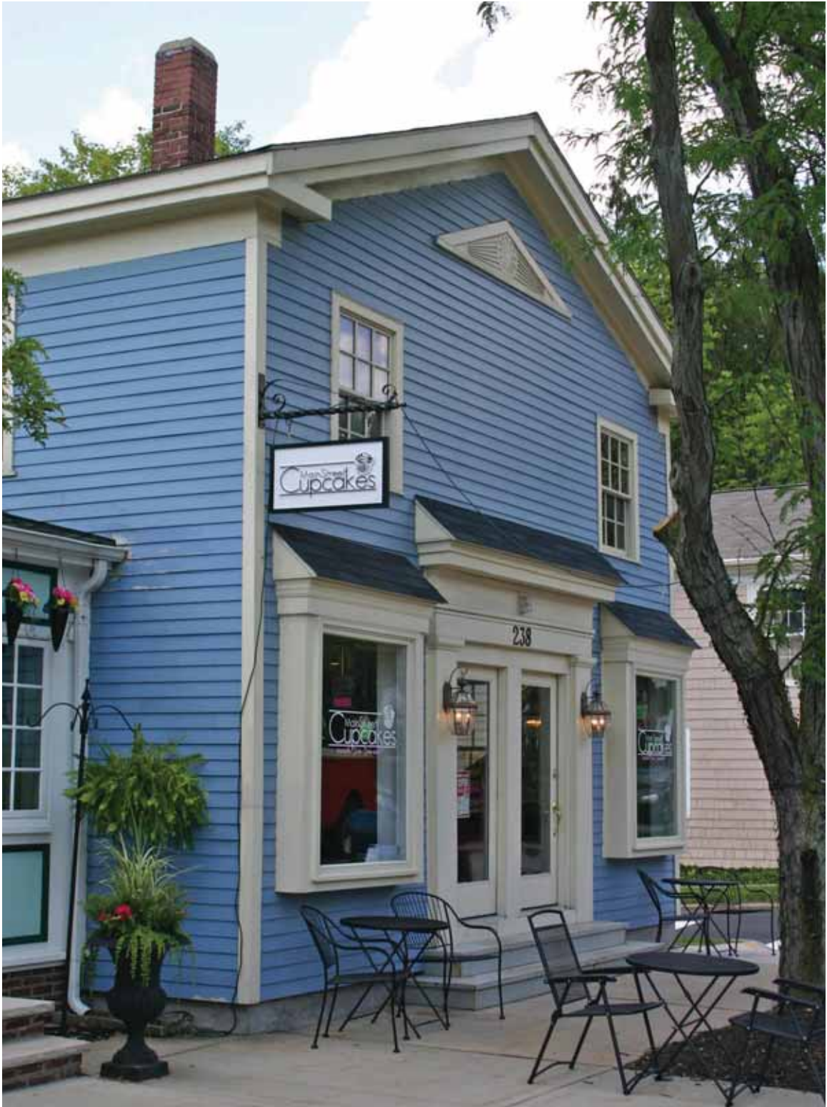
FIGURE 17. Hudson's historic North Main Street is predominated by modest two-story wood frame structures featuring front-end gables. Image by Merchants of Hudson (all rights reserved), http://www.flickr.com/photos/merchantsofhudson/2797423204
