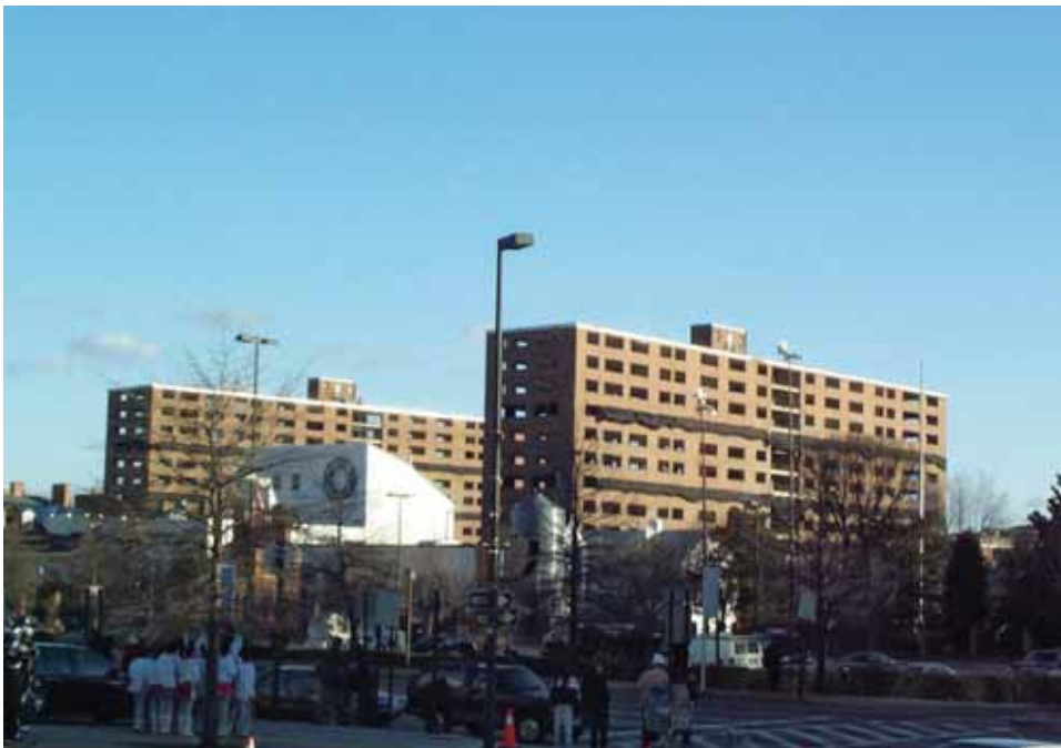
FIGURE 26. The Flag House Courts towers await demolition on the morning of February 10, 2001. Image by pagodabob (all rights reserved), http://www.flickr.com/photos/pagodabob/90457860
