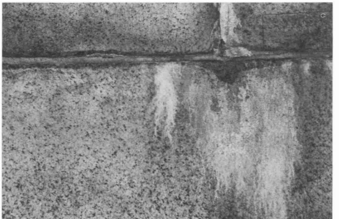
26. Area after 100-psi cleaning with walnut shells (C2) and sharp-edged sand (D2).
