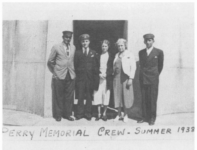
6. Base of Perry Memorial Column (1938).
