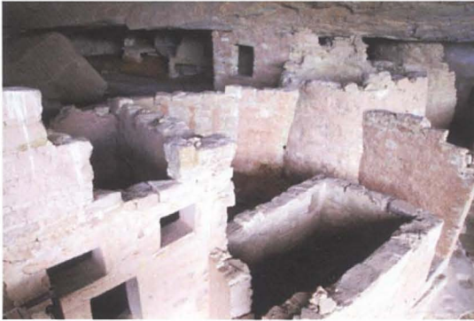
Fig. 2. Extant exterior and interior architectural surface finishes at Speaker Chief House, Cliff Palace, Mesa Verde. Courtesy Architectural Conservation Laboratory, University of Pennsylvania
