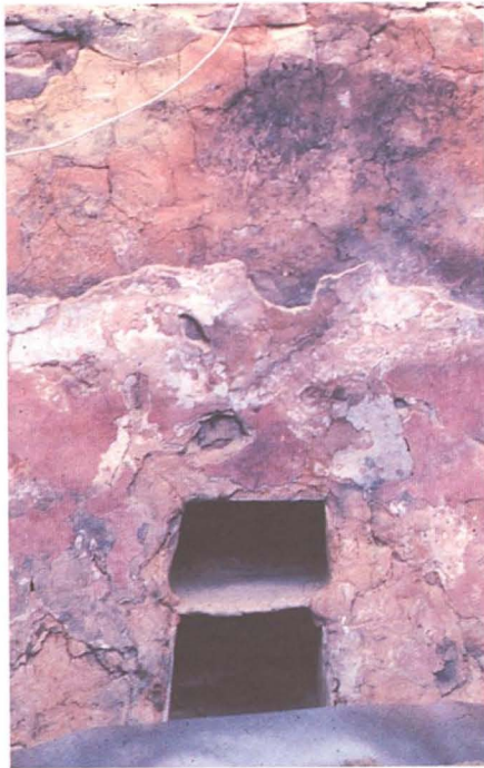
Fig. 11. Kiva C, Mug House, Sector 9—conditions. Arrows indicate areas of loss since excavation (1959–60) (a) and salts and flaking in lower wall (b). Sector 9 photo elevation and condition drawing. Courtesy Architectural Conservation Laboratory, University of Pennsylvania
