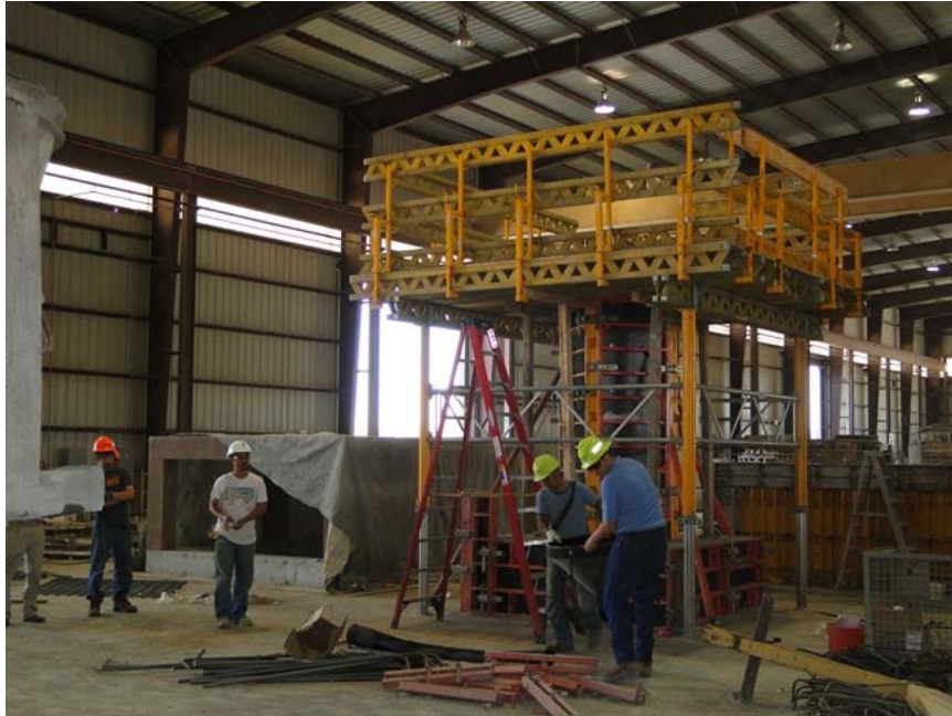
Figure A.6. Forming Column and Top Block
