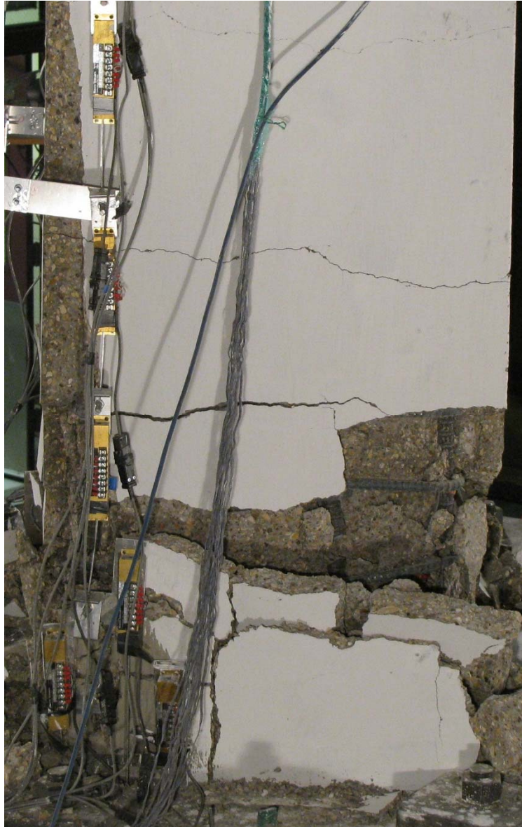
Figure 5.29. Observed Damage at the Beginning of “Failure” Damage Category
