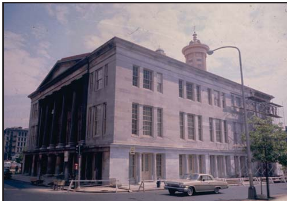
Figure C.42: South elevation Source: INHP Archives Date: May 17,1965, W.A. Creator: McCullough
