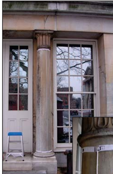
Figure 4.2: (right) Grid applied to column for recording Figure 4.3: (lower right) Grid placement detail Figure 4.4: (left) AutoCAD Base drawing used for recording
