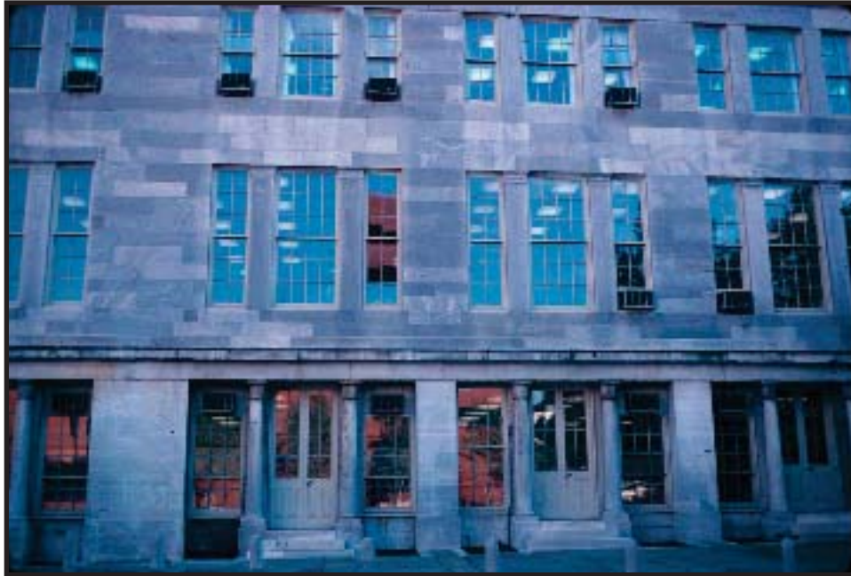
Figure C.3: North elevation April 1976 Source: INHP Archives
