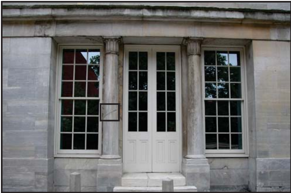
Figure C.24: North elevation, columns 1 and 2 Summer 2004 Source: University of Pennsylvania Note on column 1, a composite repair that runs diagonally across the the column that was not present in the historic photograph.
