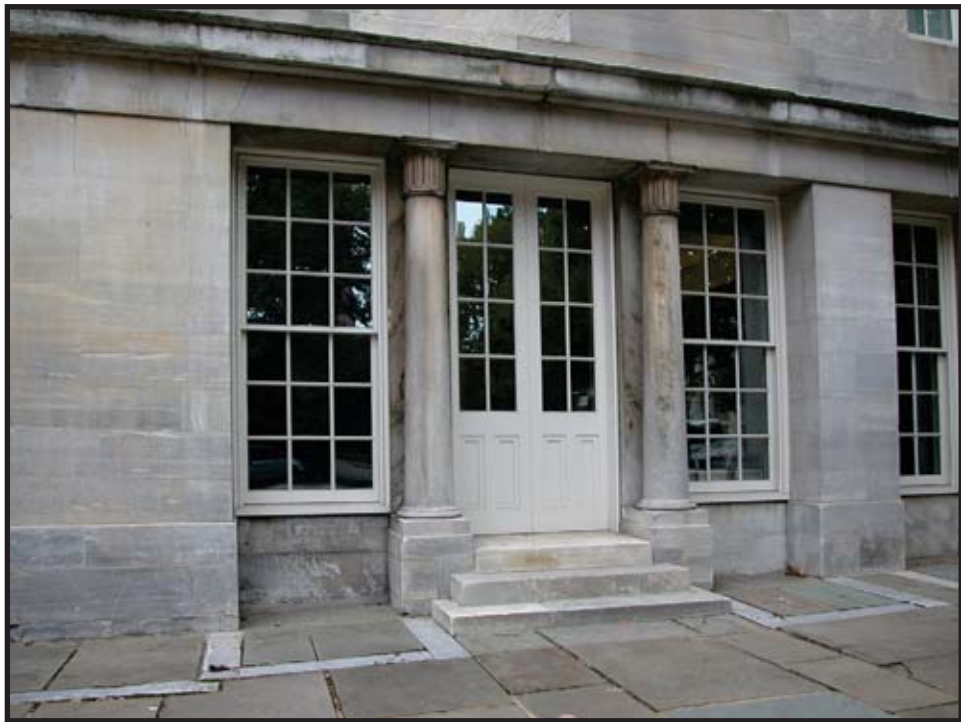
Figure C.22: North elevation, columns 3 and 4 Summer 2004 Source: University of Pennsylvania
