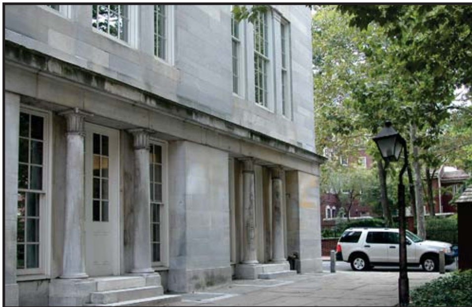
Figure C.28: North elevation, columns 6-10 Summer 2004 Source: University of Pennsylvania
