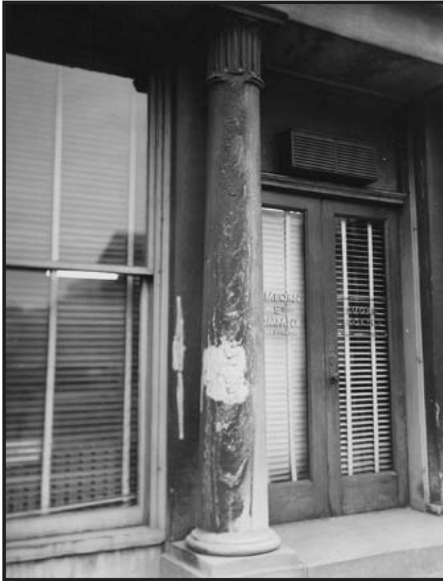
Figure C.19: North elevation, column 9 Source: INHP Archives, Historical Society of Philadelphia Caption: Merchants' Exchange: north elevation, note: deterioration of stonework on column Creator: PH Date: February 19, 1957
