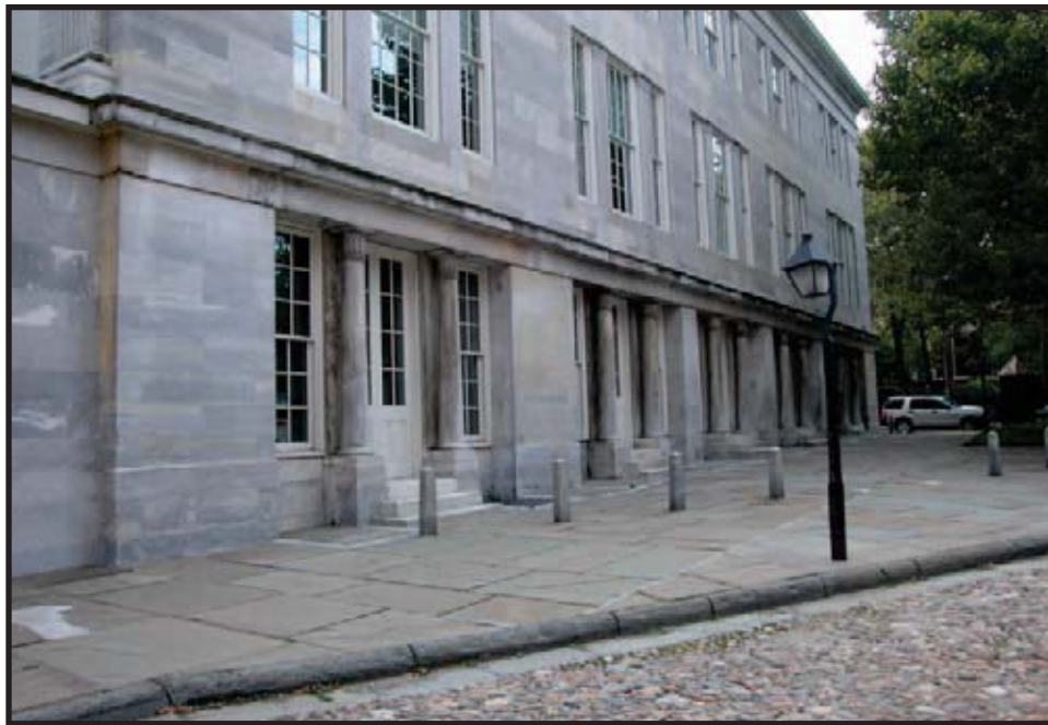
Figure C.30: North elevation, columns 1-10 Summer 2004 Source: University of Pennsylvania
