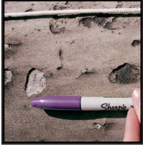
small blisters detaching from stone surface
