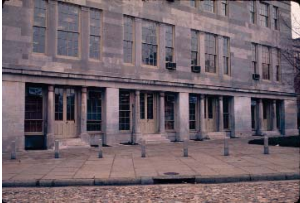
Figure C.7: North elevation, October 1975 Source: INHP Archives
