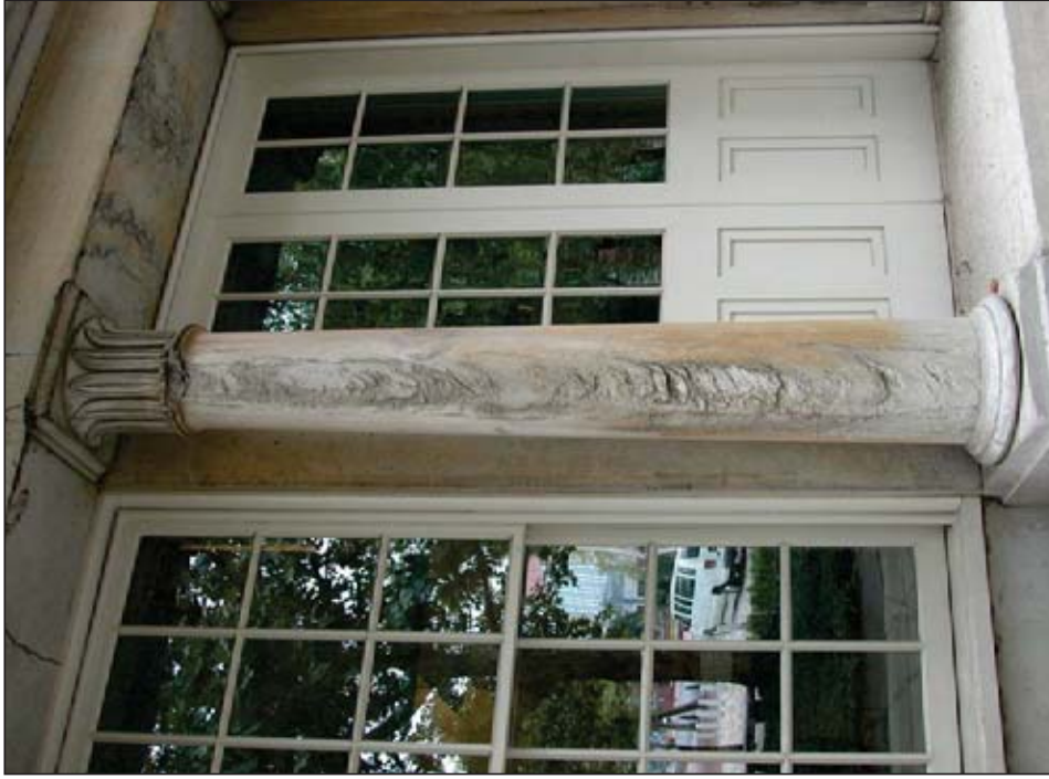
Figure 4.31: North Elevation, column 9 Source: University of Pennsylvania Date: Summer 2004
