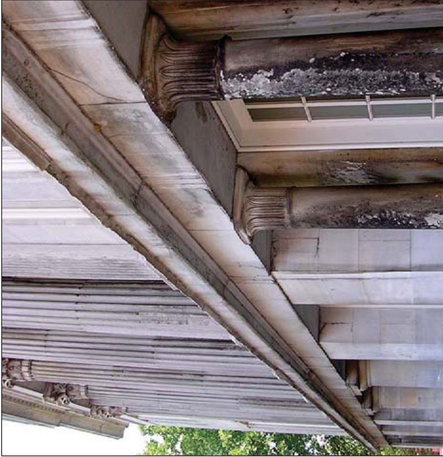
Figure 4.15: West Elevation, columns 3 and 4 Source: University of Pennsylvania Date: November 2004
