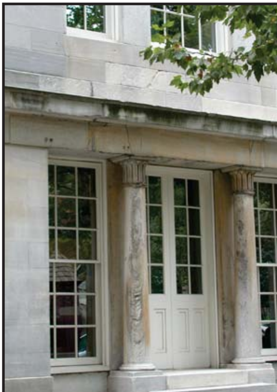
Figure C.10: North elevation, Summer 2004 Columns 9 and 10 Source: University of Pennsylvan- ia
