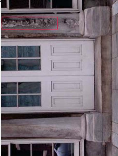
Figure 4.20: South Elevation, columns 7 and 8 Source: University of Pennsylvania Date: Summer 2004
