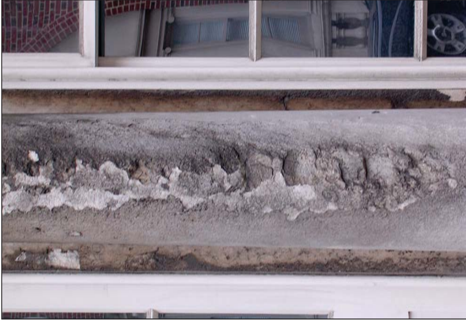
Figure 4.22: South Elevation, detail of column 8 Source: University of Pennsylvania Date: Summer 2004
