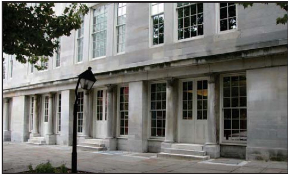
Figure C.18: North elevation, columns 6-10 Summer 2004 Source: University of Pennsylvania
