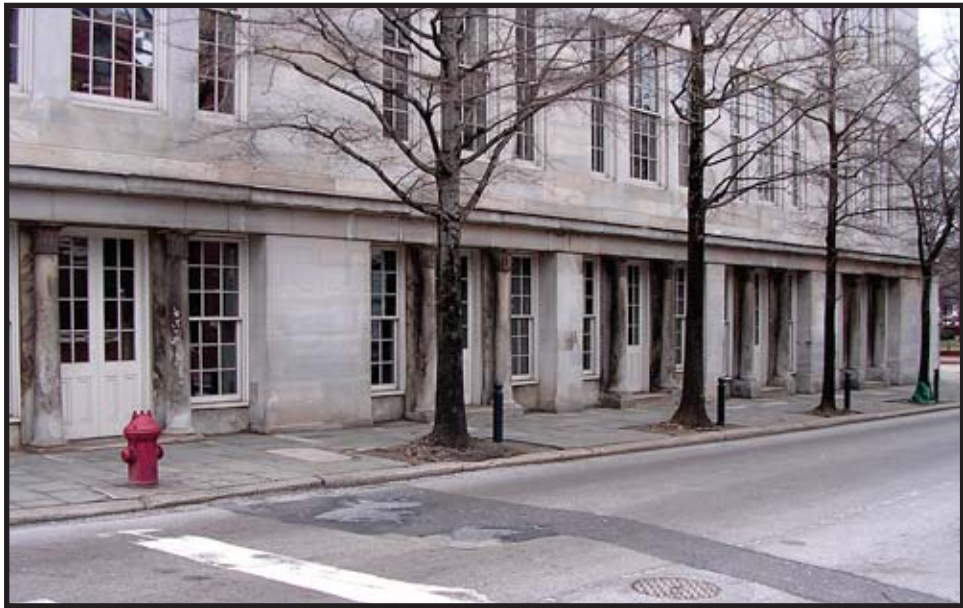
Figure C.49: South elevation, columns 1-10 Winter 2005 Source: University of Pennsylvania
