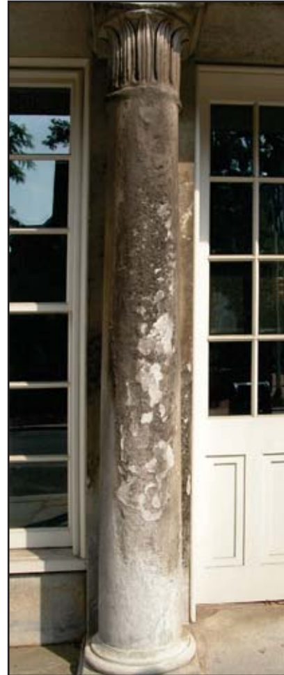
Figure 1.2: West Elevation, column 3, summer 2004
