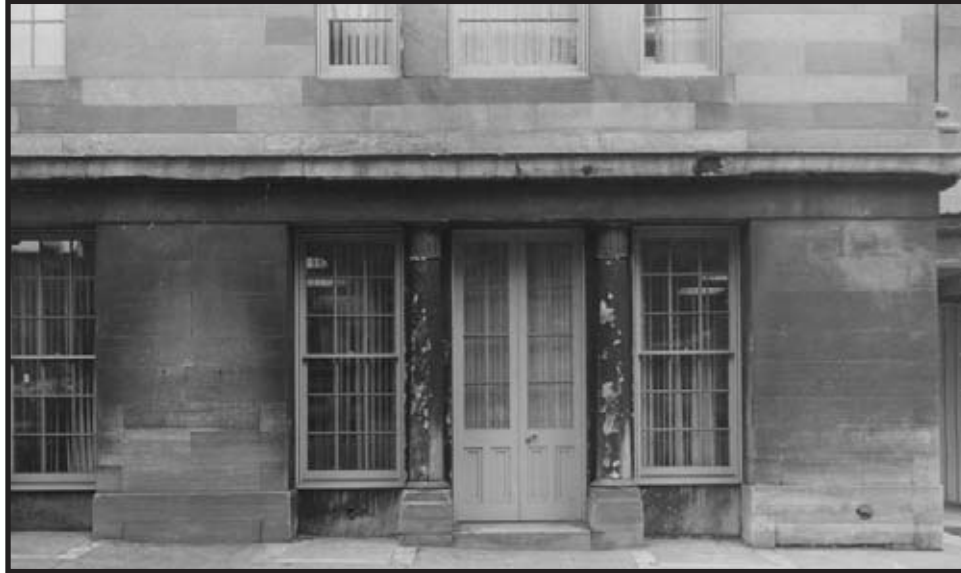
Figure C.37: South elevation, columns 9 and 10 Source: INHP Archives Caption: Merchants' Exchange marble deterioration detail Creator: W. A. McCullough Date: April 5, 1961
