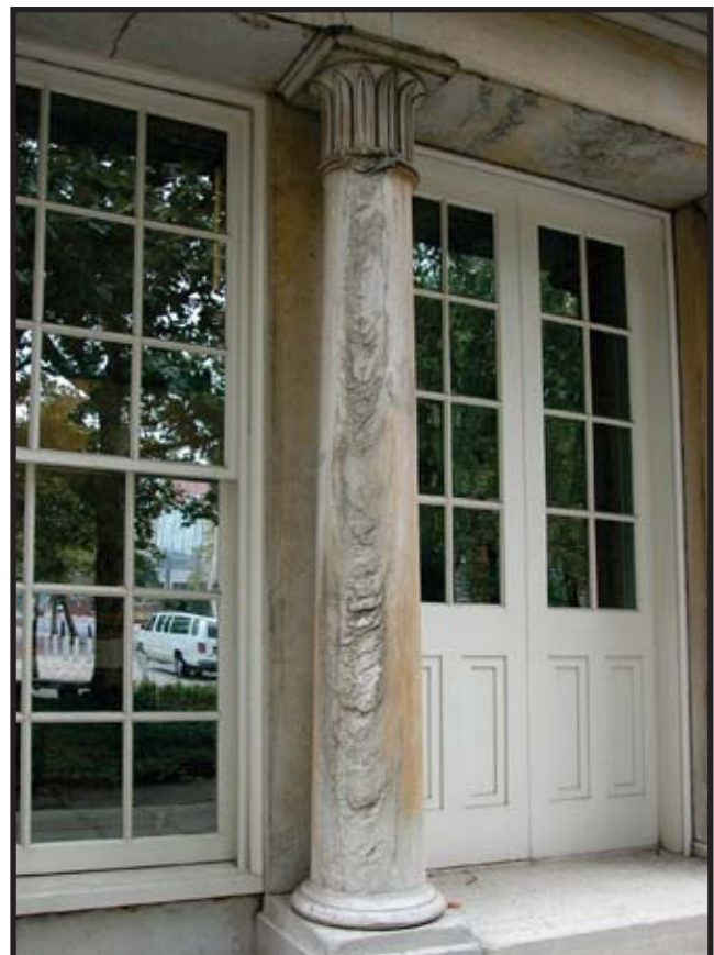
Figure C.19: North elevation, column 9 Source: INHP Archives, Historical Society of Philadelphia Caption: Merchants' Exchange: north elevation, note: deterioration of stonework on column Creator: PH Date: February 19, 1957
