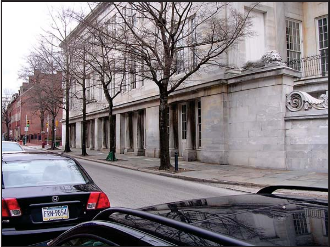
Figure C.54: South elevation, columns 1-10 Source: University of Pennsylvania Date: Winter 2005
