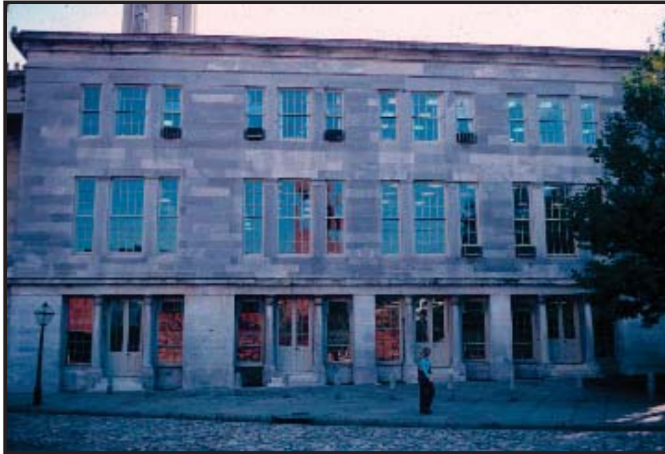
Figure C.11: North elevation, October 1975? Source: INHP Archives
