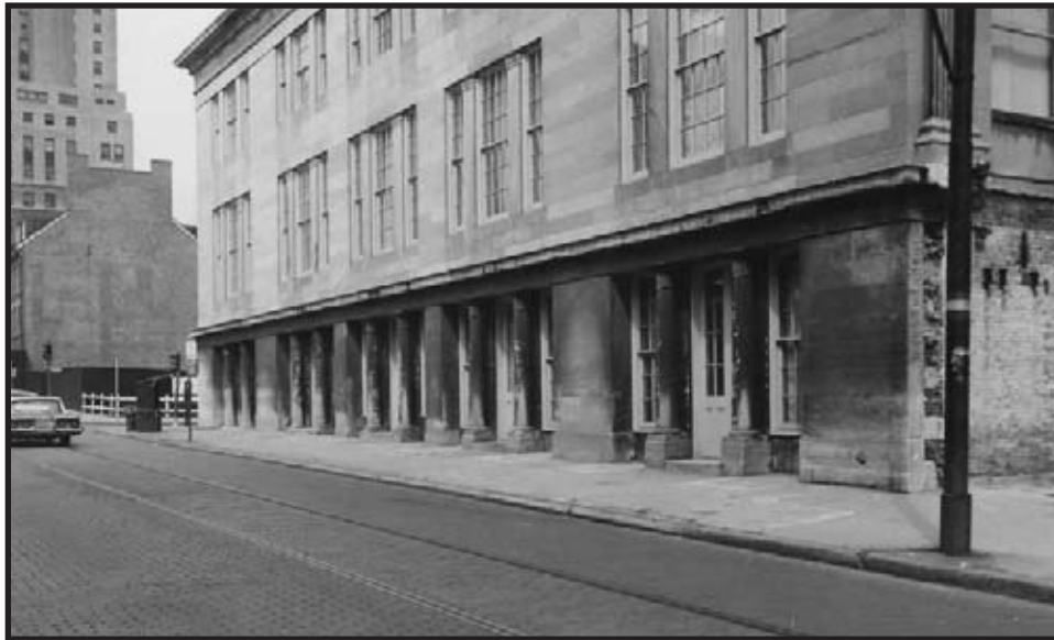
Figure C.53: South elevation, columns 1-10 Source: INHP Archives Creator: W. A. McCullough Date: April 5, 1961
