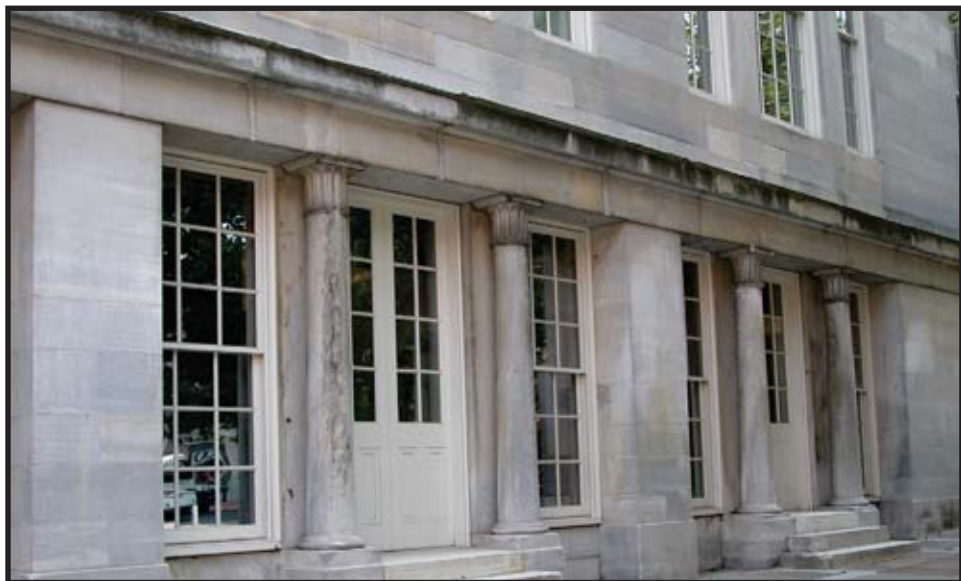
Figure C.26: North elevation, columns 5-8 Summer 2004 Source: University of Pennsylvania
