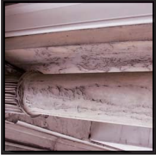
(b) blistering along mineral inclusions
