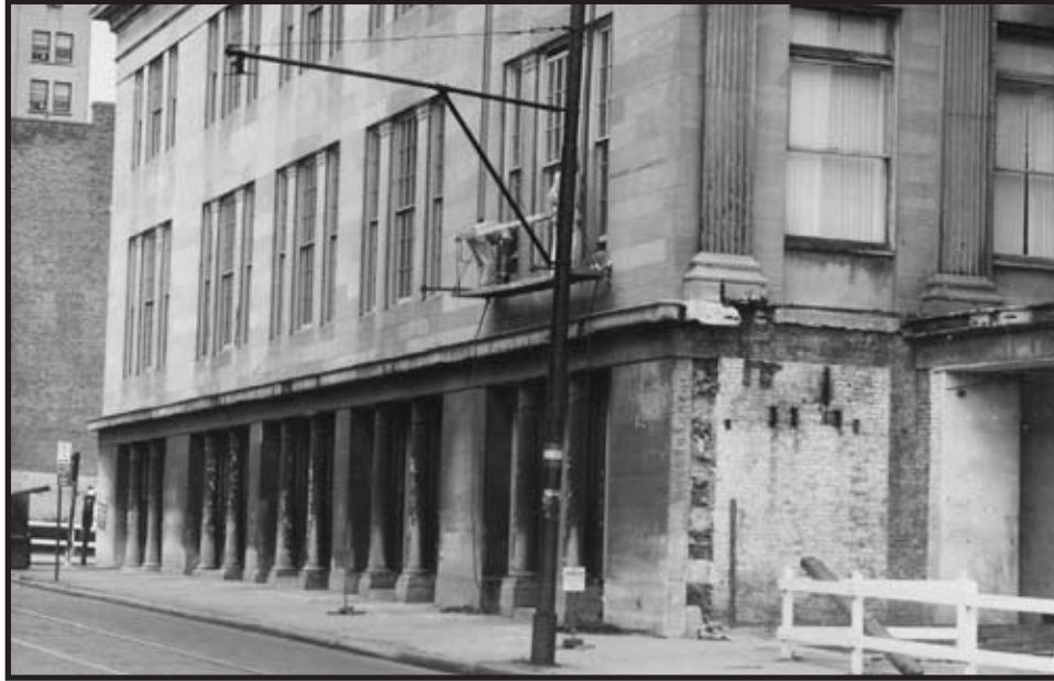
Figure C.52: South elevation, columns 1-10 Source: INHP Archives Caption: Merchants' Exchange Creator: W. A. McCullough Date: March 16, 1961
