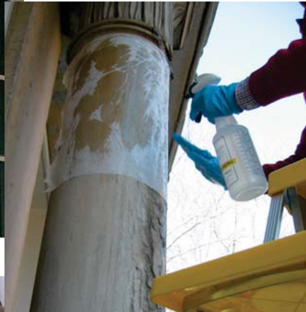
Figure 5.3: (bottom left) North elevation, column 9, Application of barium hydroxide poultice
