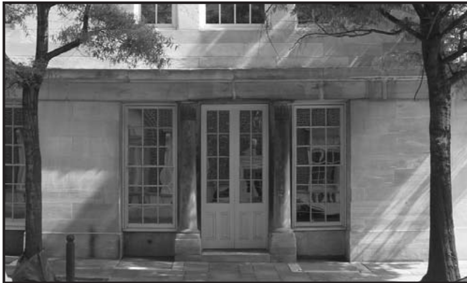
Figure C.38: South elevation, columns 9 and 10 Summer 2004 Source: University of Pennsylvania
