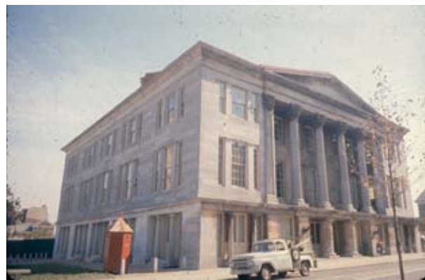
Figure 2.8: Merchants’ Exchange, after restoration, northwest façade, July 18, 1966. From the INHP Archives.
