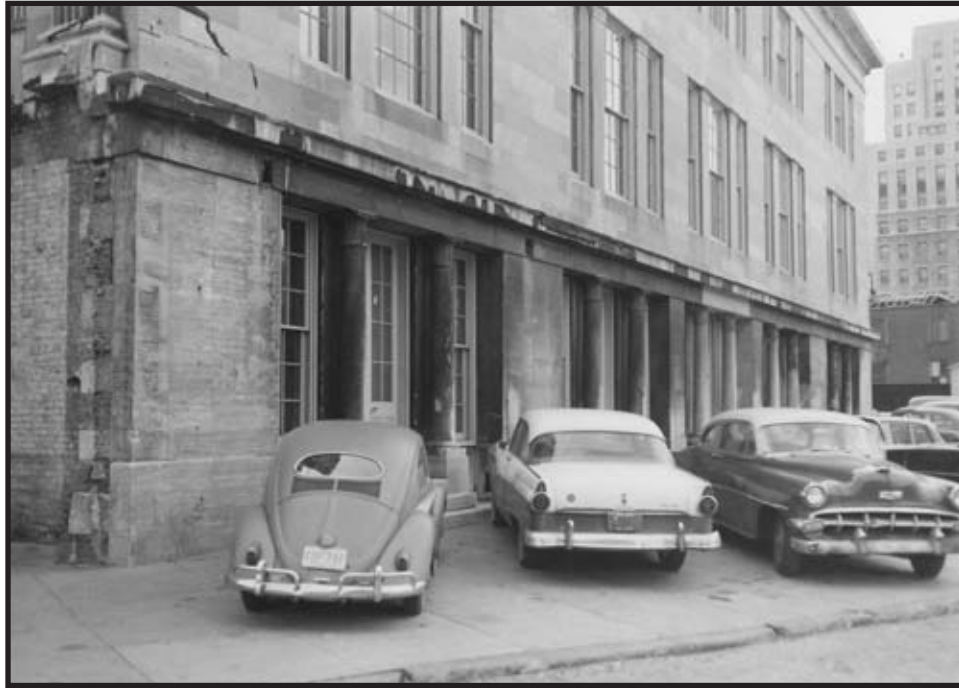
Figure C.29: North elevation, columns 1-10 Source: INHP Archives Creator: W. A. McCullough Date: April 5, 1961
