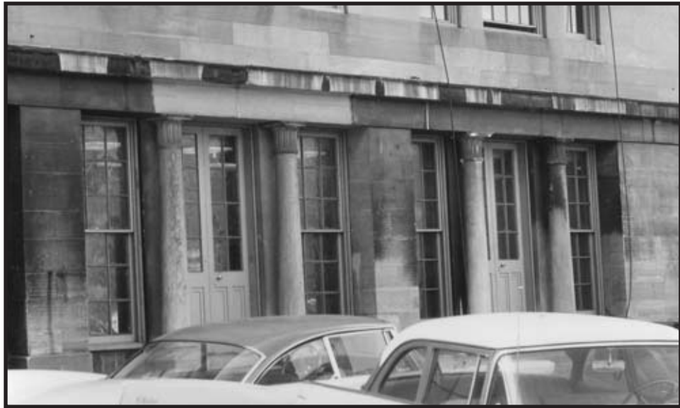
Figure C.25: North elevation, columns 5-8 Source: INHP Archives Caption: Merchants' Exchange – first level, second and third bays from west Creator: W. A. McCullough Date: March 16, 1961
