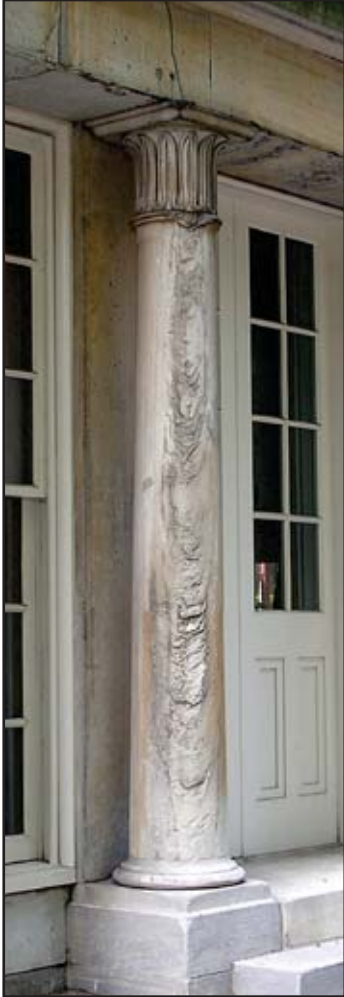
Figure 1.3: North Elevation, columns 7 and 8, summer 2004
