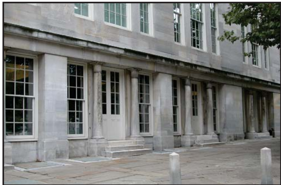
Figure C.16: North elevation, columns 5-10 Summer 2004 Source: University of Pennsylvania
