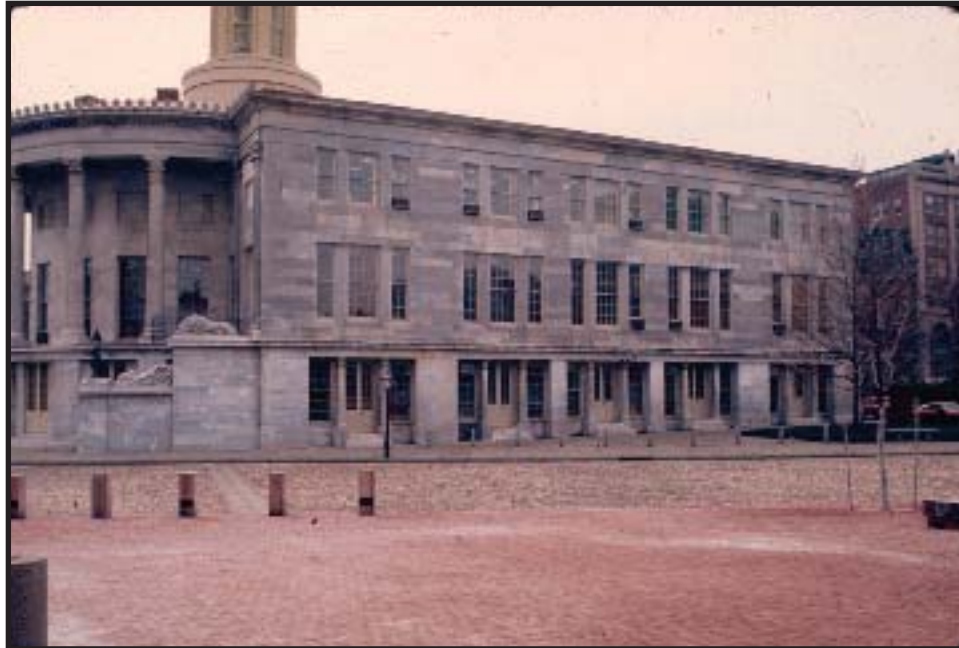
Figure C.5: North elevation, April 1976 Source: INHP Archives
