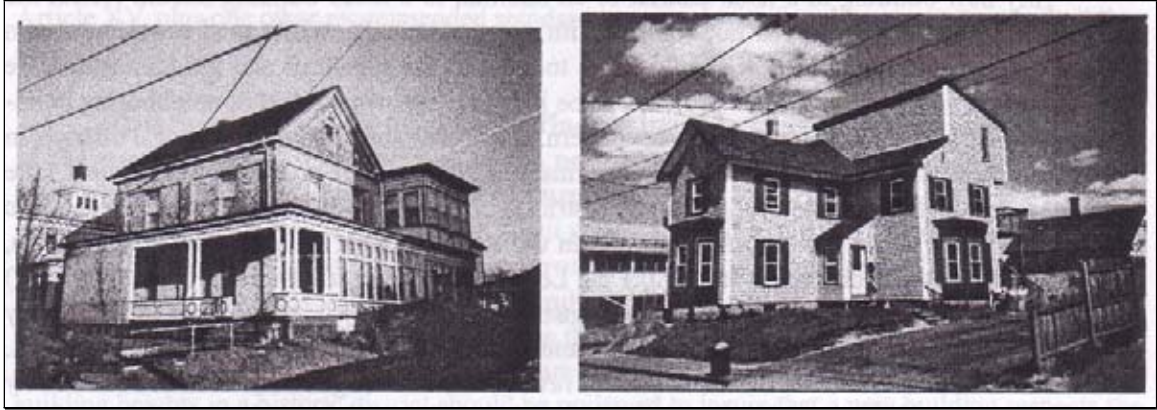
Figure 3 – Photographs from The Lewiston Historic Preservation Design Manual illustrating reversibility. The house shown at left could easily remove later additions while the house on the right would not be easy to correct according to the guidelines. 33
