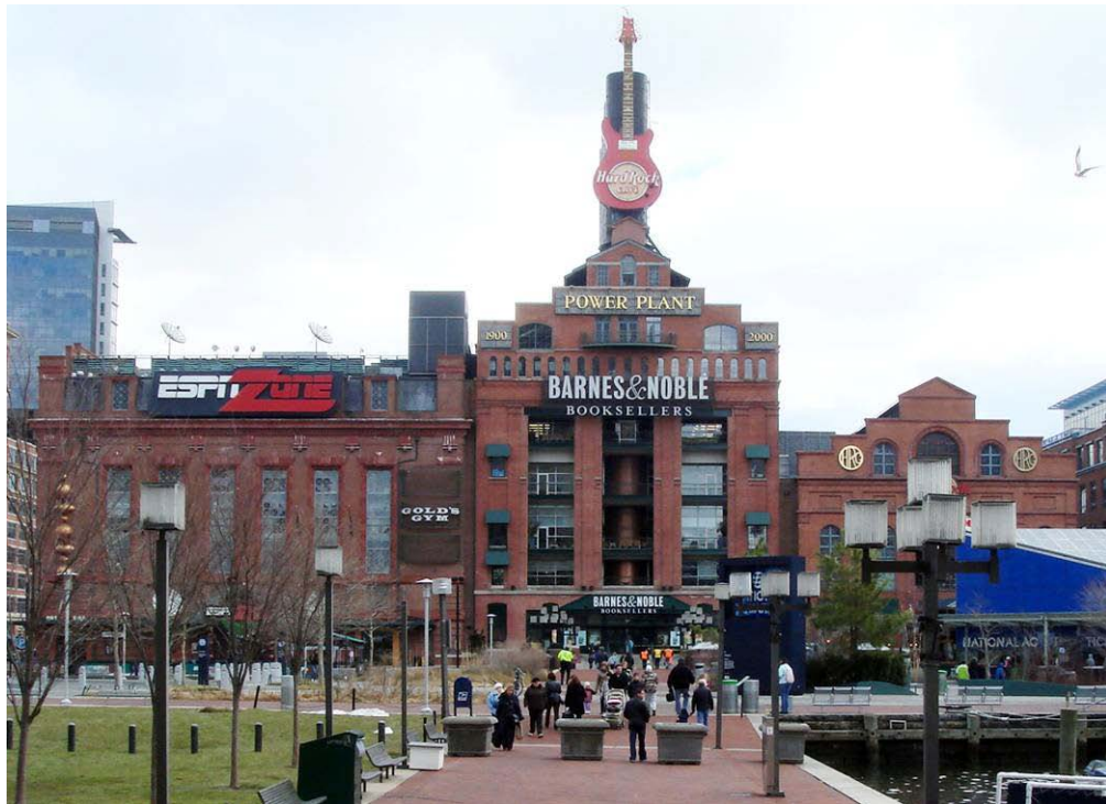
Figure 34 Restored Pier 4 Power Plant. Photo: J. Spector (2010)
