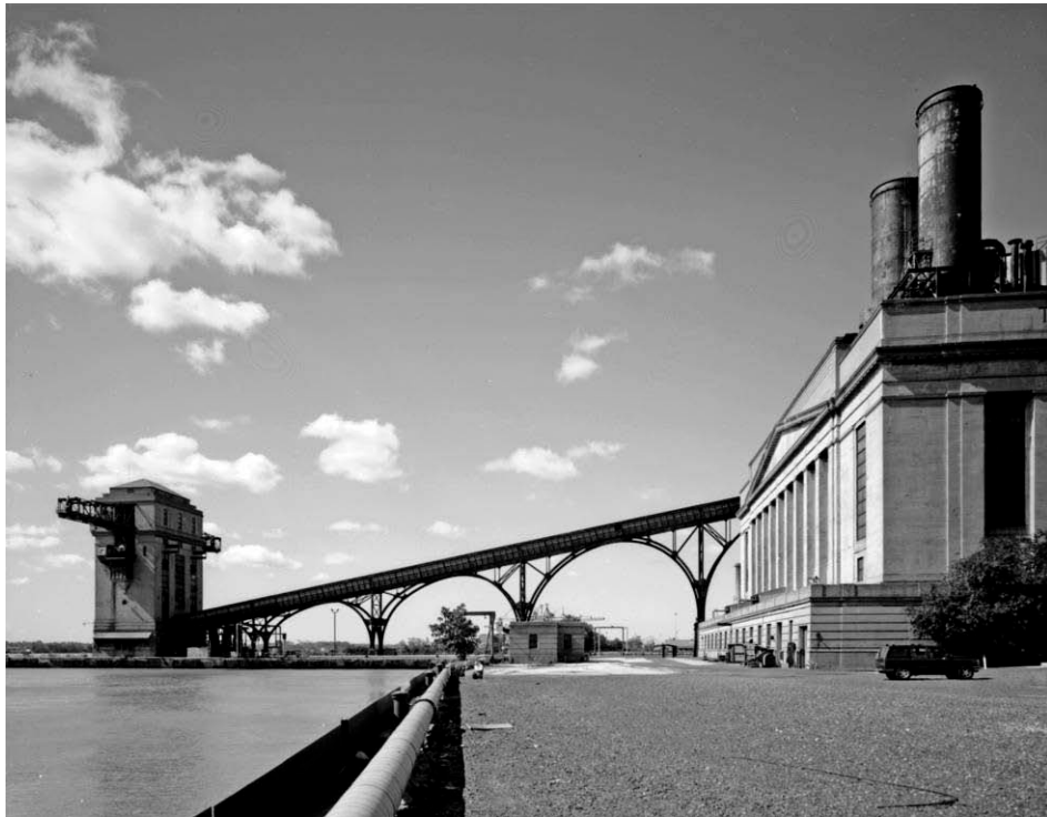
Figure 53 Richmond Power Generating Station. Photo, J.E.B. Elliot (c.2000)
