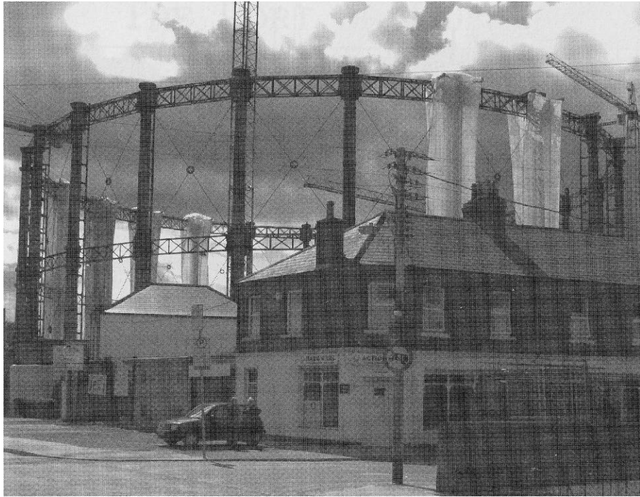
Figure 59 Clayton Gasometer. Photo, Dublin Docklands Reinvented by Niamh Moore.
