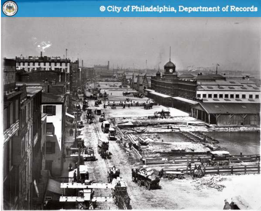
Figure 45 Delaware Avenue widening. Photo: Philadelphia Department of Records (1899)
