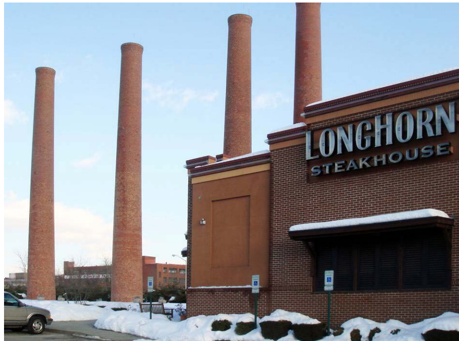
Figure 27 New smokestacks at Homestead Works. Photo: J. Spector (2010)
