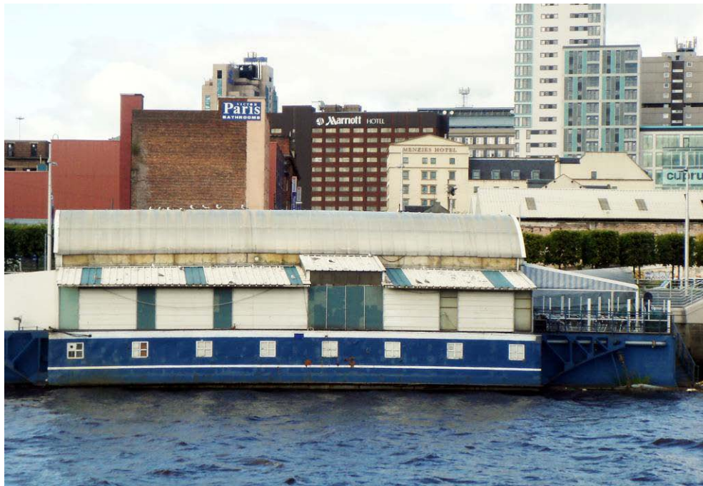
Figure 75 Riverfront warehouse with additions, Glasgow. Photo: J. Spector (2009)
