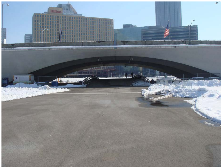
Figure 21 Concrete arch highway overpass at Point State Park. Photo: J. Spector (2010)
