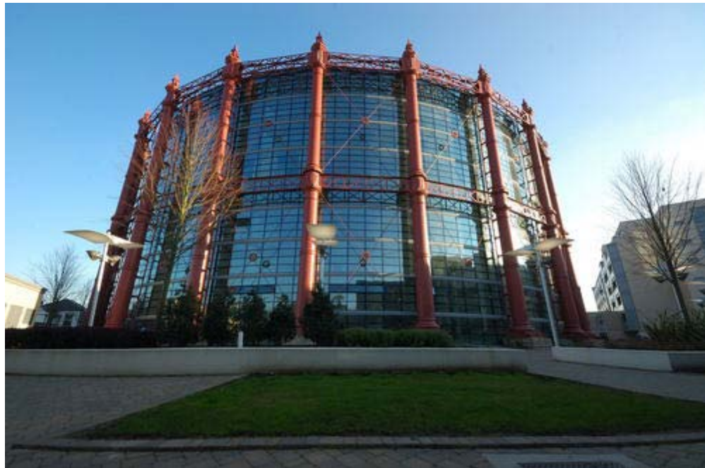
Figure 66 Alliance Building in gasometer framework, Dublin. Photo: Charles Howarth. (2007)
