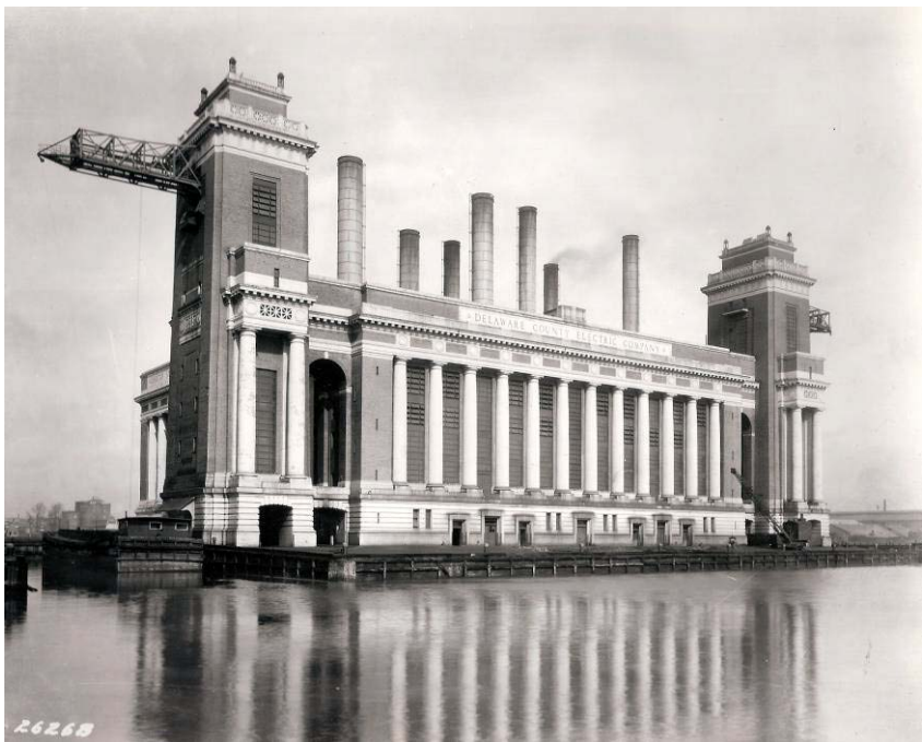
Figure 48 Chester Station electric plant. Chester, Pennsylvania (c. 1930)
