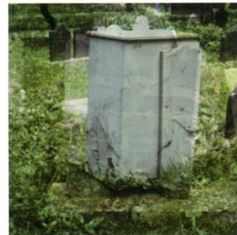
Fig. 5. Emergency stabilization using a closed, ventilated box around the structure. Photograph by Frank Matero.
