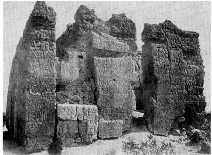
Figure 3. South elevation of the Casa Grande, c. 1888, published by Fewkes (1892). Note partial wall segment that collapsed by 1891–2.
