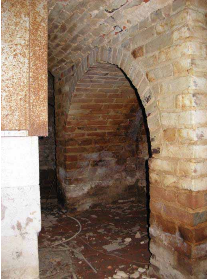
Figure 39. Photograph of the west room arched brick chimney support on the west wall of the 1859 block of the Abel and Mary Nicholson house. (Source: A. Aiken; taken 2/23/2007.)
