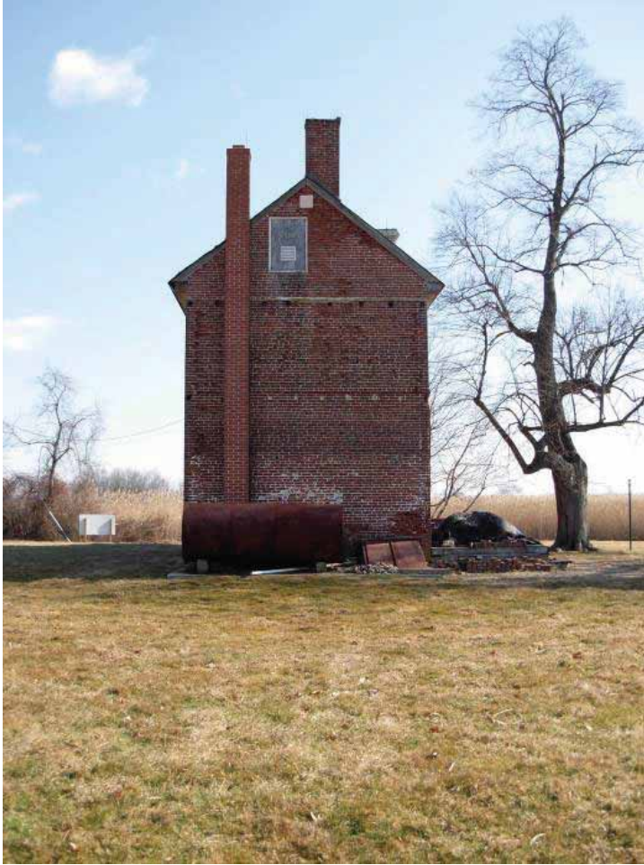
Figure 25. Photograph of the west façade of the 1859 addition block of the Abel and Mary Nicholson house. (Source: A. Aiken; taken 2/23/2007.)
