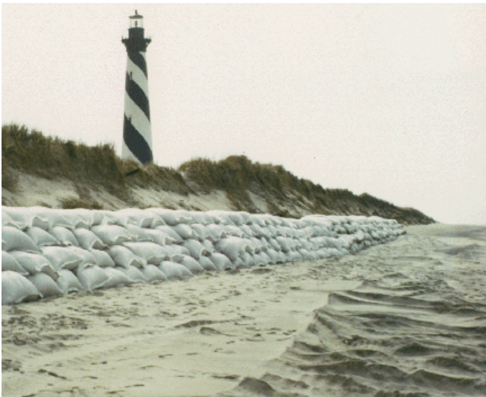
Figure 6. Photograph of the Cape Hatteras Lighthouse and the nearby beach. The sandbags are there to prevent further beach erosion. (Source: United States Geological Survey: pubs.usgs.gov/circ/c1075/images/lighthouse.gif )
