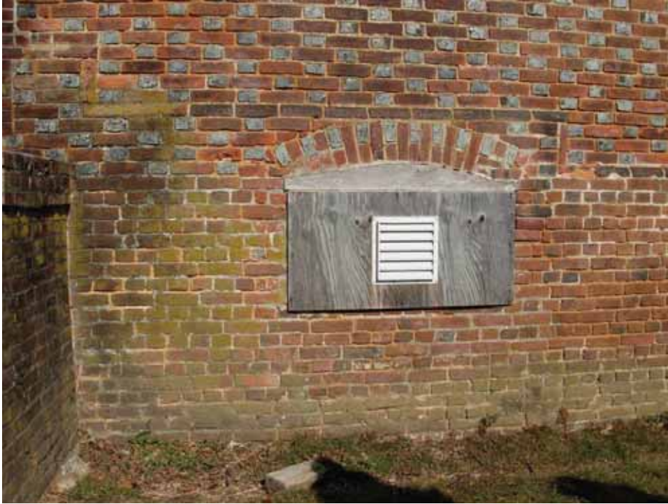
Figure 54. Photograph showing the water table and change in brick coursing on the east end of the south façade of the 1722 block of the Abel and Mary Nicholson house. (Source: A. Aiken; taken 2/23/2007.)
