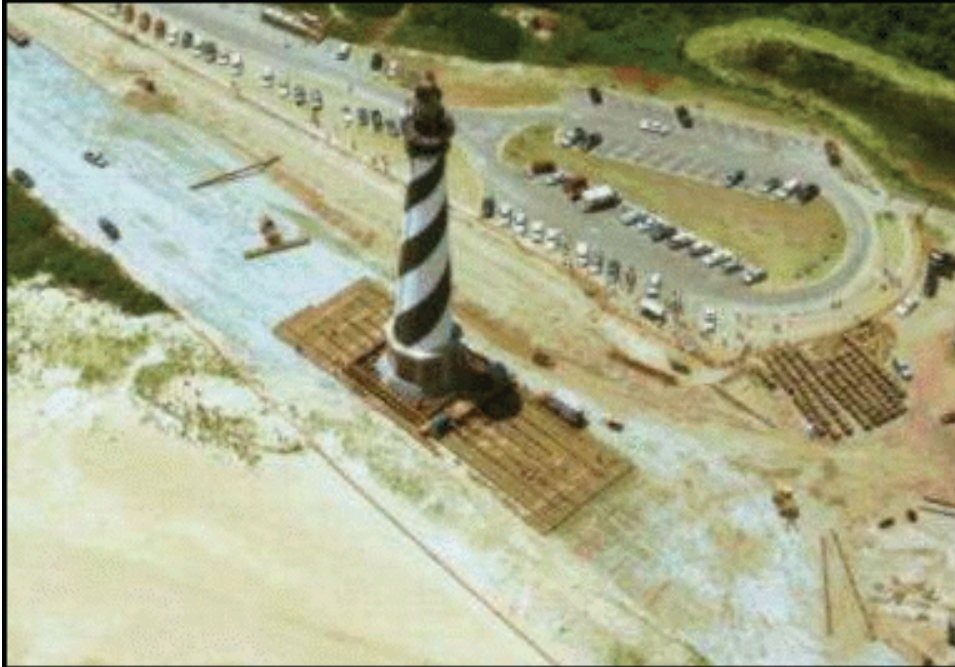
Figure 7. Photograph of the Cape Hatteras Lighthouse and the moving apparatus. (Source: National Park Service Photo: http://www.nps.gov/archive/caha/views.htm )
