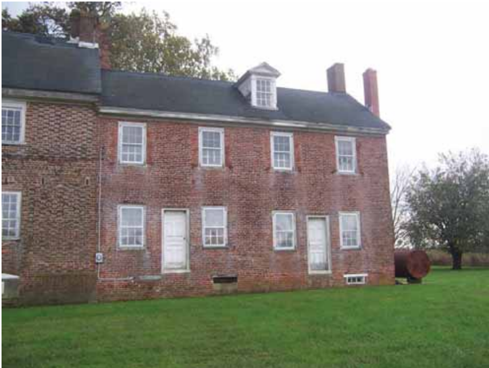
Figure 24. Photograph of the north façade of the 1859 addition block of the Abel and Mary Nicholson house. (Source: A. Aiken; taken 10/12/2006.)
