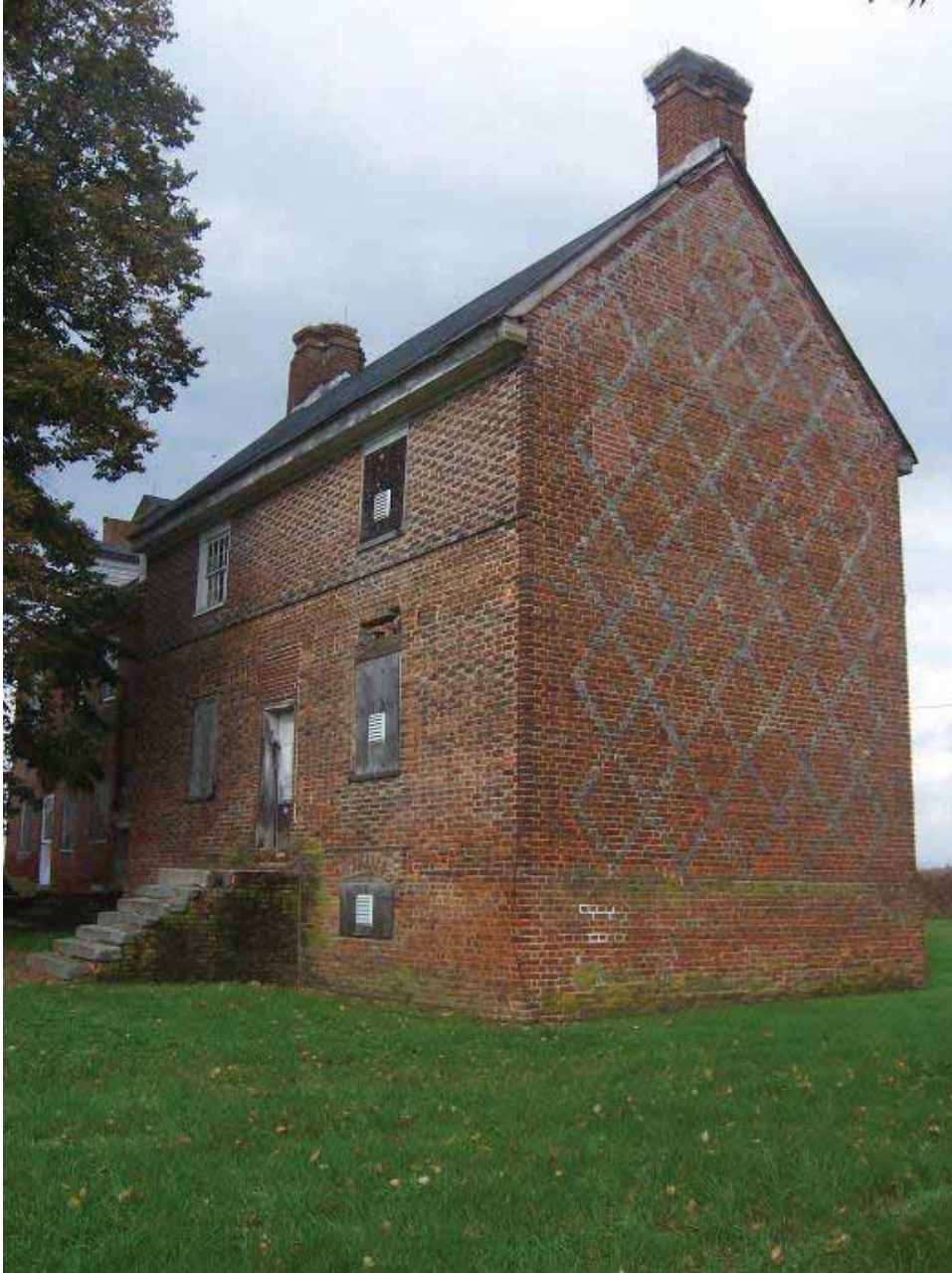
Figure 20. Photograph of the notable diapered-pattern brick end on the east façade of the Abel and Mary Nicholson house. (Source: A. Aiken; taken 10/12/2006.)
