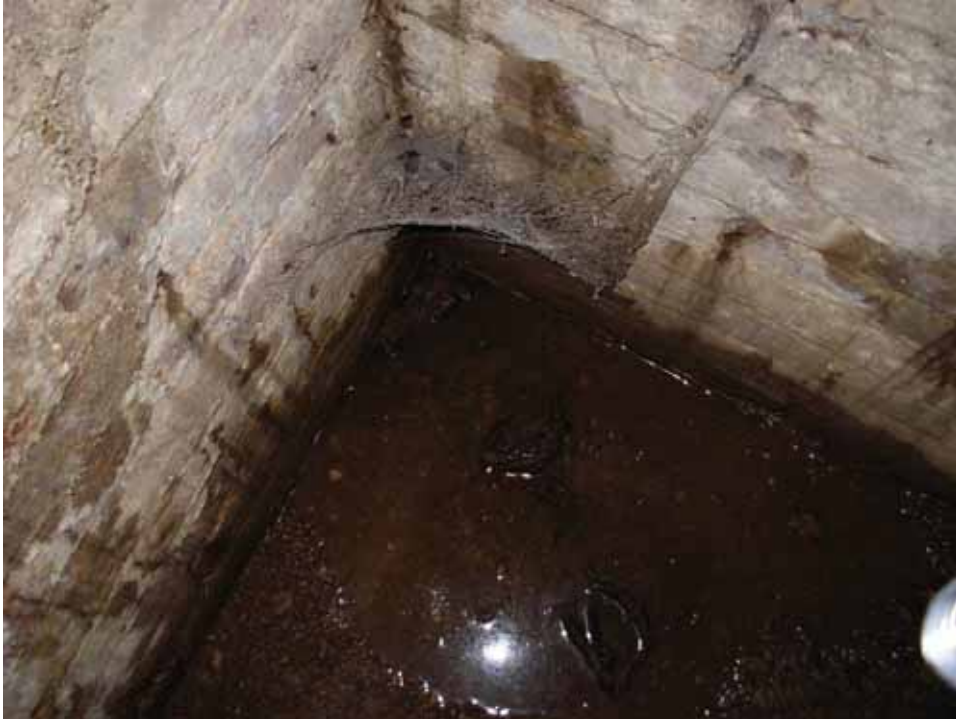
Figure 42. Photograph of the pool of water found at the southeast corner of the 1722 block east room of the Abel and Mary Nicholson house. (Source: A. Aiken; taken 2/23/2007.)
