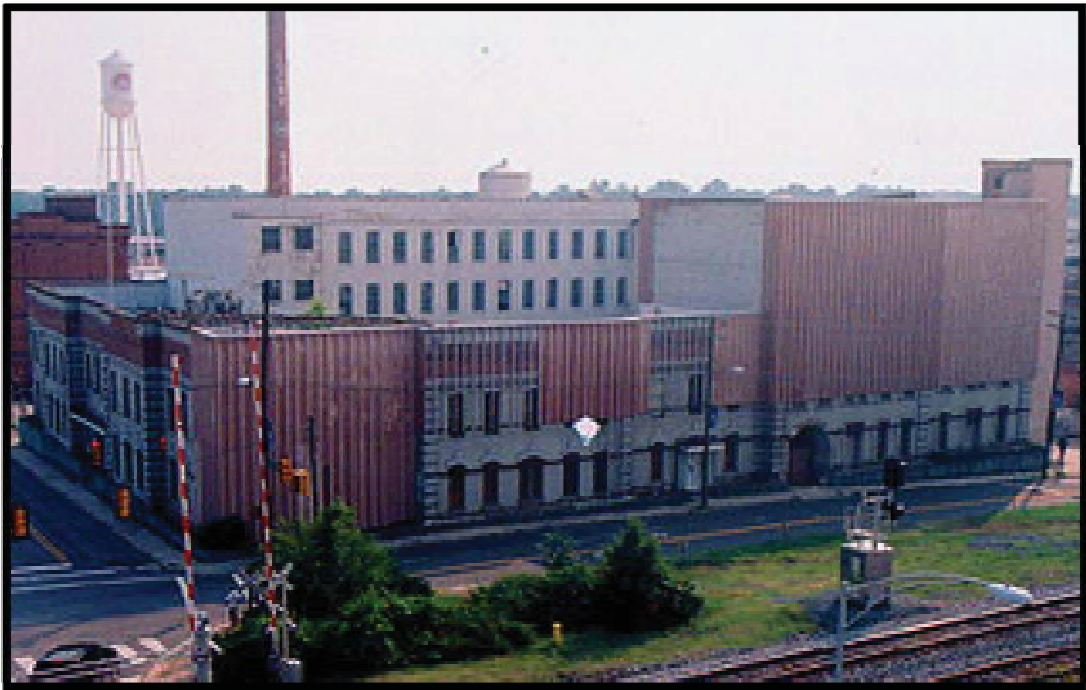
IMAGE 20: Blackwell Building façade removal (mid-2005)
