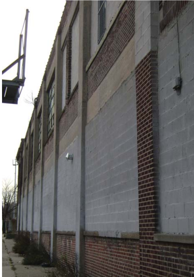
Figure 11a. View of Eastern facade, looking South
