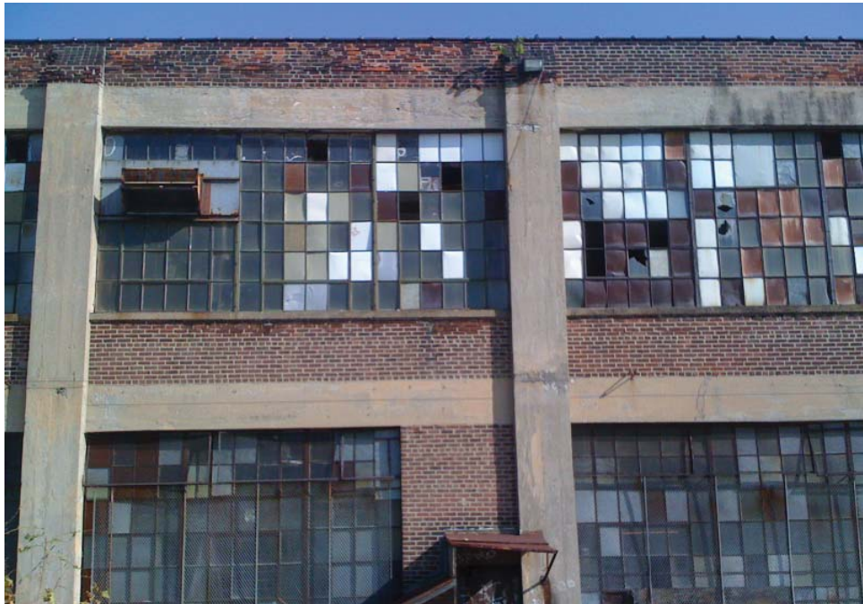
Figure 11b. View of Western facade, looking East
