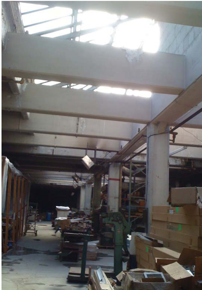
Figure 11c. Interior view of second floor
