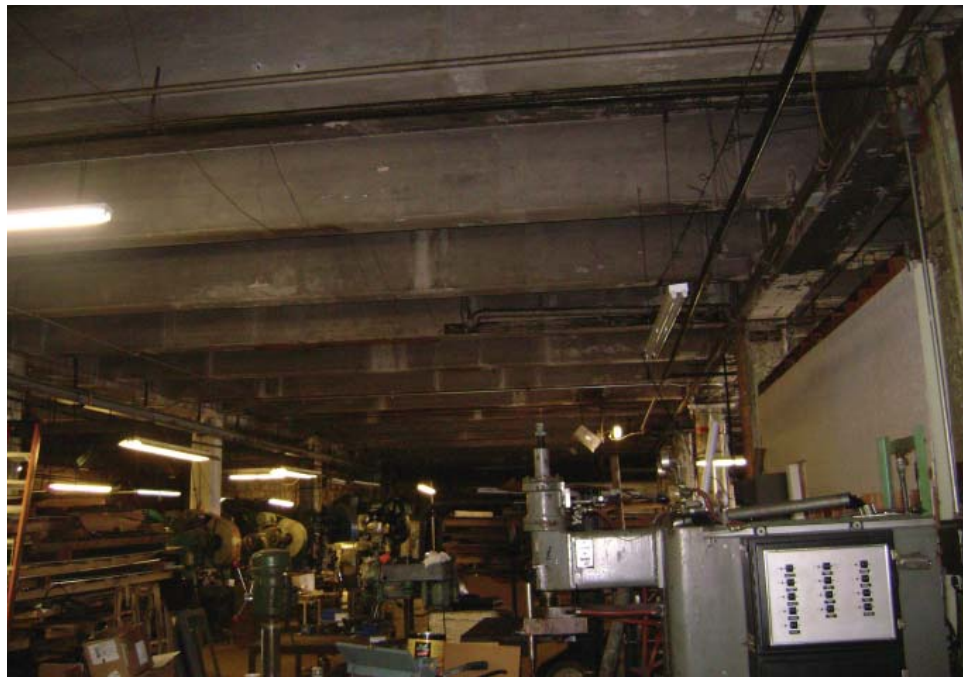
Figure 11d. Interior view of first floor
