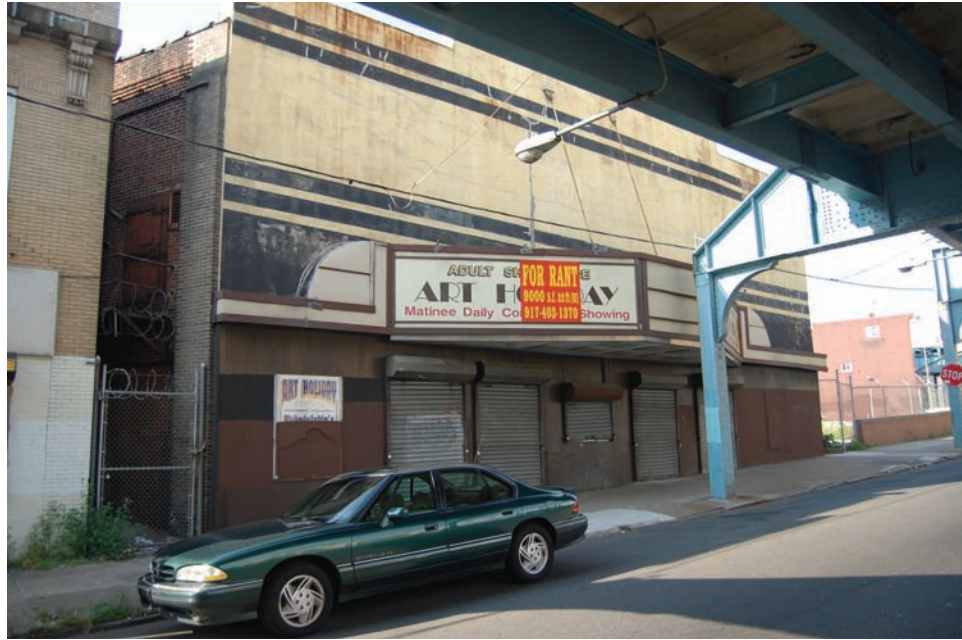
Figure 23. Holiday/Ace/Windsor Theatre William Harold Lee—Additions/Alterations (1938); Interior Redecorating (circa 1970) Source: Glazer, 54; PAB 4204-4212 Kensington Avenue, Philadelphia Photo by Author
