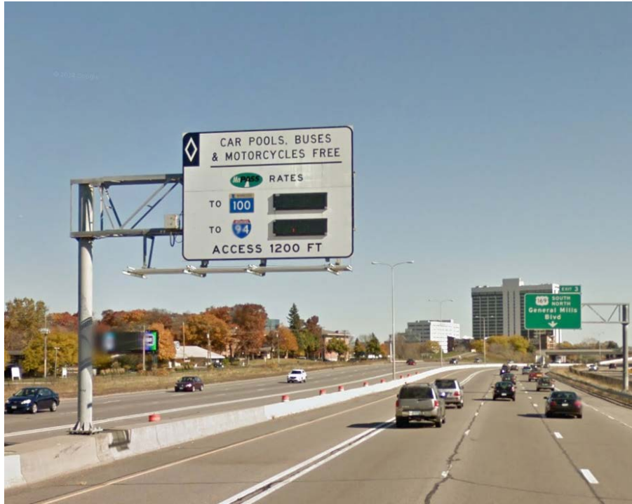
Figure 1-2 MnPASS price sign showing the two destination in I-394 EB
