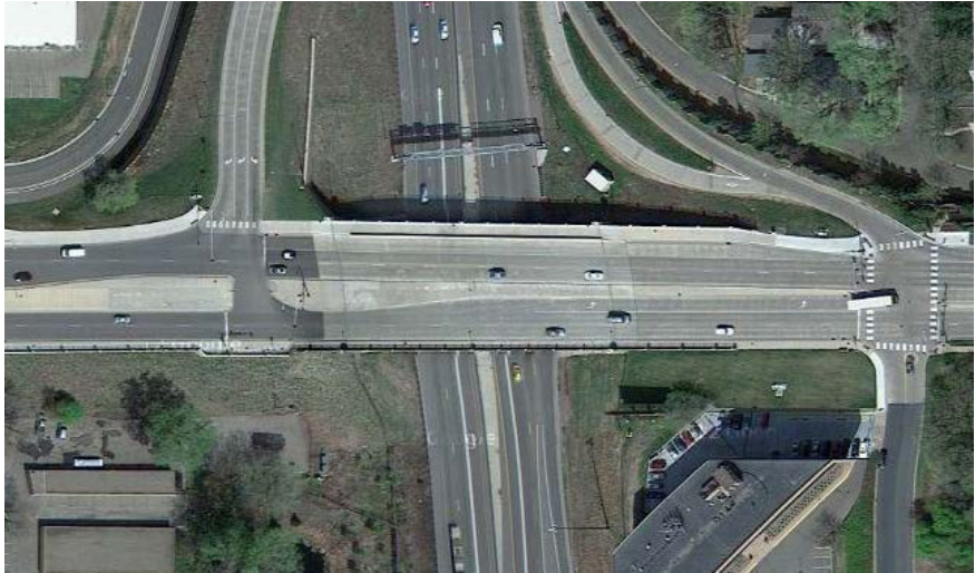
Figure 3-7 I-35W and 76th St Aerial Imagery (Google Maps)
