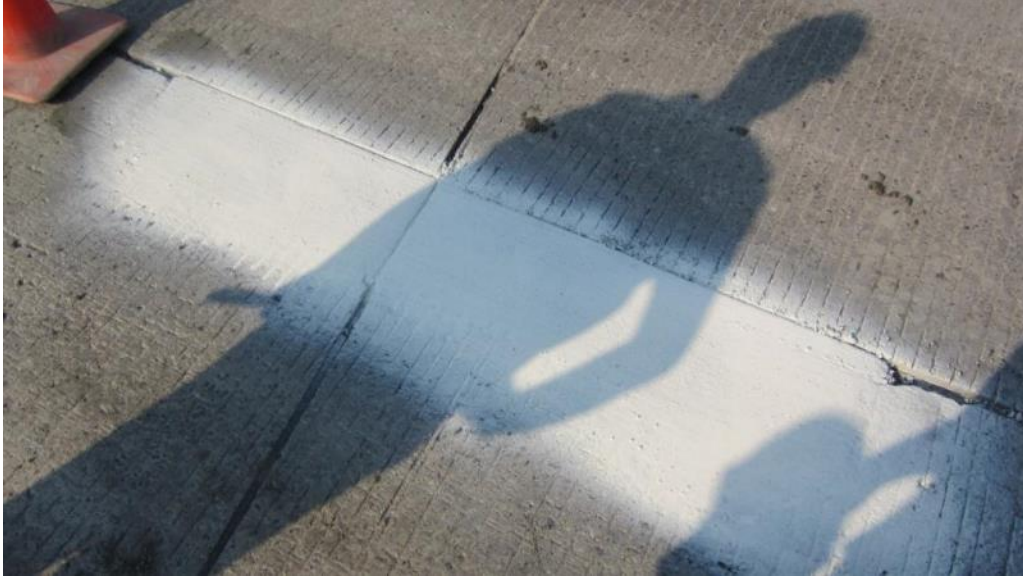
Figure 87: Finished patch with curing compound applied
