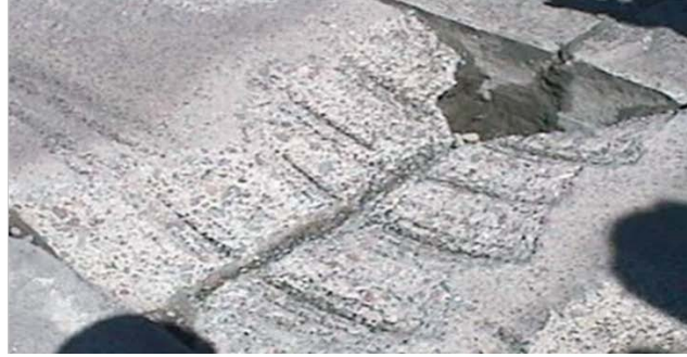
(b) Milled patch area
