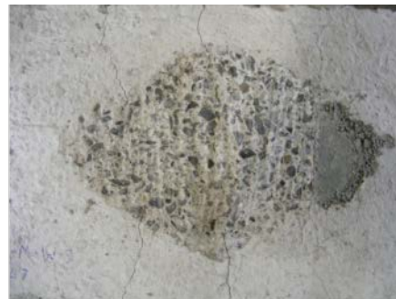
(b) Slab after testing
