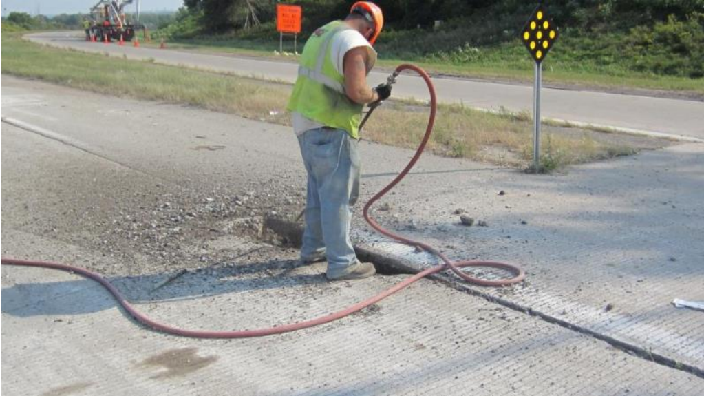
Figure 81: Air blasting the hole to remove excess loose material
