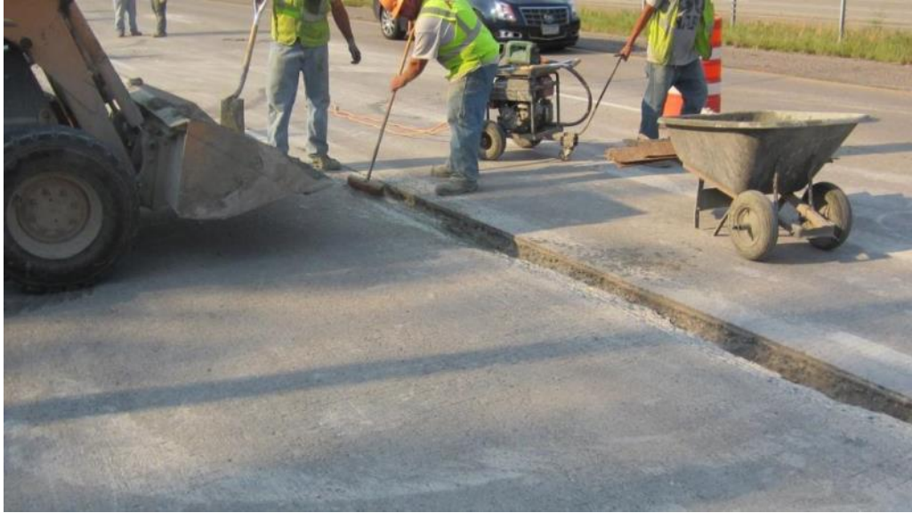
Figure 85: Applying the concrete slurry that provides adhesion for the patch material
