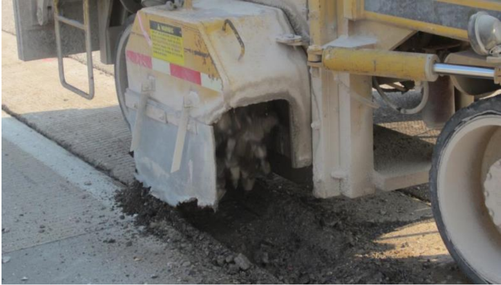
Figure 79: Milling machine grinding a spalled section of concrete
