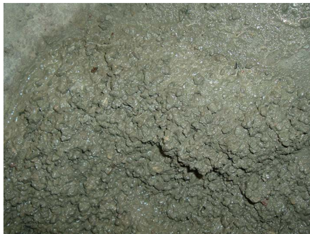
Figure 3-2 Fresh 3U18 patching material before placement
