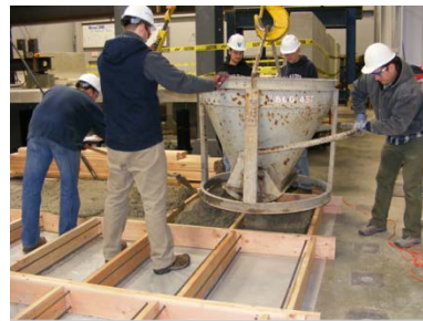
(a) Concrete placement
