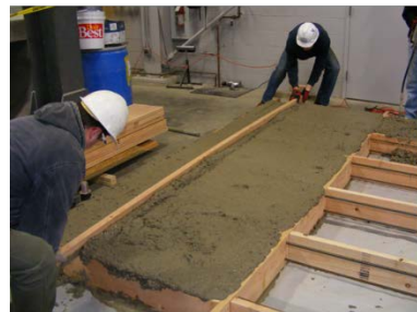
(c) Concrete screeding
