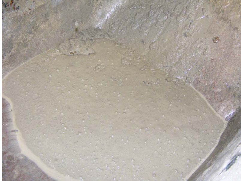
Figure 3-3 Fresh Futura-45 patching material before placement
