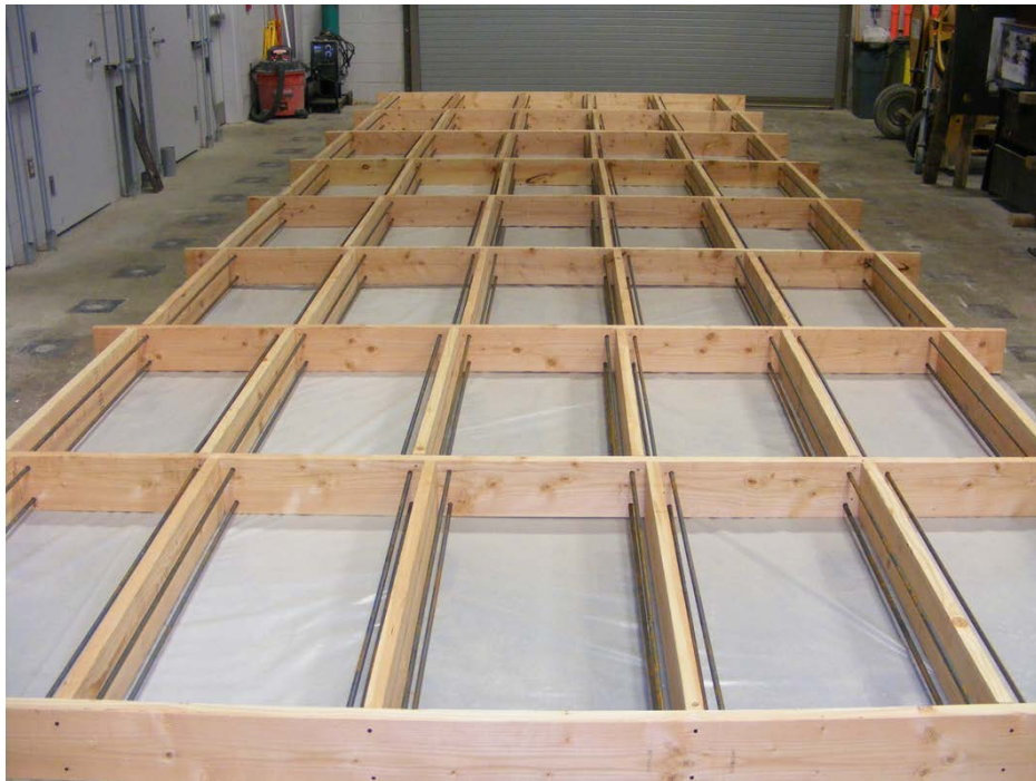
Figure 3-13 Formwork for slab bending specimens
