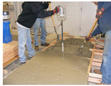
(b) Concrete vibration
