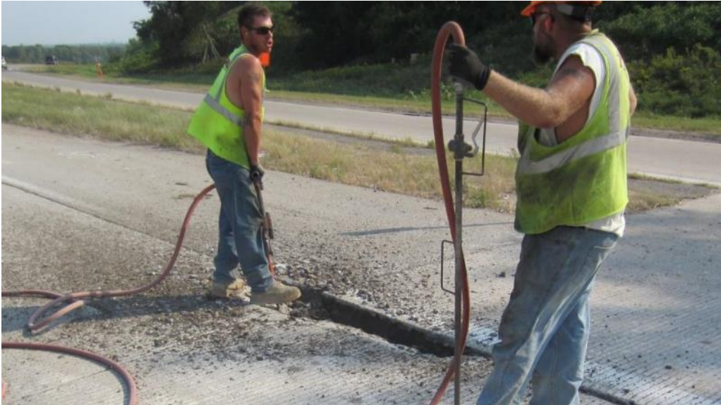
Figure 80: Chipping the edges to meet MnDOT specifications
