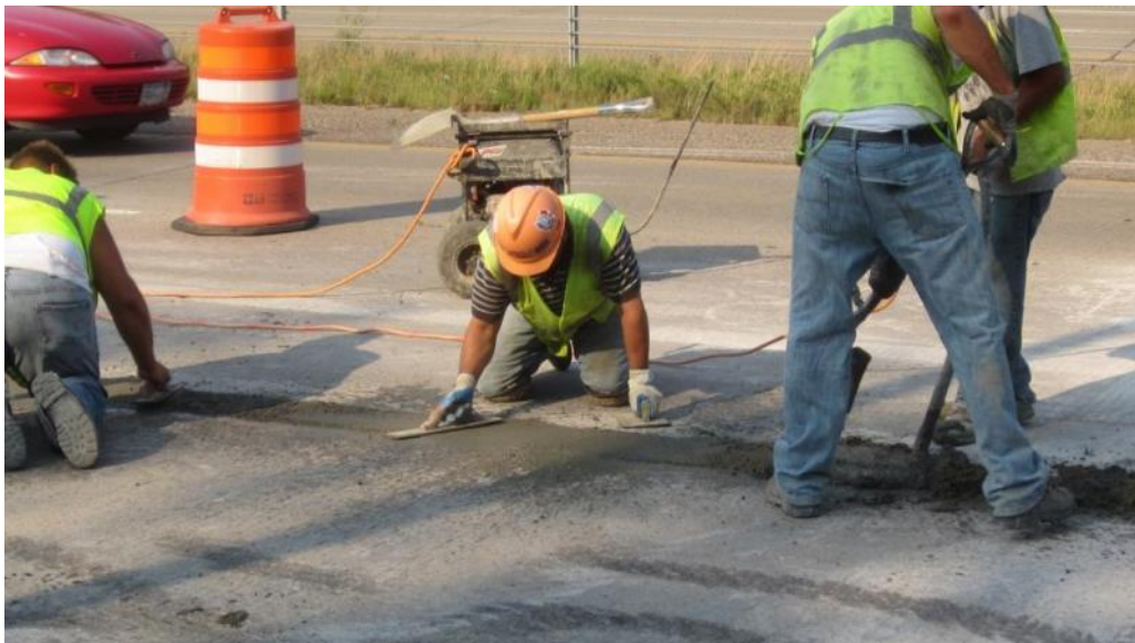
Figure 86: Placement, consolidation and finishing
