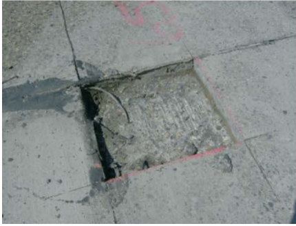
(a) Saw cut and chipped patch area
