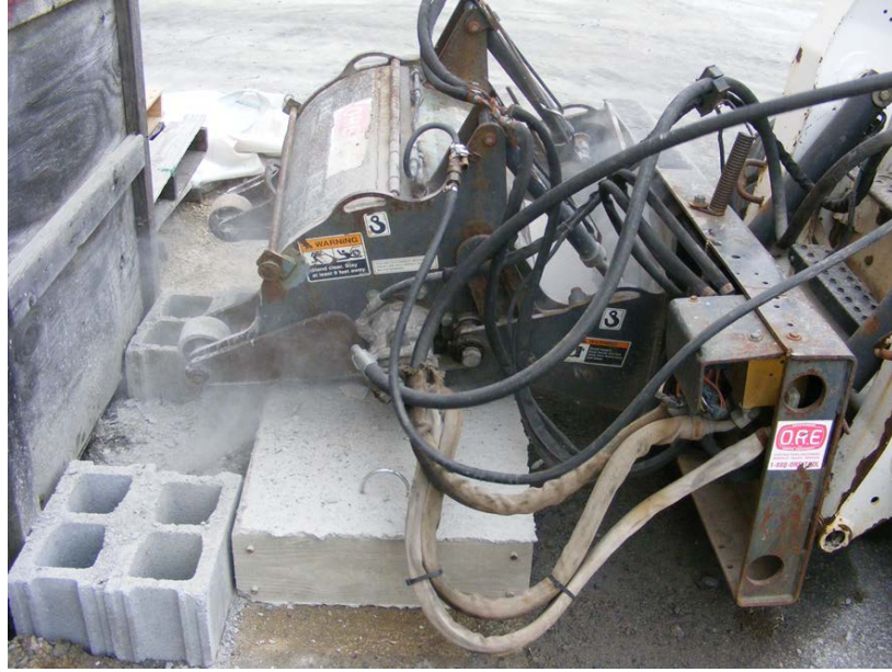
Figure 3-16 Slab being milled
