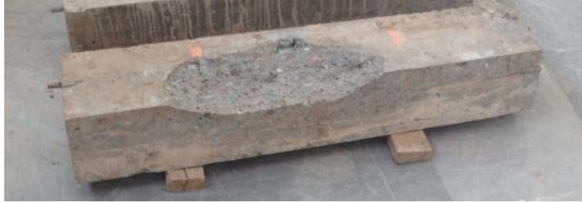
Figure 19: Slab after being cut longitudinally to expose the patch material edge.
