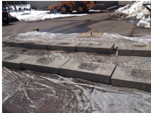
Figure 18: Test slabs containing partial-depth simulated repair areas.
