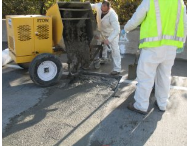
Figure 1-1 Futura-45 bag mix being placed in the field ( http://www.wrmeadows.com/futura-45-horizontal-repair-mortar/ )
