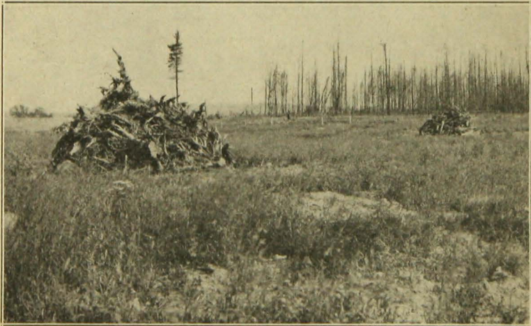
Fig. 7. After Stumping and Before Plowing
