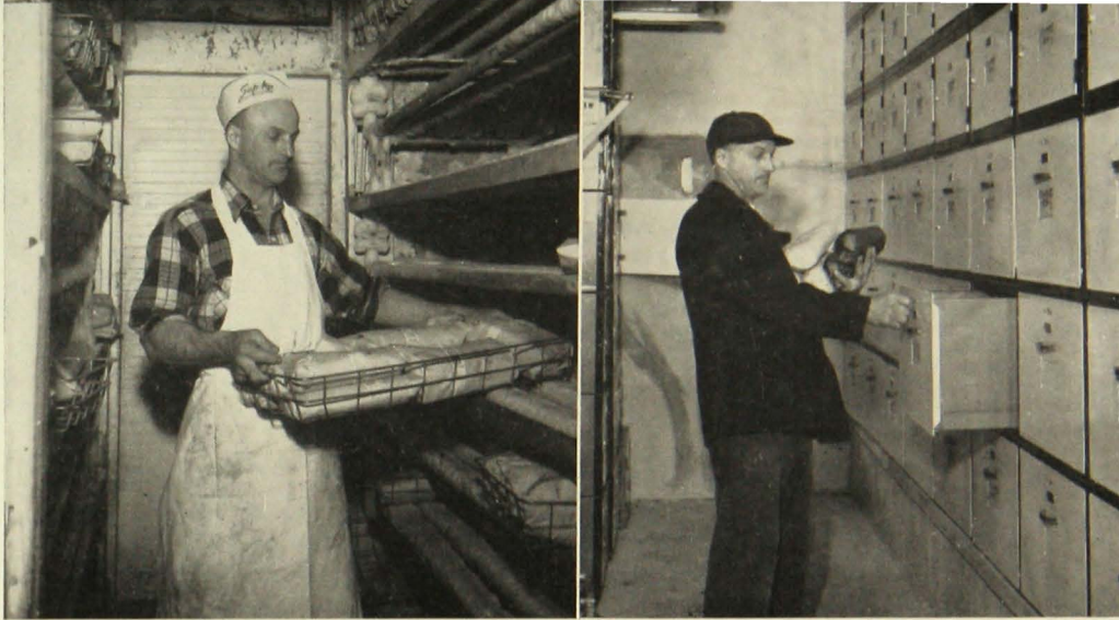
Fig. 6. Packages of food are frozen quickly in a freezer room (left) and stored until needed in the drawer- (right) or door-type lockers.
