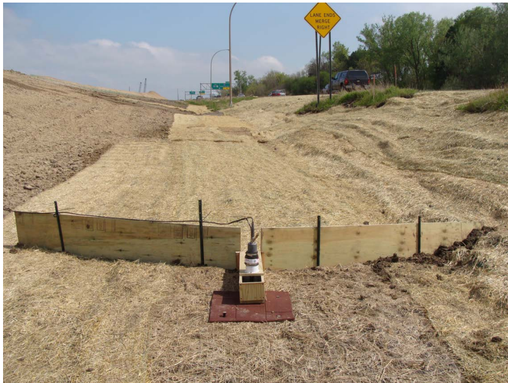
Figure 5.5. Turbidity box with wing walls monitoring ditch
