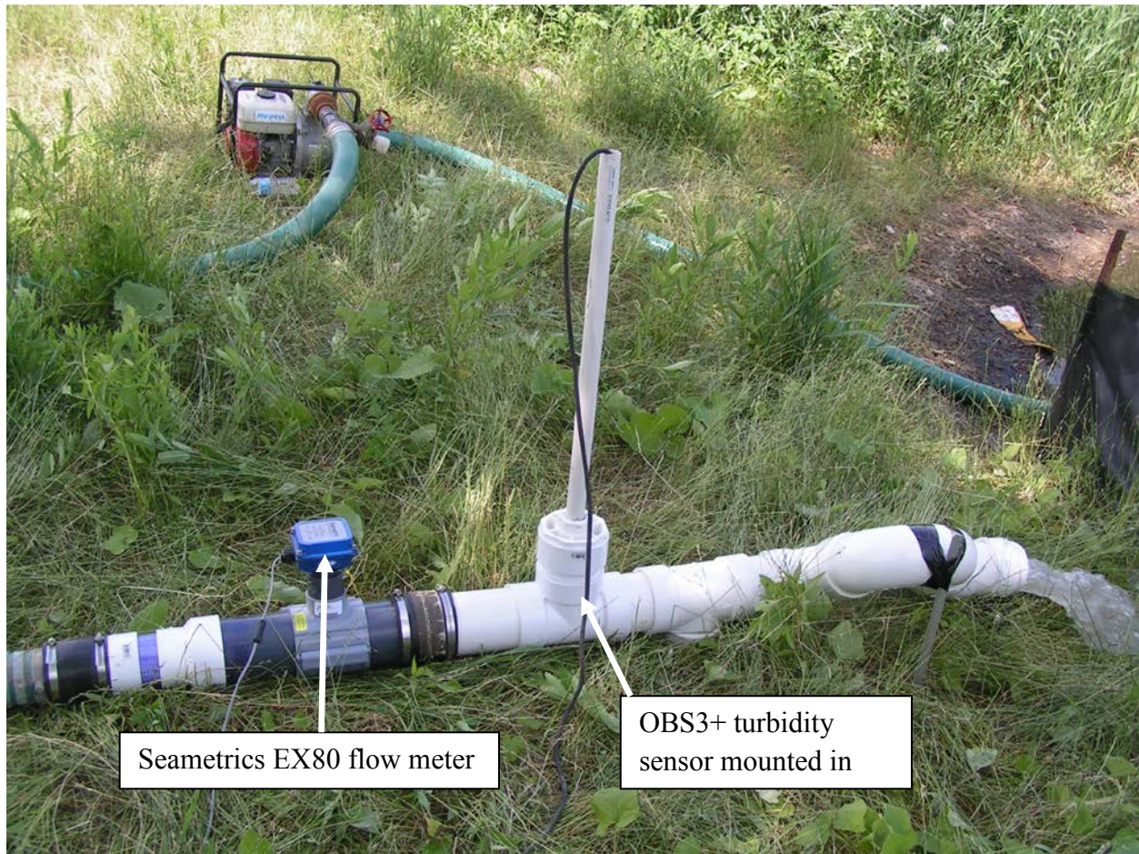
Figure 5.13. Portable de-watering monitoring system
