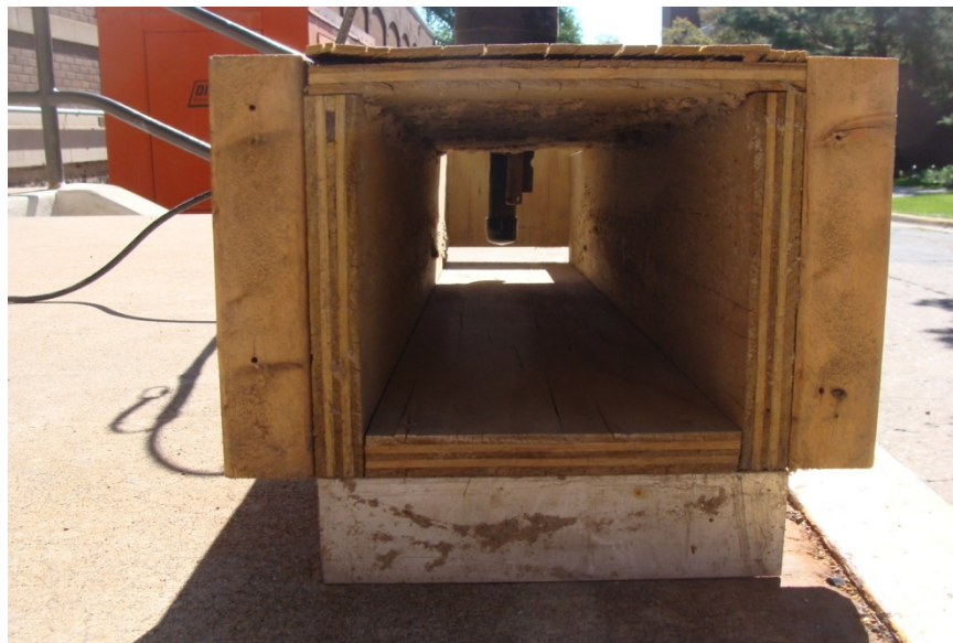
Figure 5.2. Upstream end with 1 1/2 inch angle iron attached to prevent water undercutting beneath the box.
