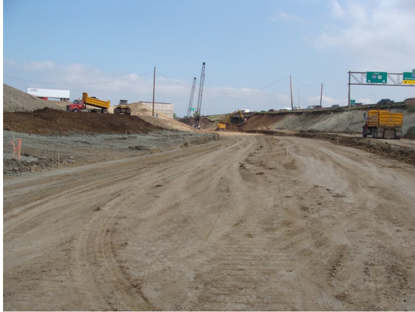
Figure 5.24. Construction site at Snelling/694
