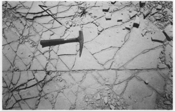
FIGURE 9. Waterville Quarry floor with apparent offset of N5E-trending joints against N45W systematic joints.
