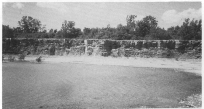
FIGURE 6. North wall of Waterville Quarry showing first-formed N45-50W systematic joints.
