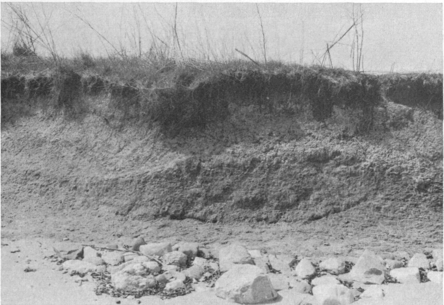
FIGURE 13. Talus washed from base of bank by waves. April 8, 1949.
