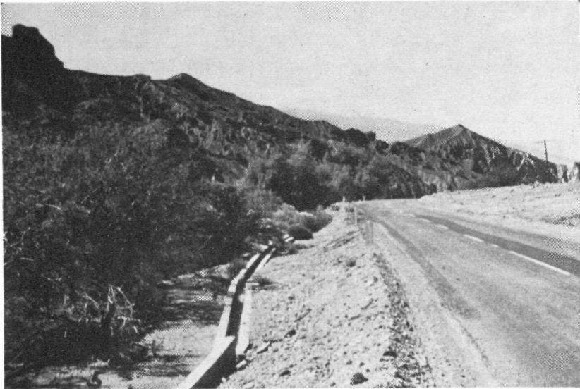
FIGURE 5. Furnace Creek Wash. From Travertine Stream and Pond, the water flows in a cement trough, as pictured, into the Furnace Creek Ranch area. The trough runs parallel to Rt. 190.
